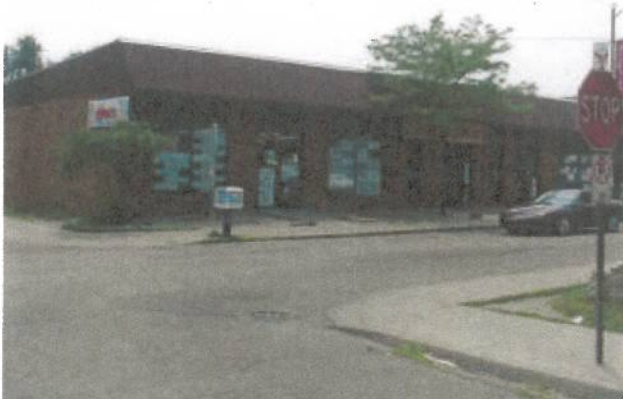
Example of 'marginal' building in the neighborhood.
