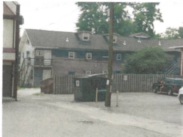
Example of 'maintenance deprived' building in the neighborhood.
