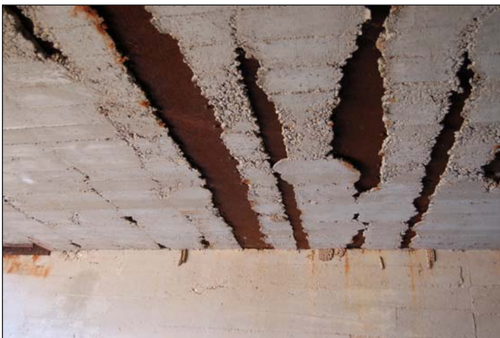
Bottom of Deck
