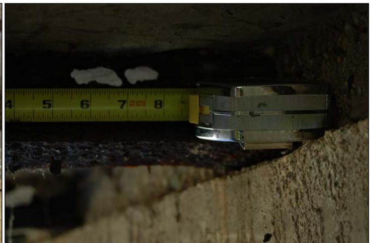
Beam # 4 from North
