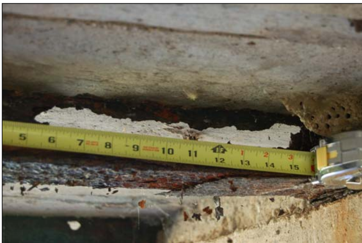
Beam # 3 from North
