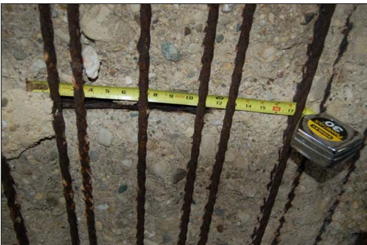
Bottom of Deck
