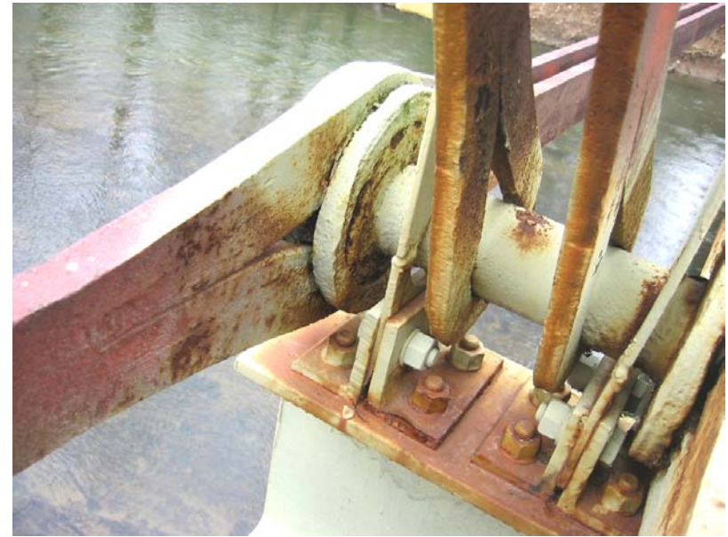
130 Panel point L8 south - thin hanger section
