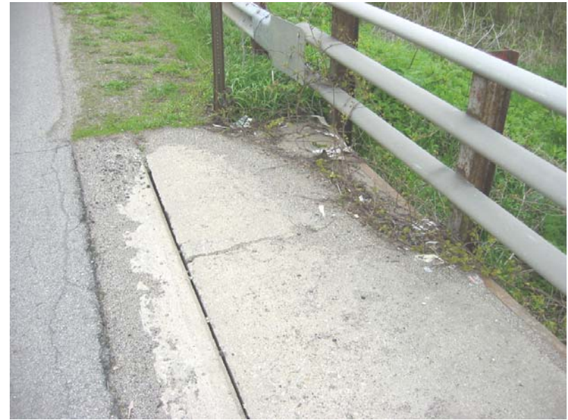
125 Widened deck cracked at northeast corner
