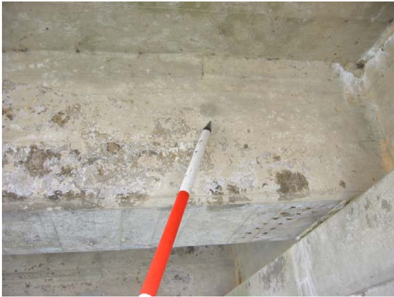
121 Typical horizontal cracks in beams
