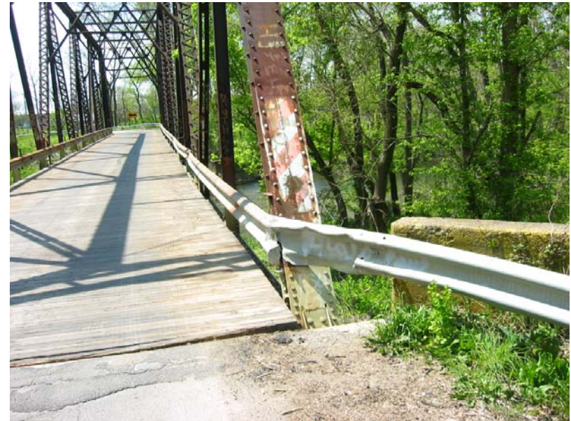
161 Rail damage at the northeast corner
