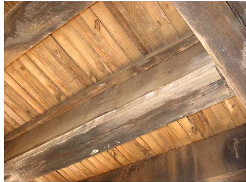
226 Beam split at top and bottom in main span
