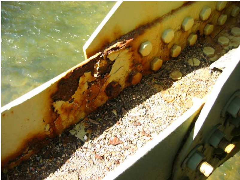
161 Rust-through at one leg at L6
