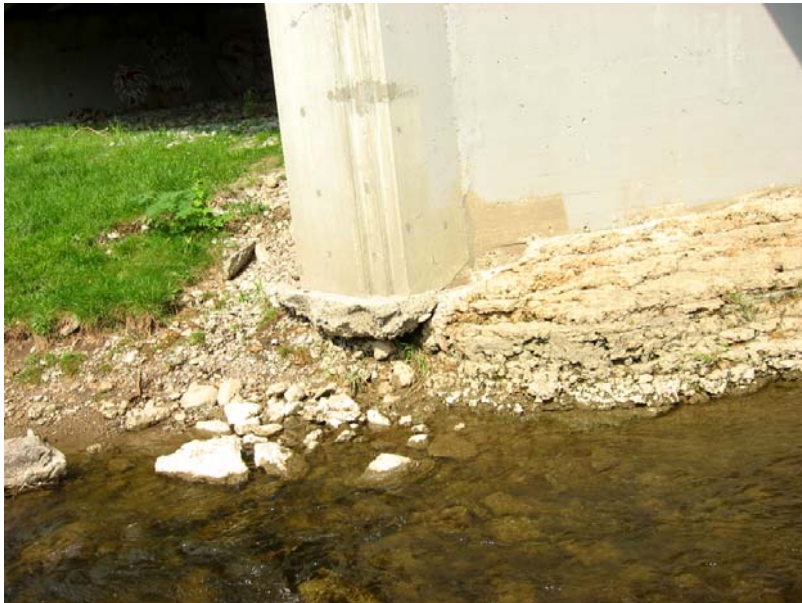
506 Base undercut at the ends of the piers
