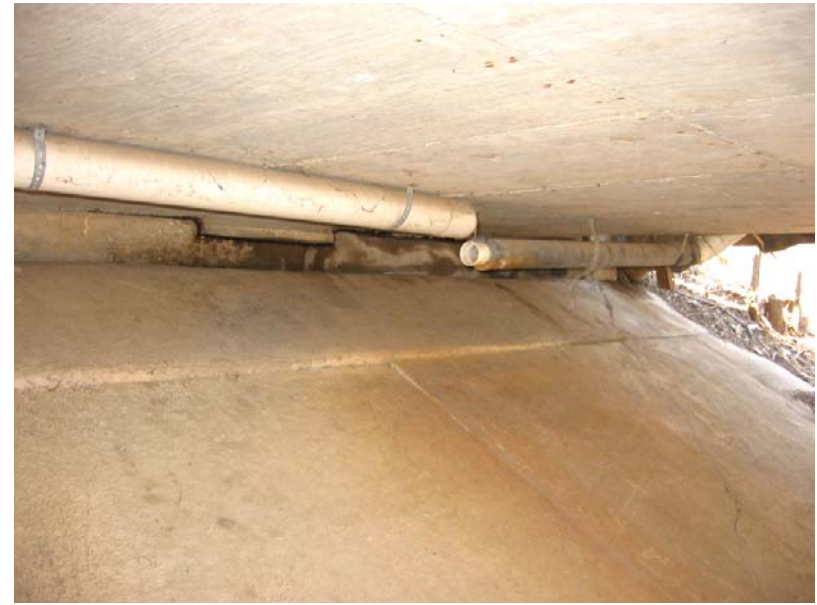
268 Pipe broken at the west end bent
