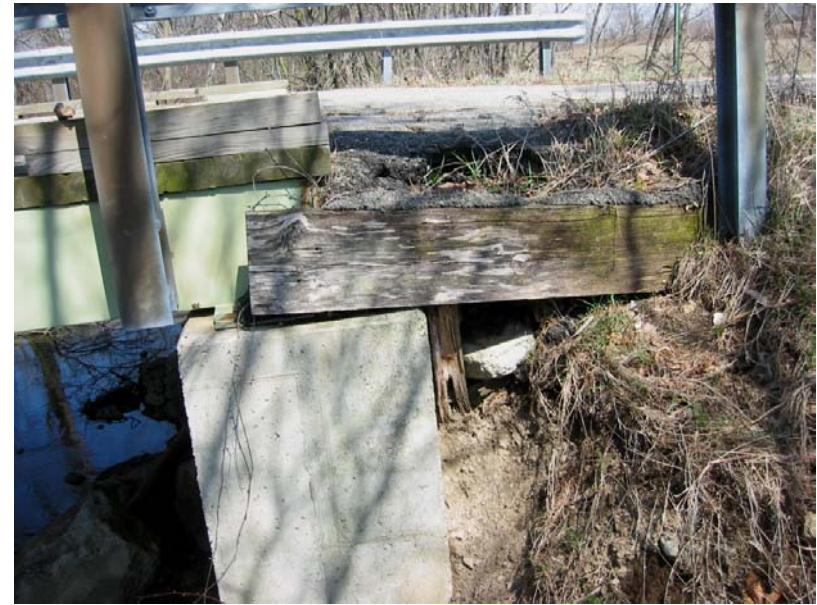
042 Typical erosion at corners
