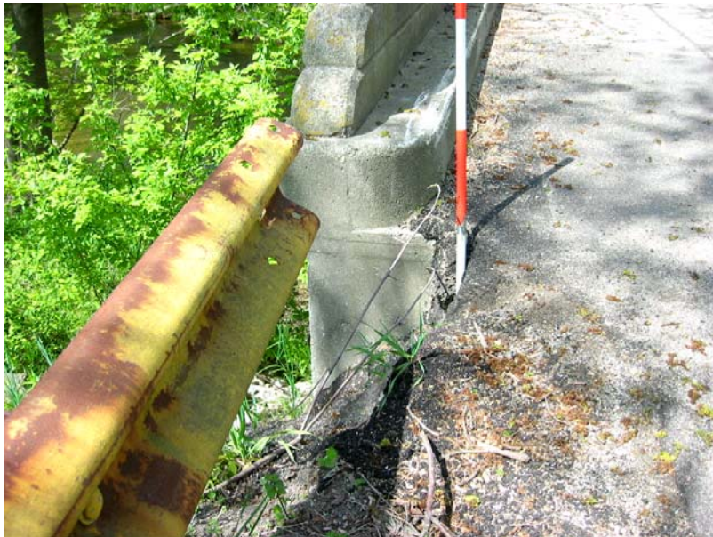
092 Eroded southeast shoulder
