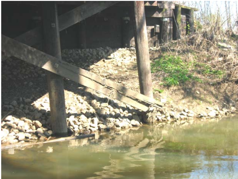
063 Split timber brace at the north interior bent
