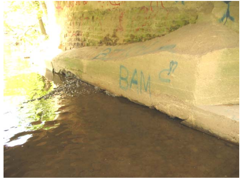
092 West abutment deteriorated at the waterline
