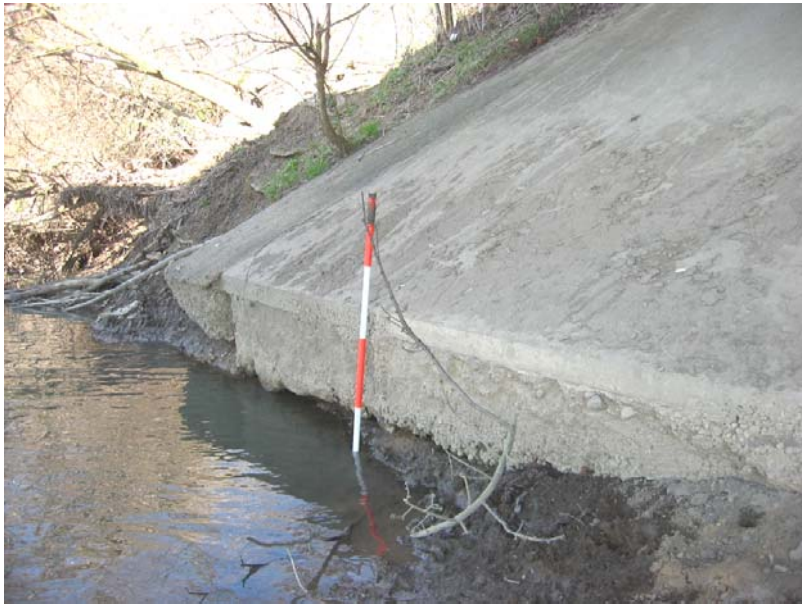
141 Erosion at the toe of the north slopedewall
