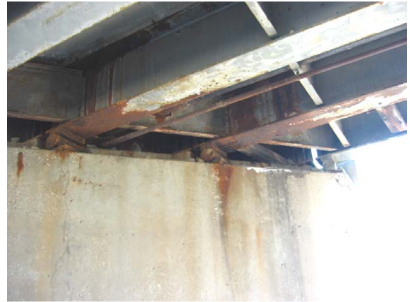
513 Rust and delamination in beams at the west pier
