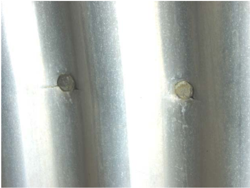
058 Tears around bolt heads
