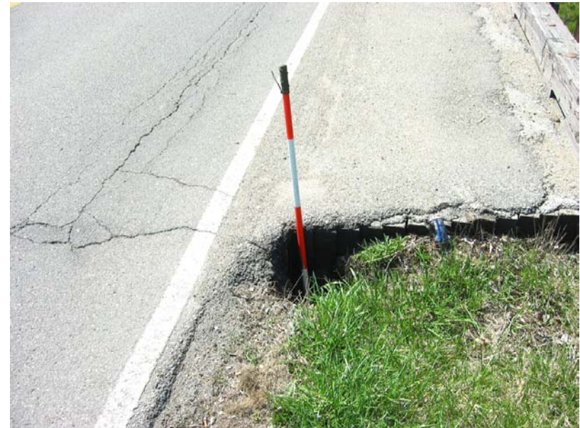
047 Apparent fill loss - hole at the northeast corner
