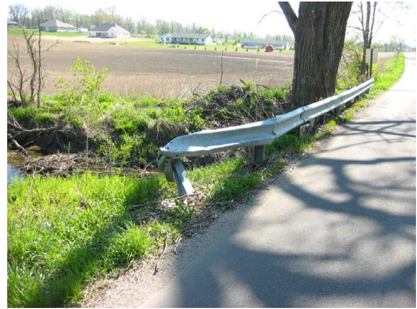
158 Damage to west end of guardrail
