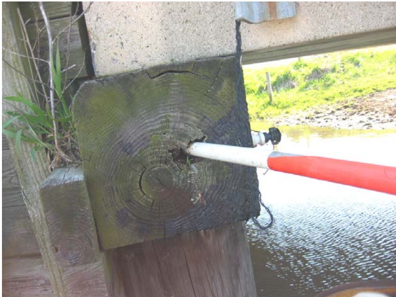
015 Rot in the north end bent cap at the west end
