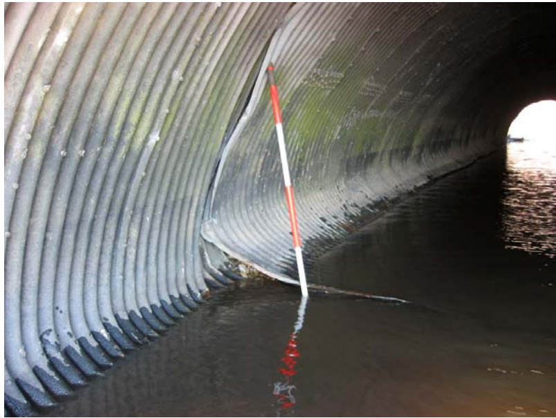
207 Open joints at arch plates
