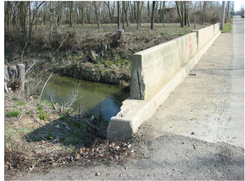
502 Bridge rail broken at the northeast corner (very little re-steel)
