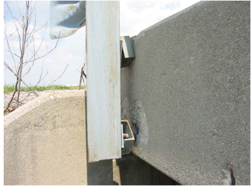
003 Northwest rail post connection damaged
