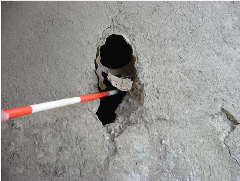
001 Failed pipe and void at the north sloped wall
