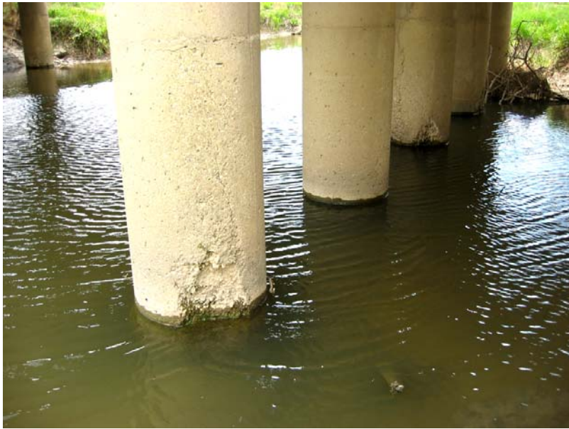
100 Spalled pile encasements
