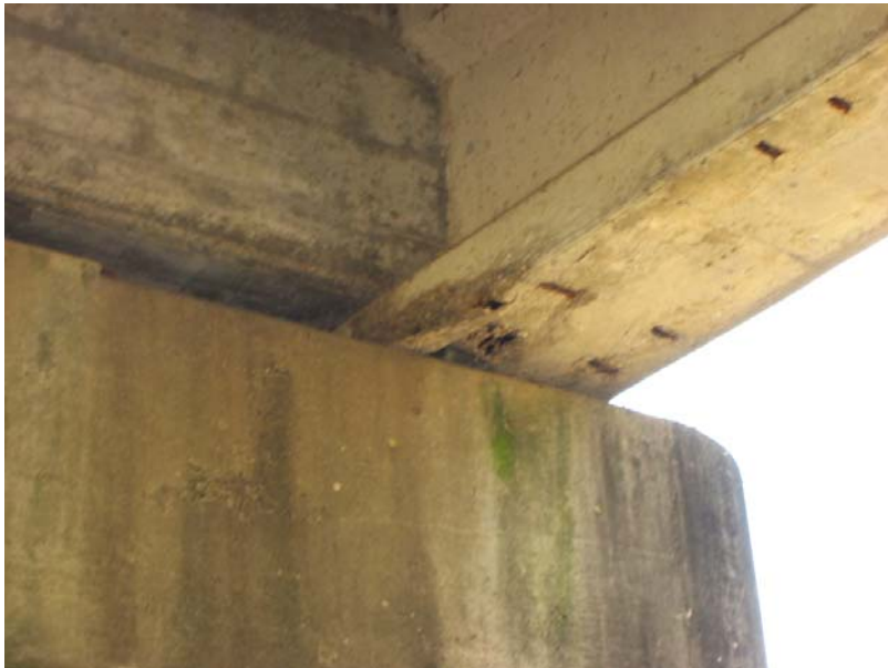
020 Bottom flange of beam spalled - exposed strands
