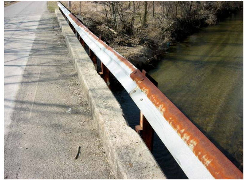
198 Damaged rail and connections
