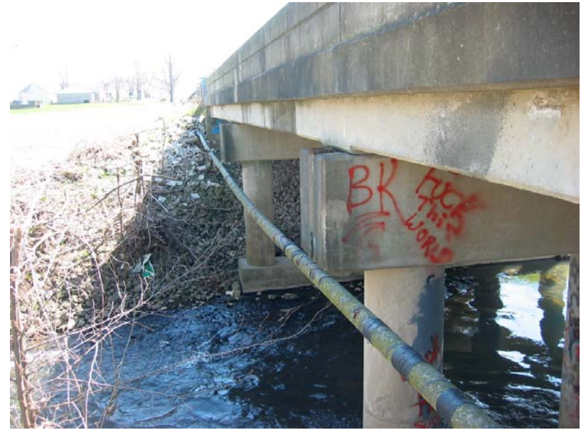
209 Gas main hanging - hangers are broken
