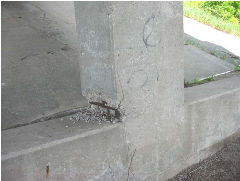
520 Damaged column in the north interior bent
