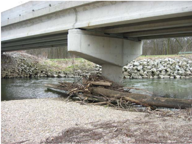
131 Debris buildup at south pier
