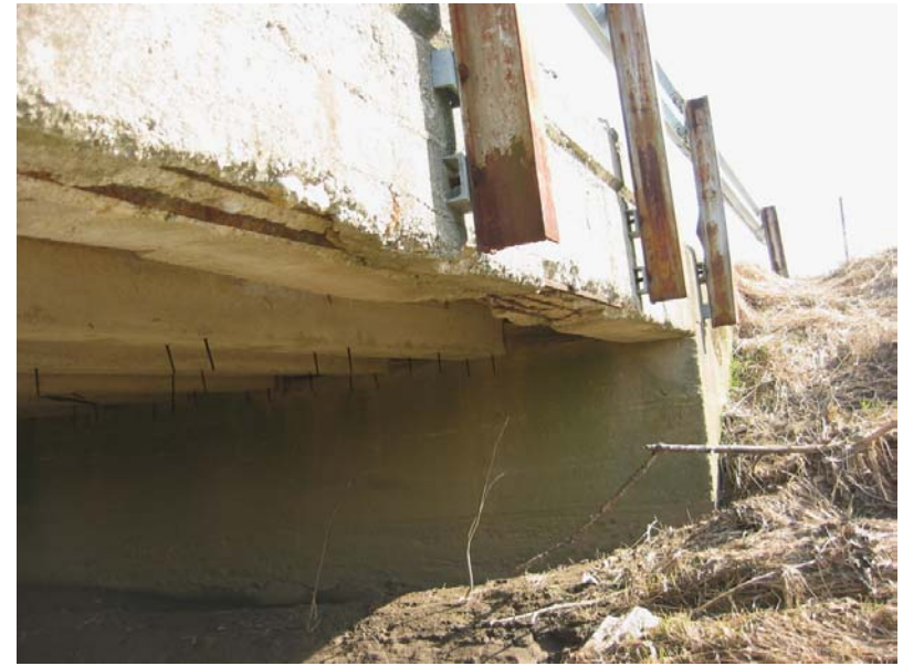
035 Spalled outside beam
