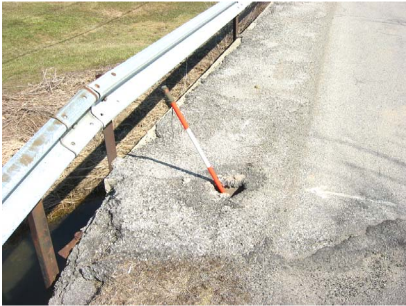
191 Hole in pavement at northwest
