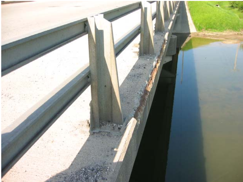
193 Spalls along the north coping
