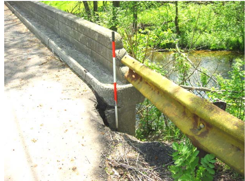
092 Eroded southwest shoulder
