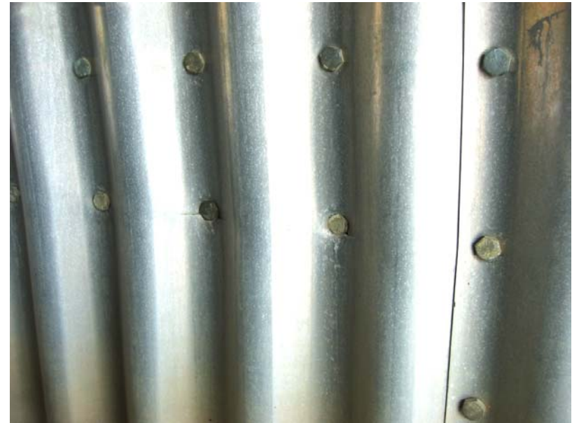
058 Tear in plate at bolt head
