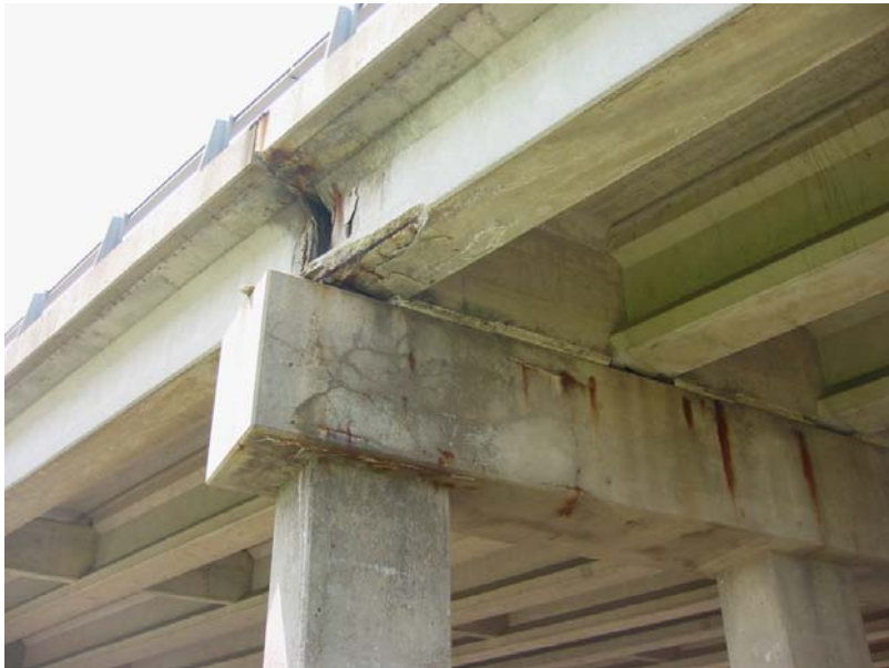
520 Beam damage at the east end of the north interior bent
