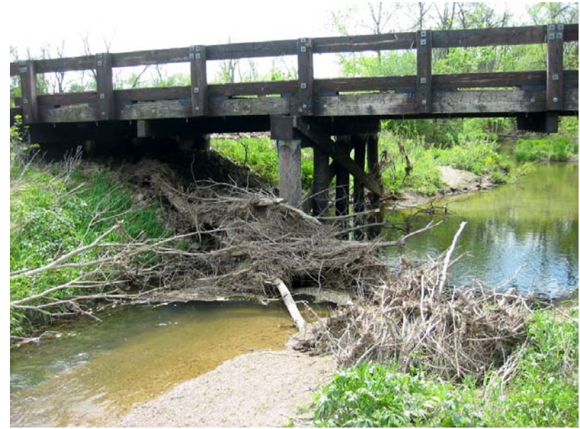
097 Debris at the south interior bent
