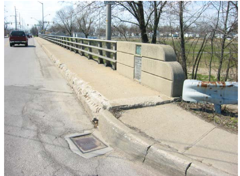
513 Settled sidewalk, deteriorated curb
