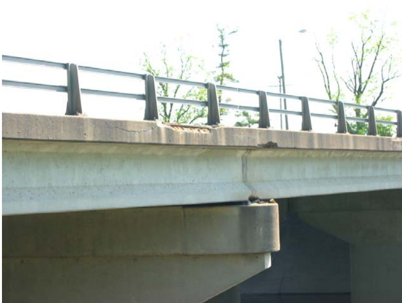
193 Damage to the south coping and typical spalled grout at beam ends
