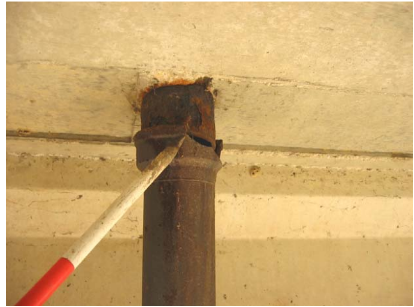
123 Northeast pipe extension broken
