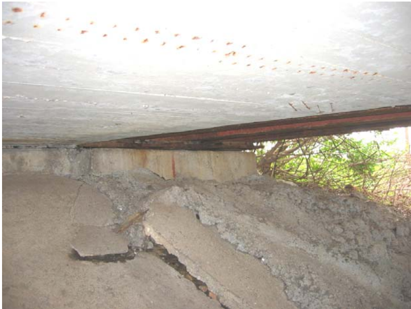
125 Southwest substructure settled and slopewall damaged at southwest corner
