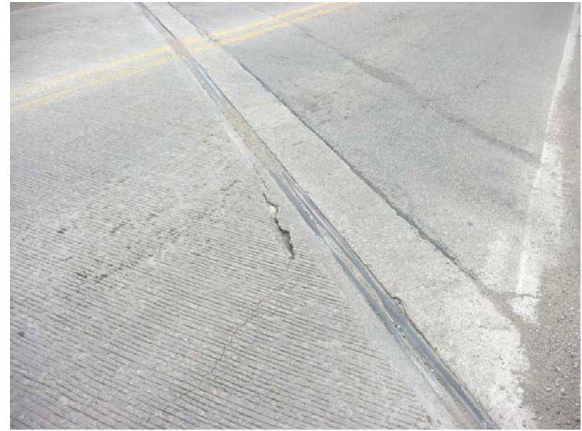
143 West end of deck cracked and damaged
