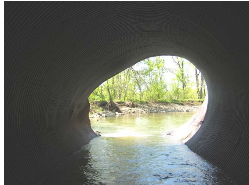
016 East pipe outlet distorted
