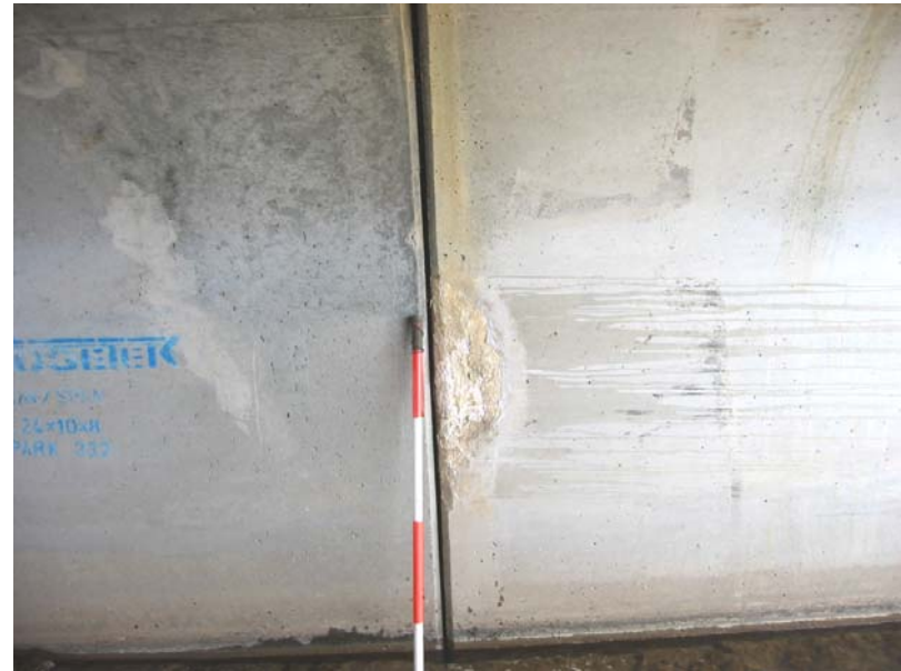
070 Deteriorated patch in arch below
