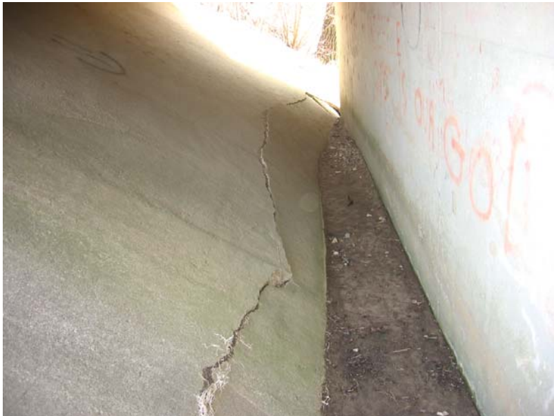
120 North slopewall broken and settled.
