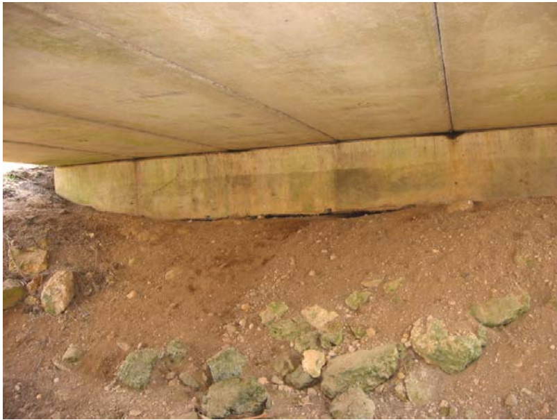
165 Burrows and undermining at the south endbent
