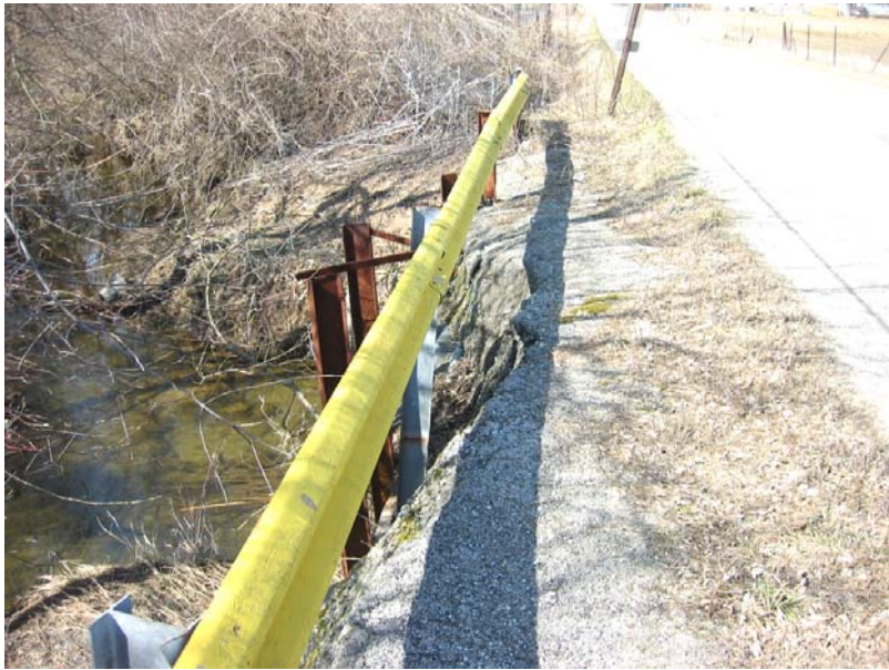
194 West shoulder eroded
