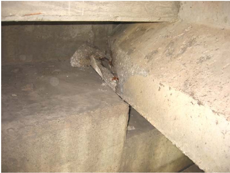
193 Typical damage at the beam ends at the endbents
