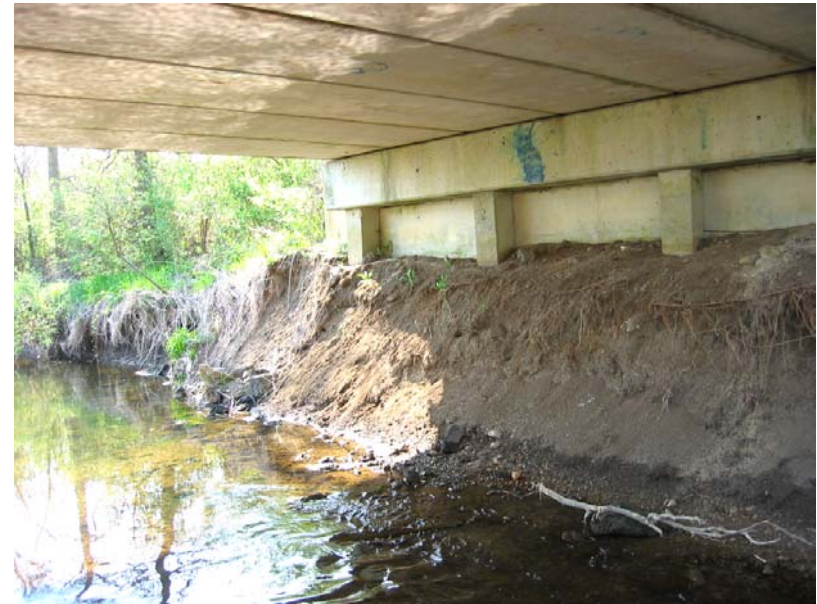
109 Erosion at the south bank
