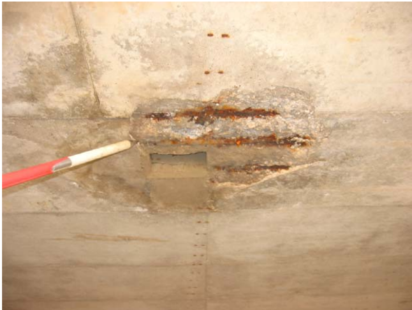
268 Spalls around drain outlets
