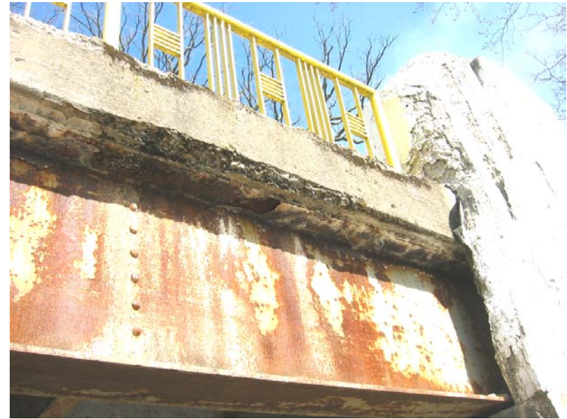
107 Rust and section loss in top of west beam
