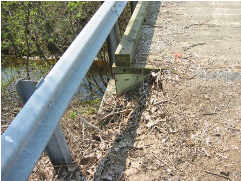
017 Erosion at the southeast corner
