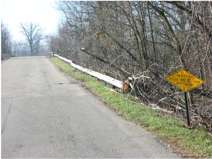
084 Damage at the northwest approach rail
