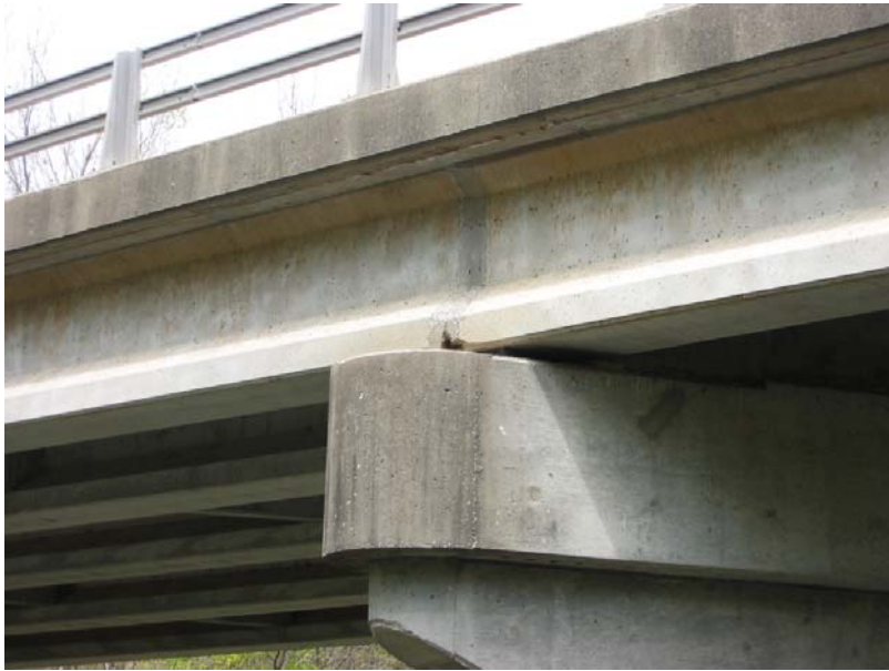
148 Deteriorated grout at beam ends over piers
