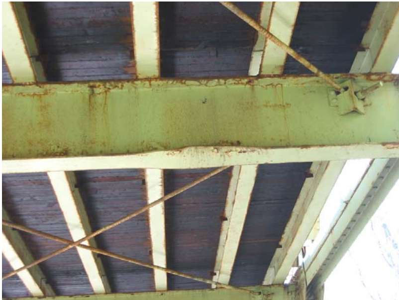
161 Floor beam 7 with damaged flange
