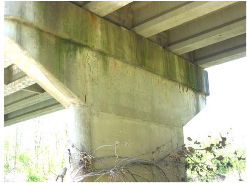
021 Spalling in piers
