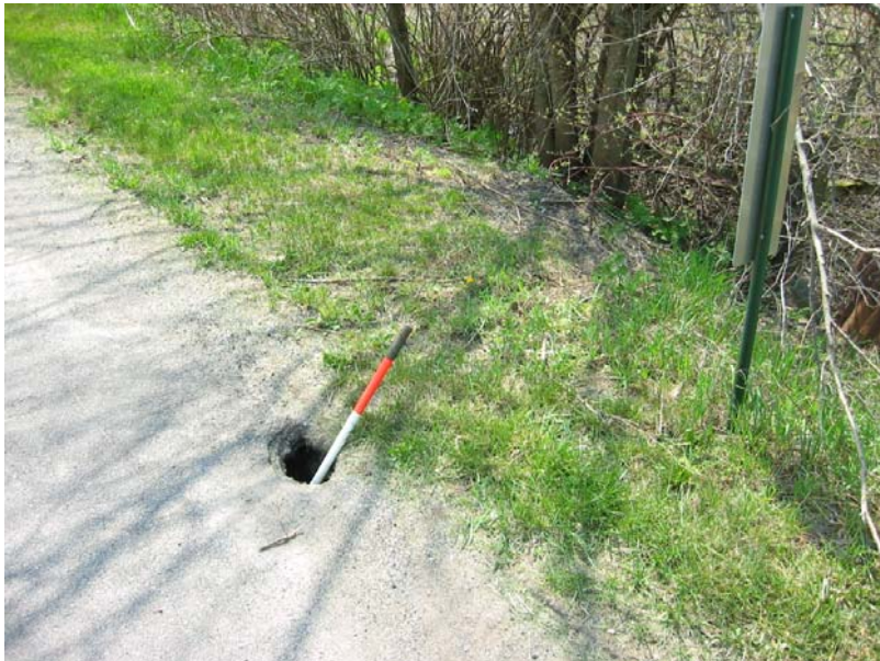
165 Hole in the south approach pavement
