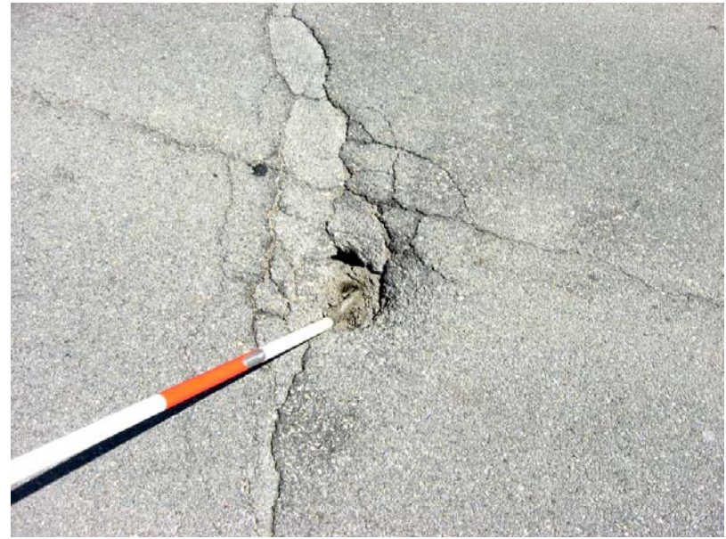
069 Apparent fill loss - hole in pavement at south end
