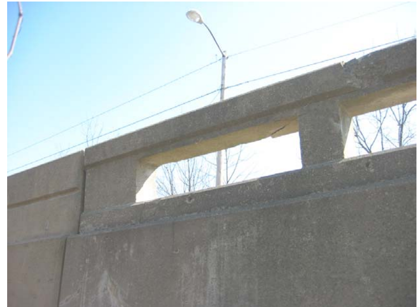
141 Northwest rail damaged - picture from outside
