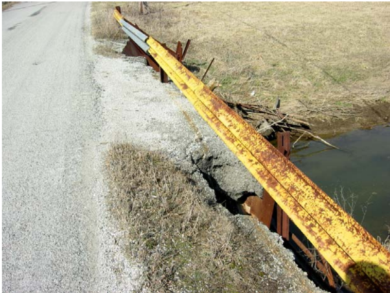
196 East side fill failure
