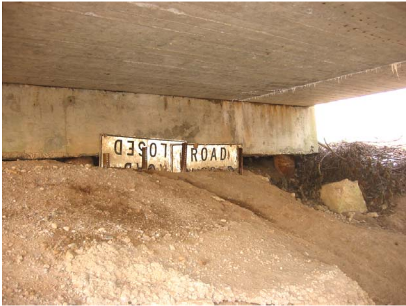
118 West end bent cap undermined - north end
