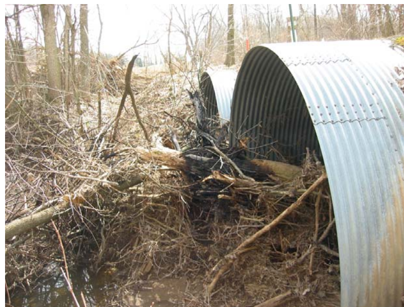
040 Heavy debris at inlet
