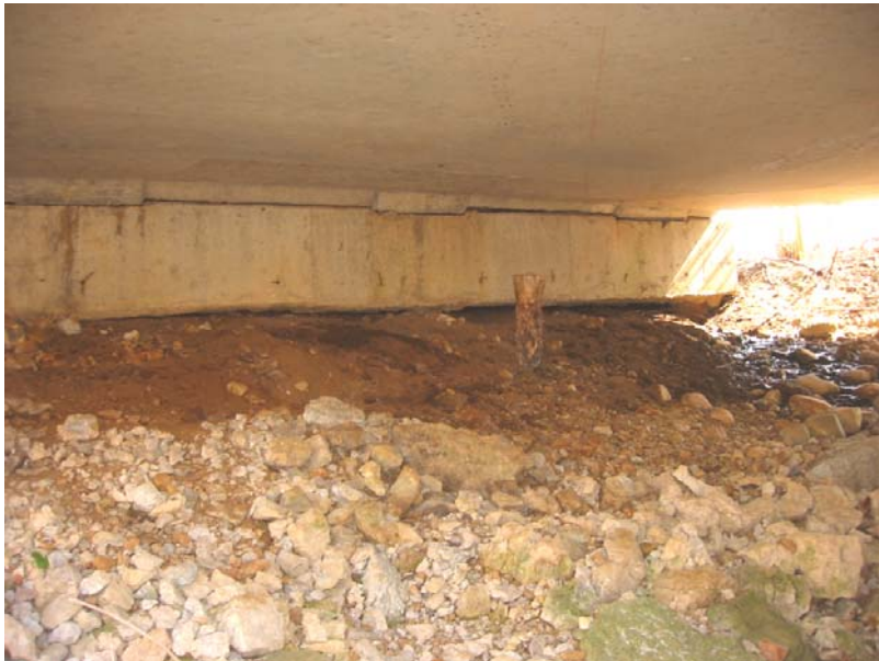
111 North end bent cap undermined
