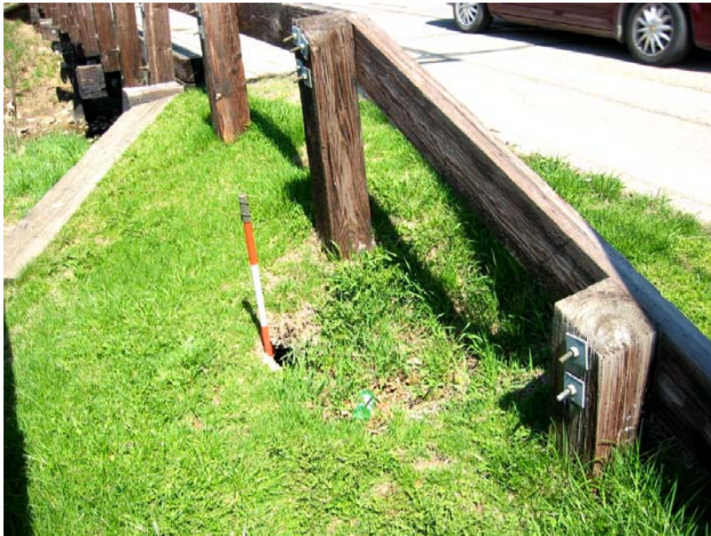
052 Hole in shoulder at the southwest corner
