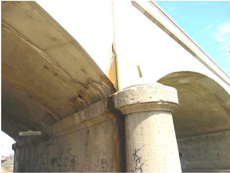
503 Seepage at the south end of the west pier
