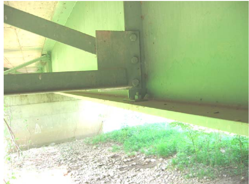
095 Typical diaphragm at the bottom
