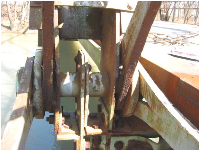
045 Panel point L2 north - heavy pack rust, section loss in loop bars and compression member
