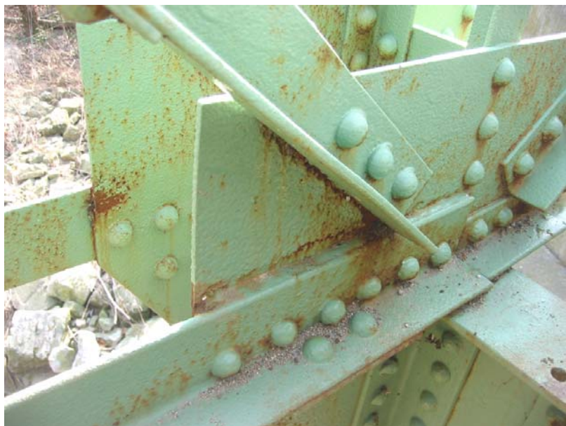
108 Southeast floor beam connection - inside of inner plate.
