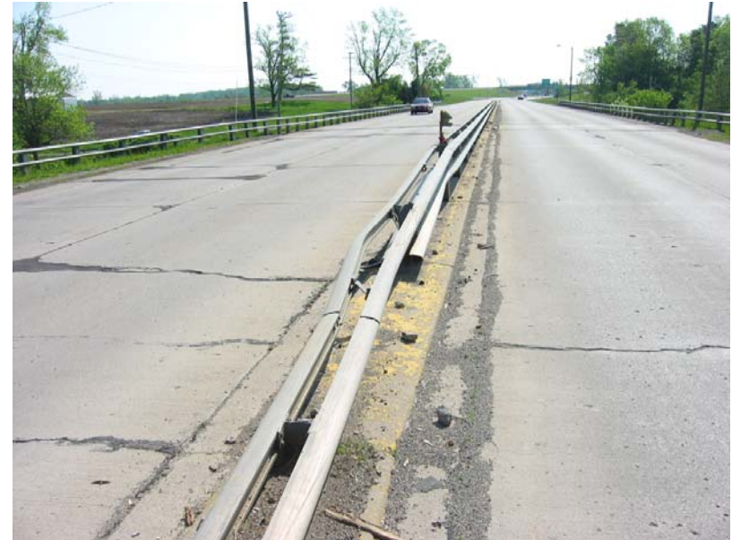
193 Damage to the west end of the median rail
