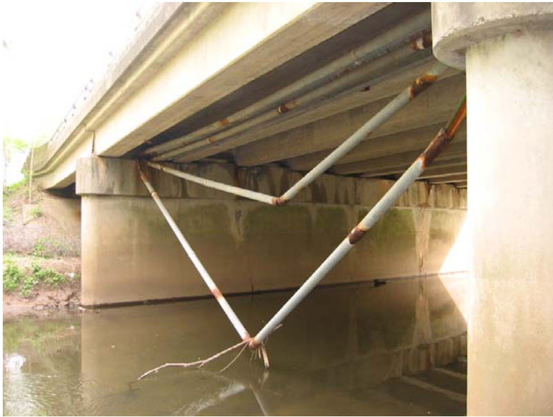
501 Broken and sagging conduit
