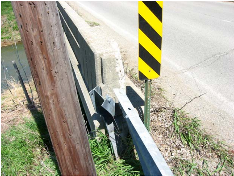
069 Collision damage to southwest rail
