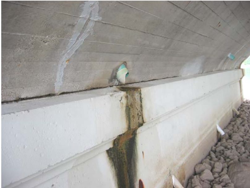
514 Weephole pipe extension broken – seeping onto pier
