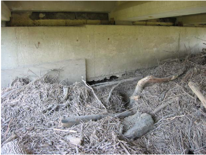
003 North endbent undermined and debris accumulation
