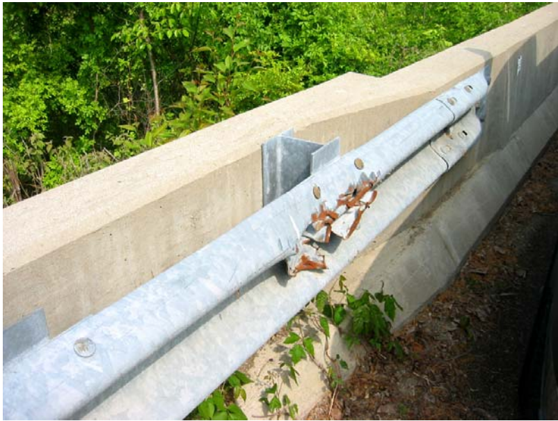
095 Damage at the southwest rail transition
