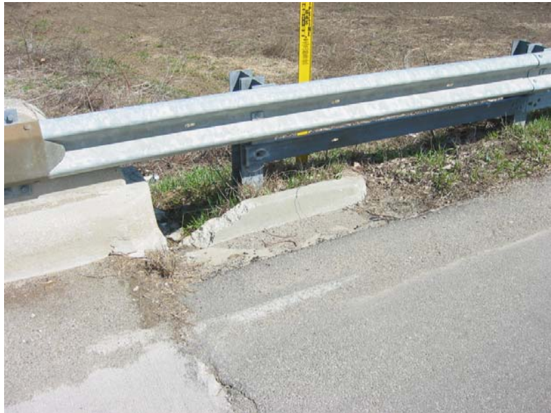
209 Northeast curb broken, allowing erosion
