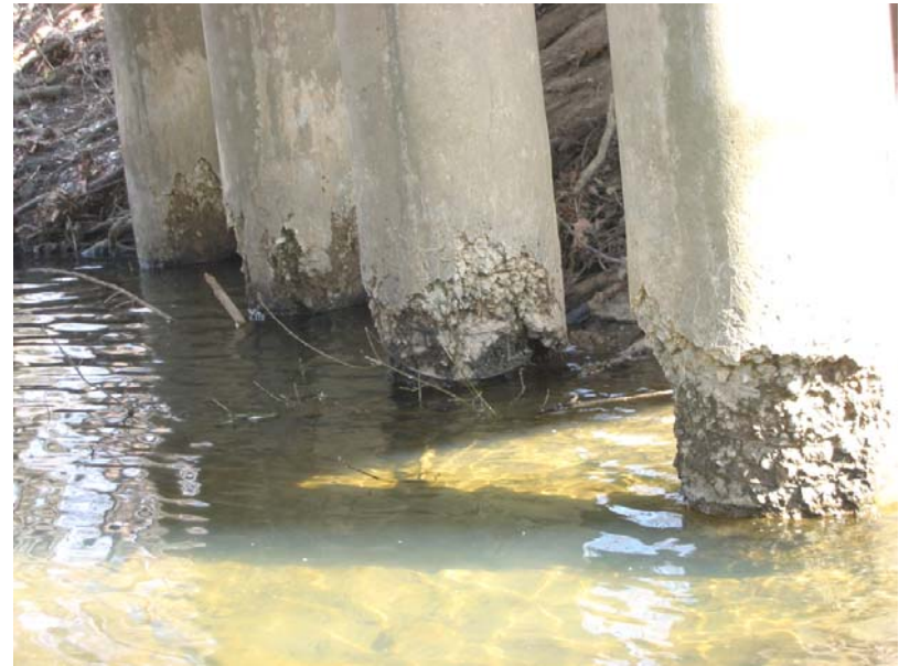
118 Pile encasements deteriorated
