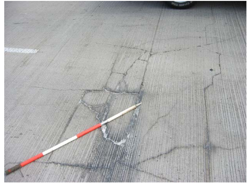
520 Cracks in the wearing surface - southbound
