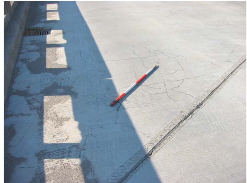
123 Wearing surface cracked
