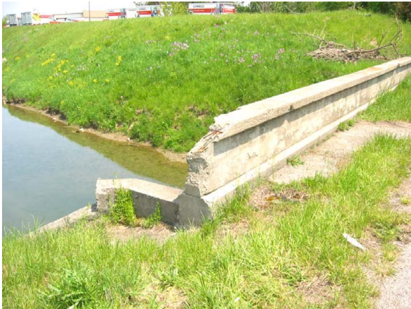
507 Damage to the northwest rail
