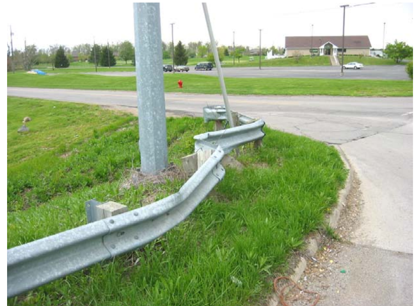
124 Rail damaged at north intersection
