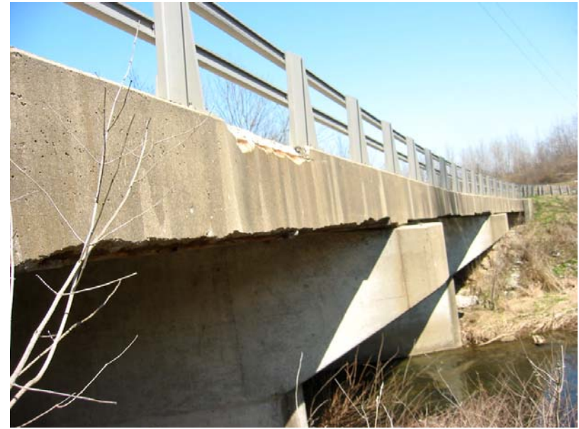
146 Spalls in the east coping at the south span
