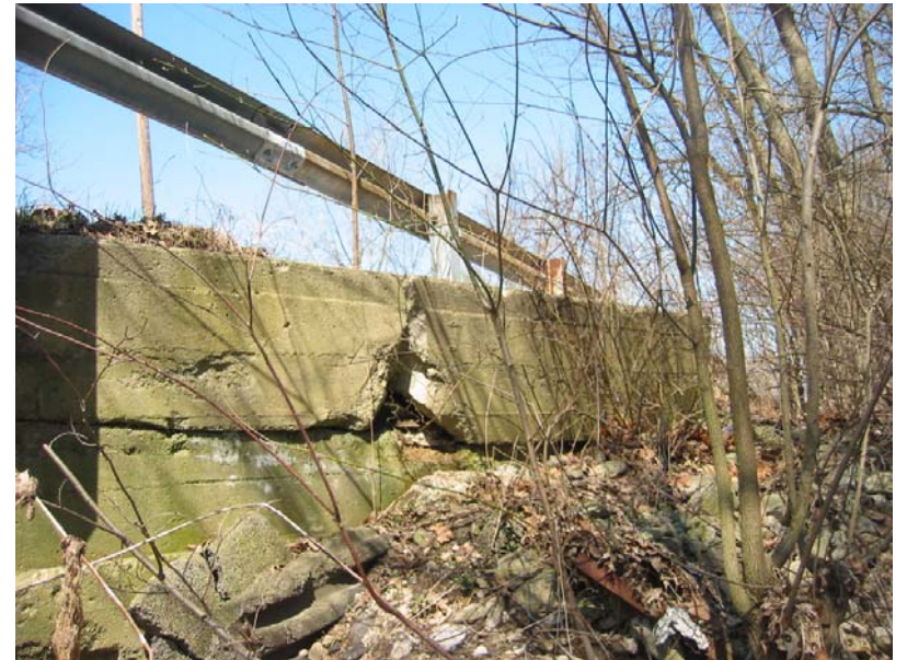
213 Northeast wingwall failing
