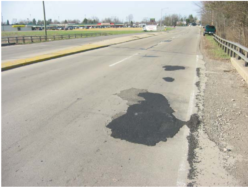
195 Wearing surface spalls and patches
