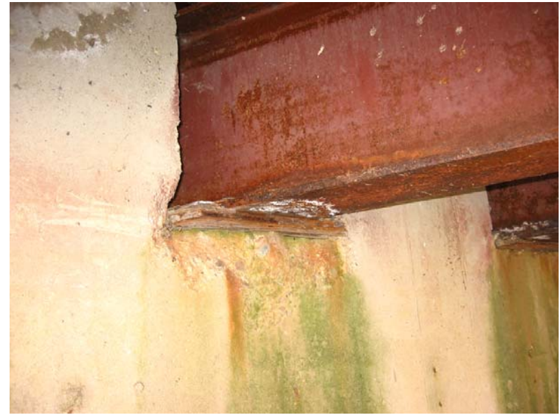
244 Spall at the beam seats and rust with delamination at beam ends
