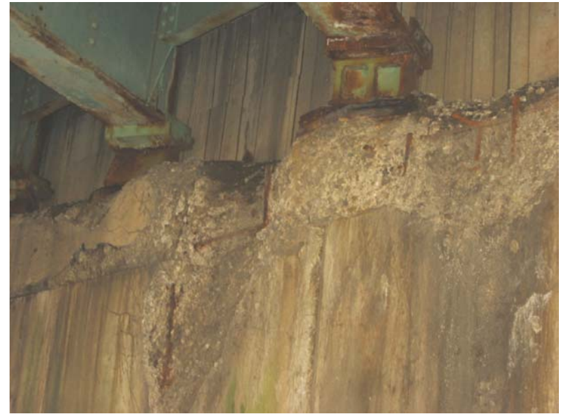
195 Abutment caps and beam seats deteriorated
