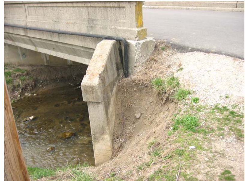
245 Erosion at the southeast corner
