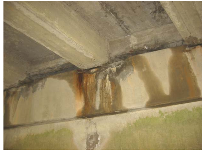
501 Cracks and efflorescence at the beam seat
