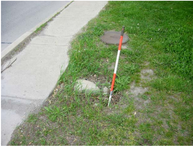
517 Hole in shoulder at the northeast corner
