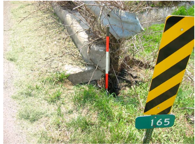
165 Erosion at the northwest corner
