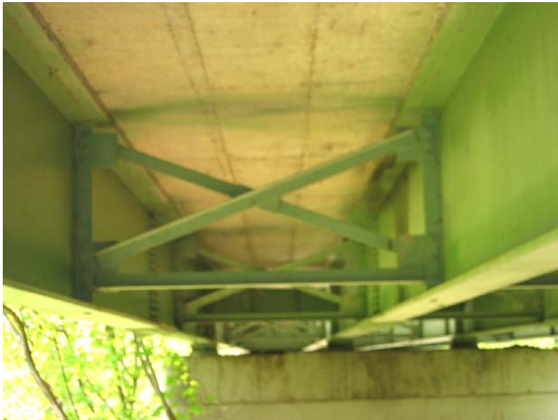
095 Typical configuration of diaphragms
