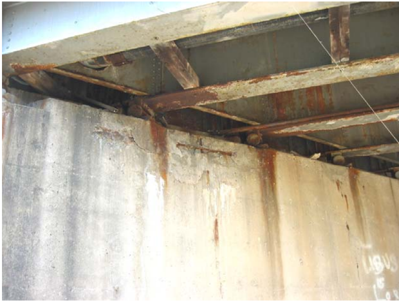
513 Spalls at the beam seats in the east pier
