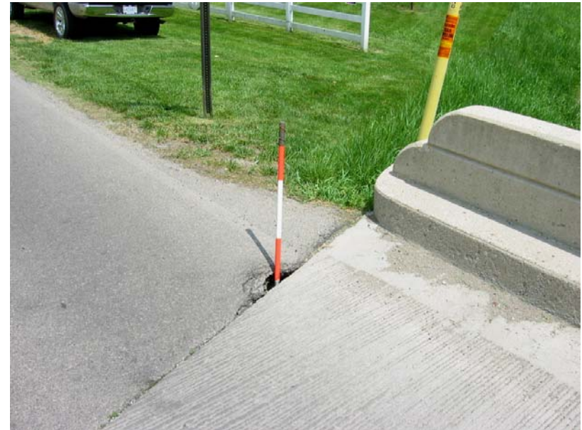
518 Hole in the pavement at the north end
