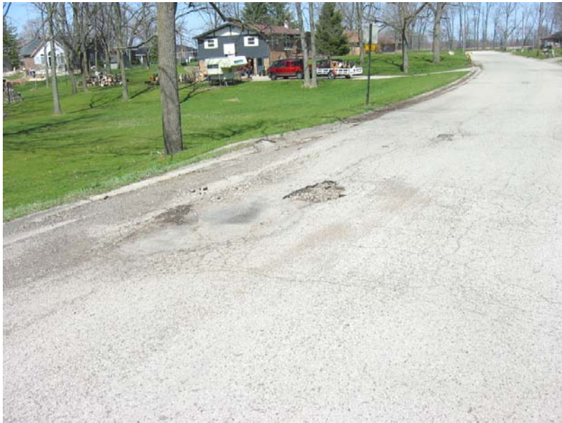
269 Settled road and potholes over the north pipe
