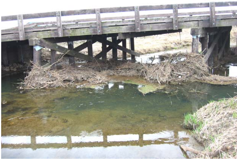
129 Debris buildup at center span
