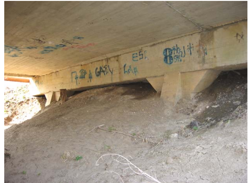
502 Erosion at the north endbent
