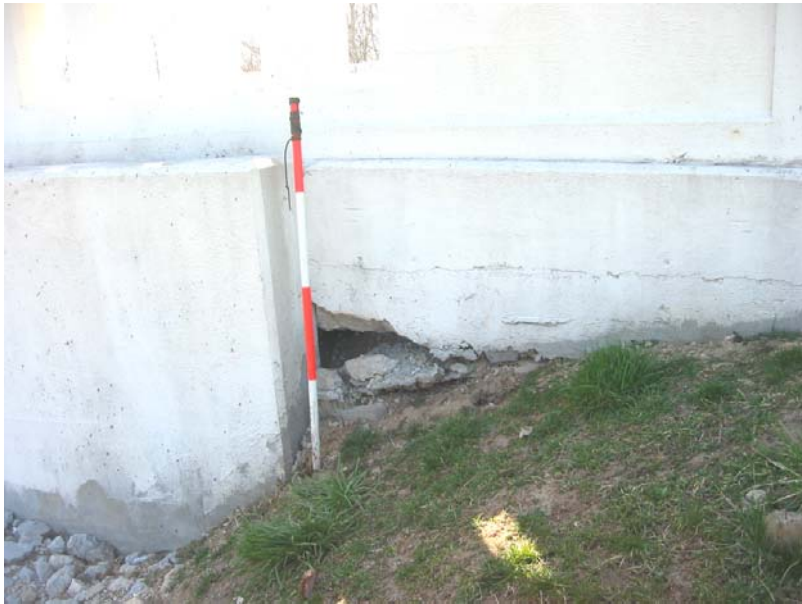
504 Void, minor damage at the north approach pad
