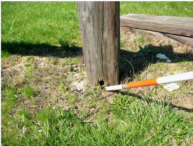
047 Rotted rail post at the northwest corner
