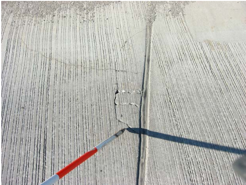
179 Cracked and loose overlay
