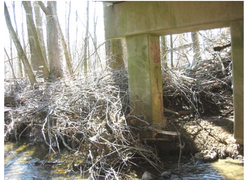
112 Brush dumped upstream of the west interior bent
