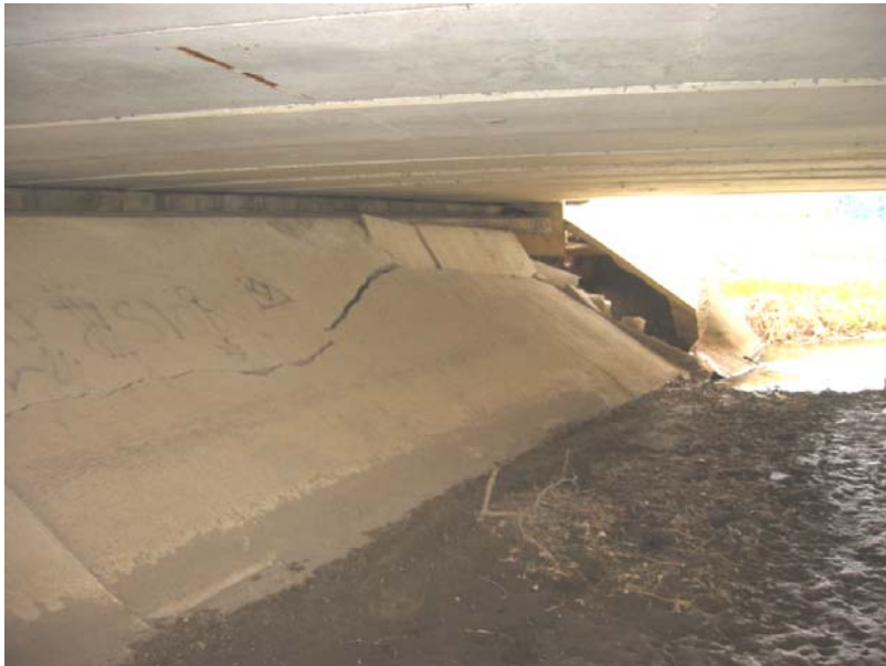
509 Failed sloped wall, lost fill – 3 of 3 photos
