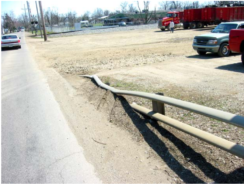
268 Damage at the southeast approach rail
