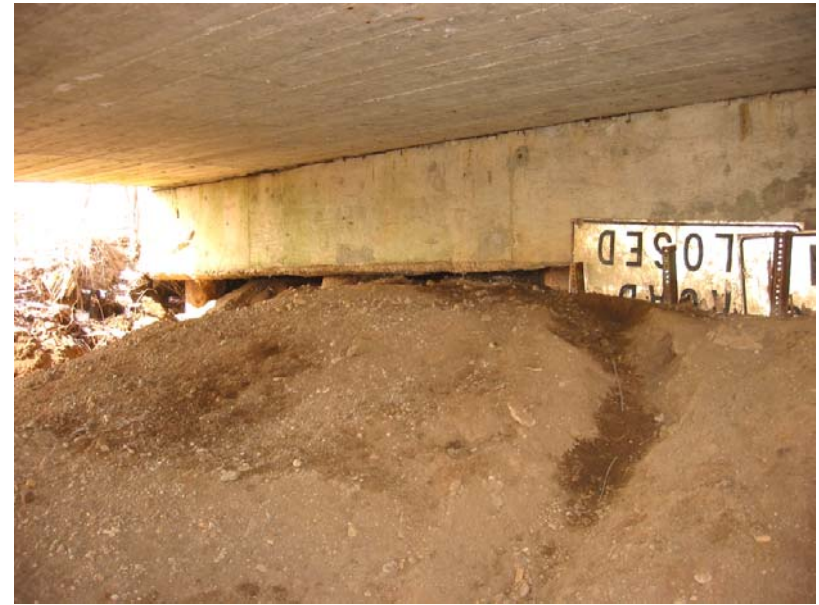
118 West end bent cap undermined - south end
