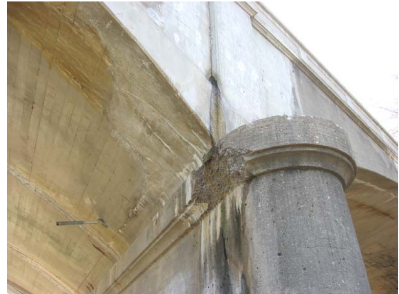
503 Seepage and deterioration at the north end of the west pier
