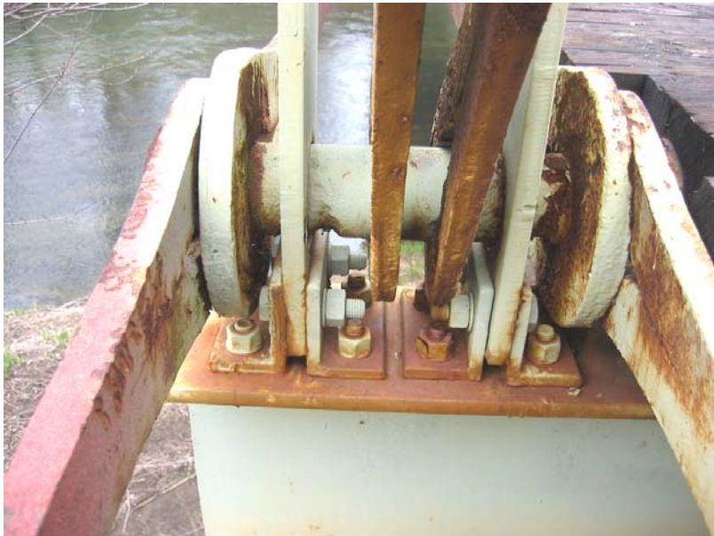
130 Panel point L9 south - section loss at pin
