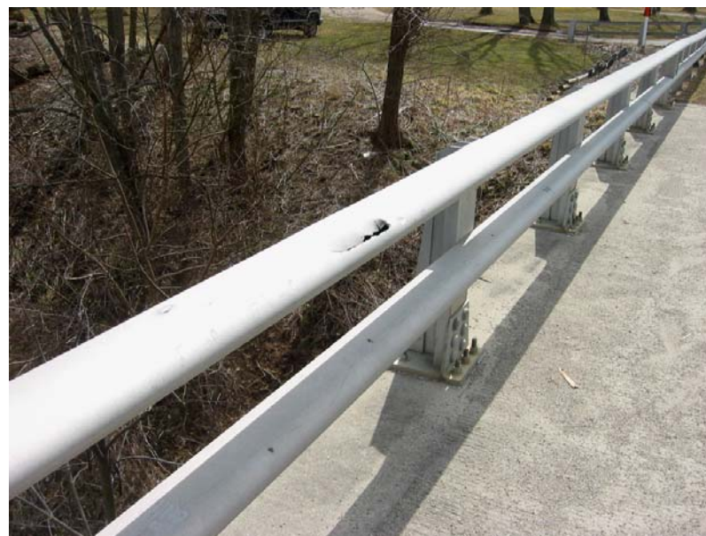
039 Bridge rail damage
