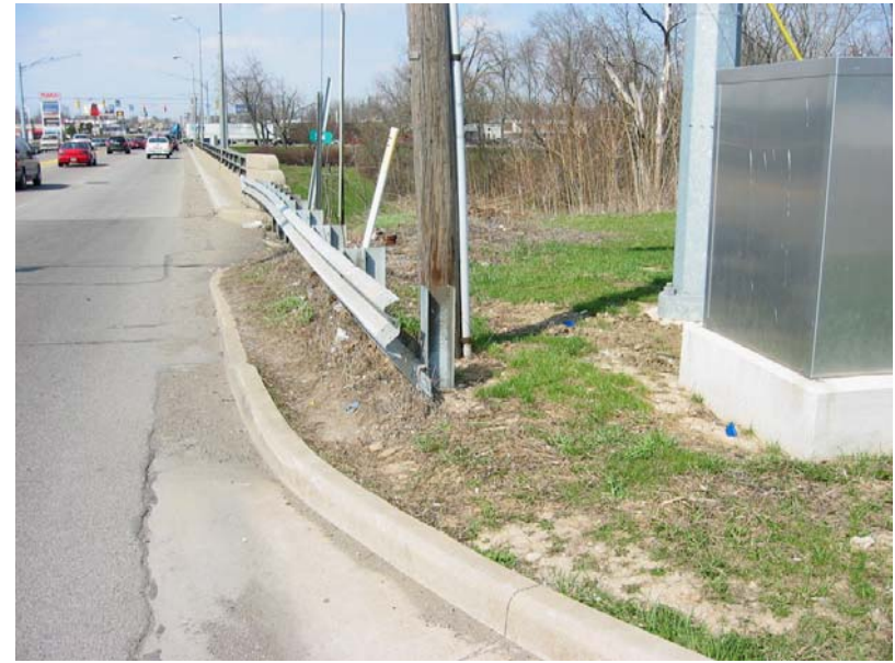
516 Southeast end treatment missing
