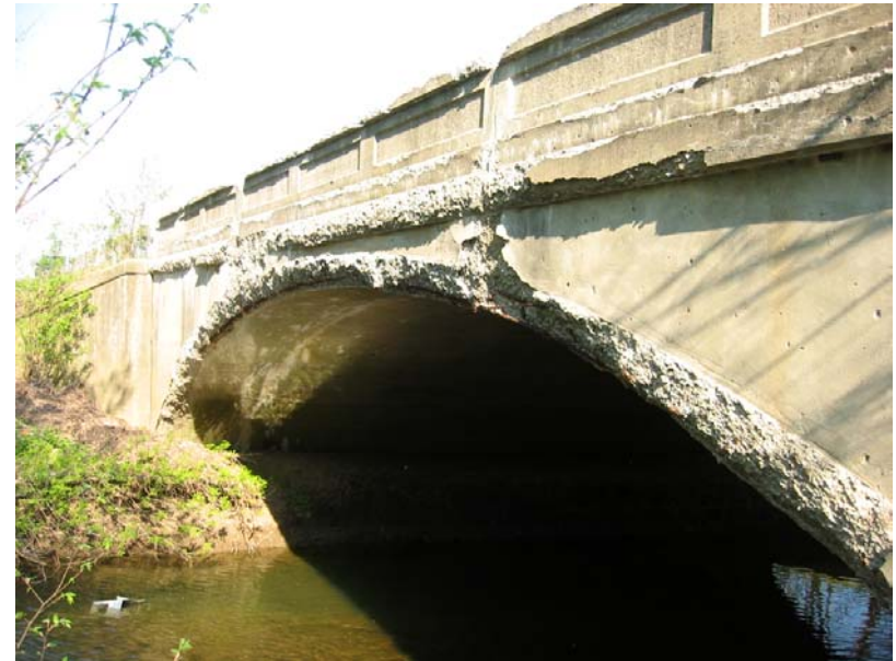
122 South coping deterioration
