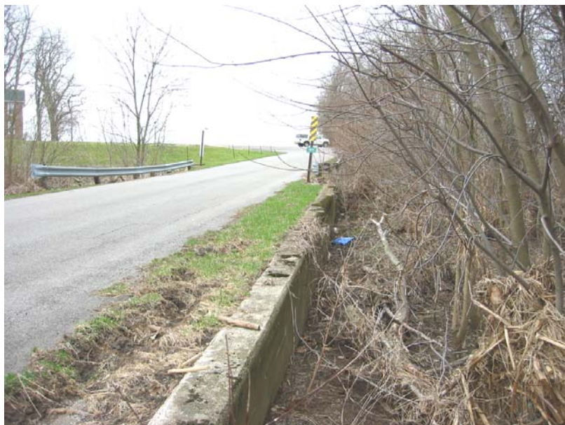
137 Dropoff at retaining wall
