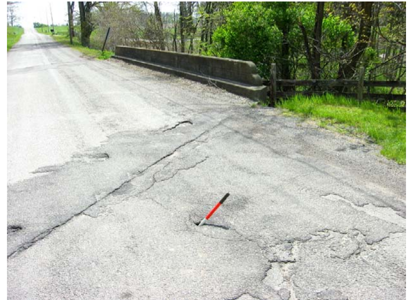
170 Hole in pavement at the west approach
