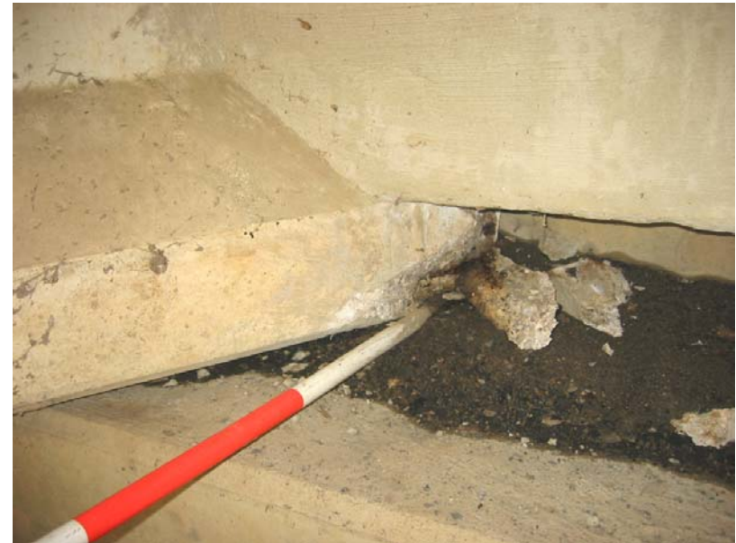
123 North end of center beam broken
