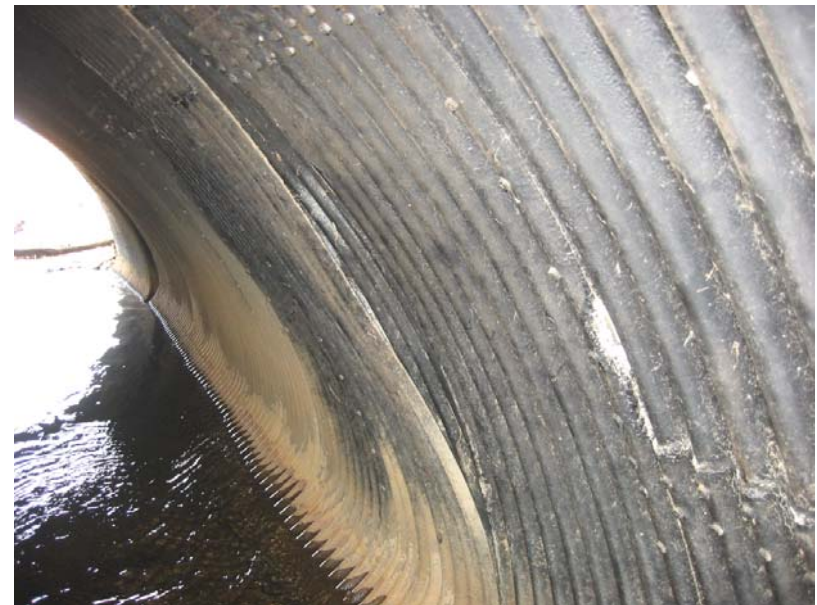
207 Open joints at arch plates
