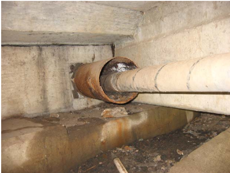
518 Conduit - possible source of fill loss at the northeast corner
