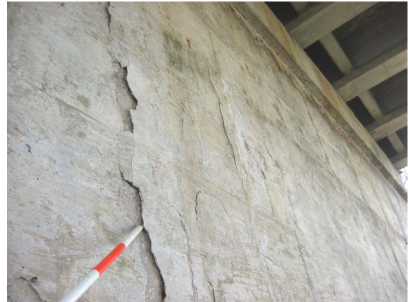
516 Typical pier face spalls and delamination
