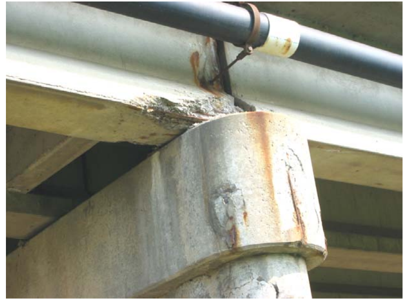
516 West end of the north pier, damaged beams
