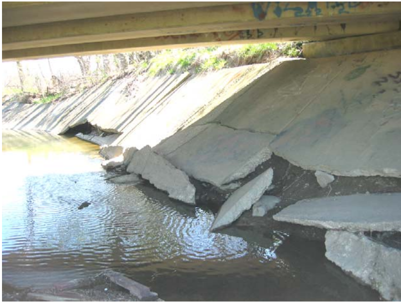
056 West slopewall failed
