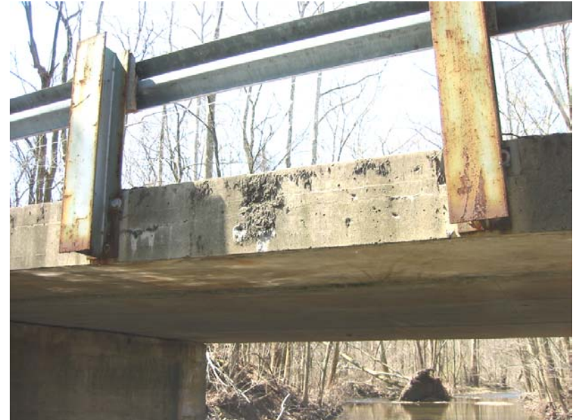
213 Crack at the midspan of the east outside beam
