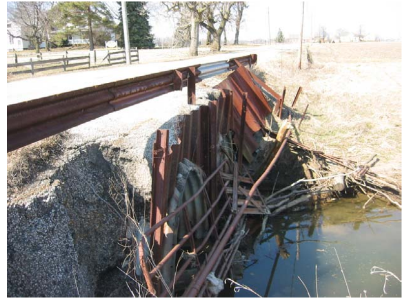
196 Debris at east side, retaining wall failure
