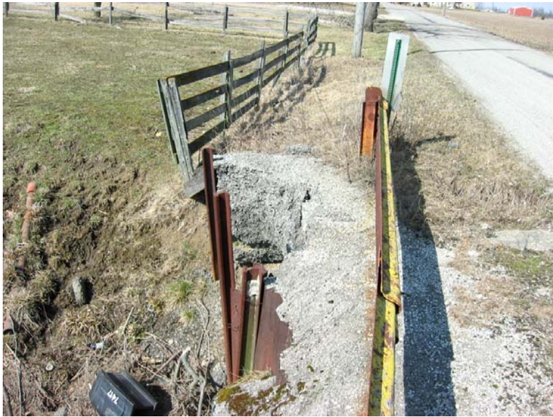
196 West sheet pile failure
