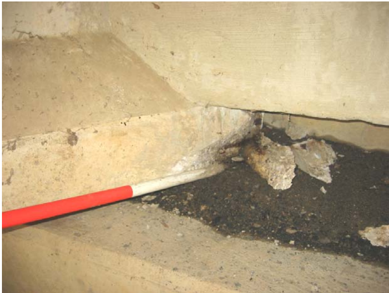
123 North end of center beam broken
