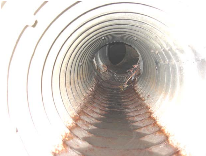
517 Apparent breakdown in drainpipe at the northeast corner
