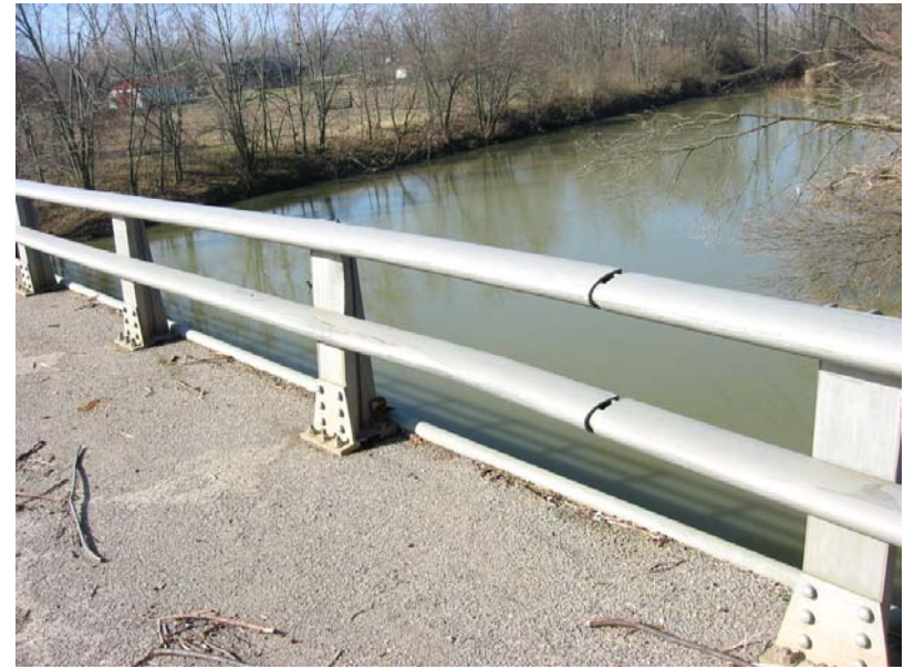
084 Damaged bridge rail and post
