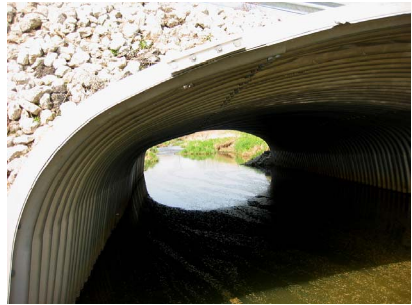
058 Distortion at the south side of the arch
