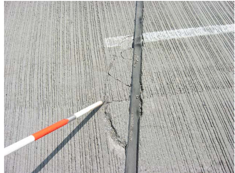
520 Spalled wearing surface at the joint - southbound
