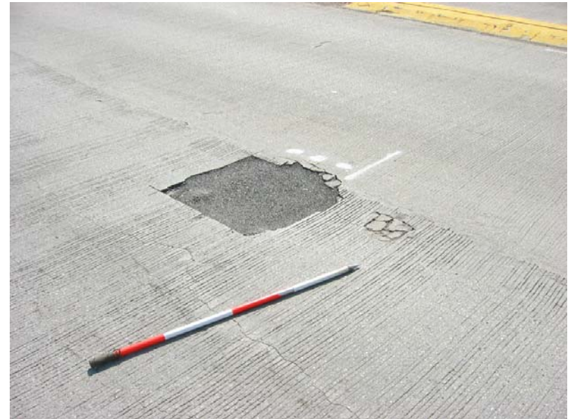
516 Northbound wearing surface spalls and patches
