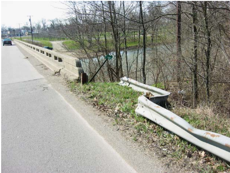
141 Northwest approach rail damage
