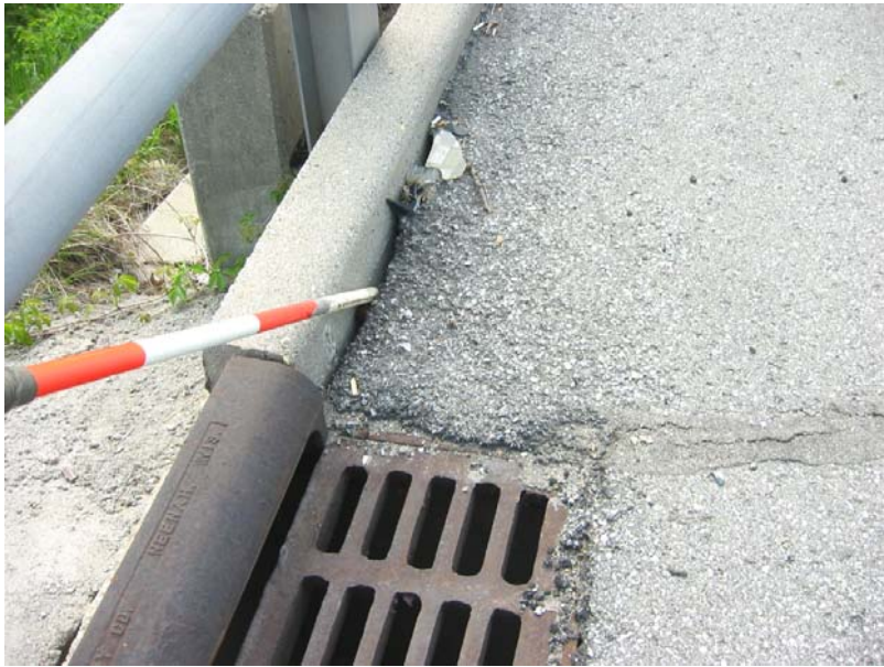
520 Gap between asphalt and curb allows water through - void below
