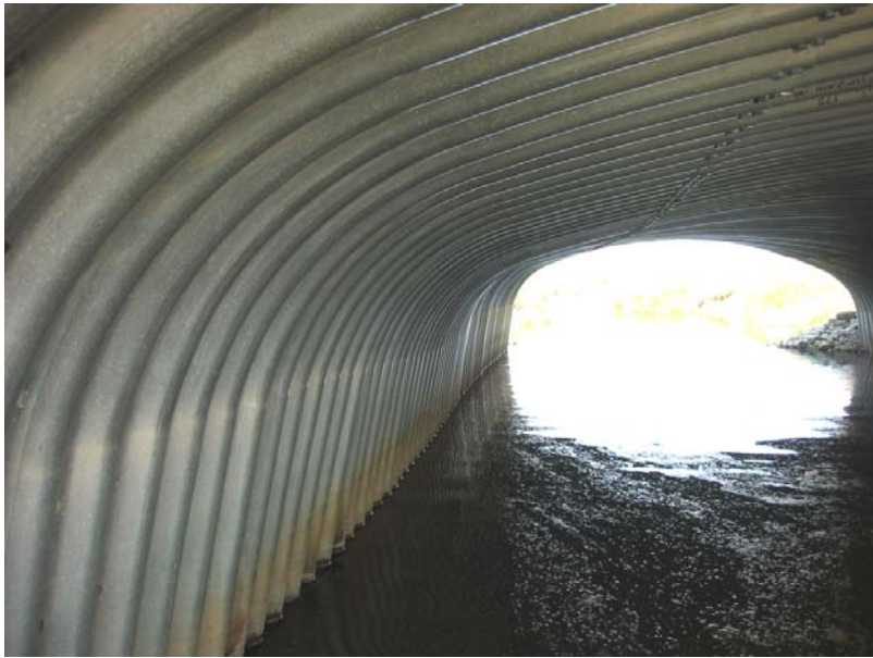
058 Distortion at the south side haunch of the arch
