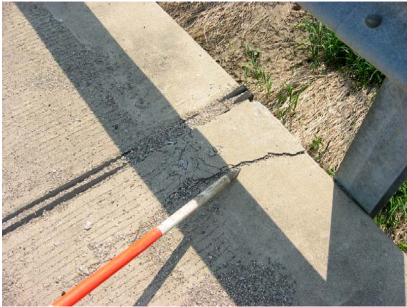
163 Crack in wearing surface at joint - typical of three locations
