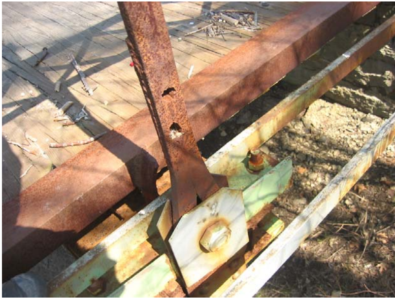
045 Panel point L11 south - 2 holes in vertical with patch steel welded in place
