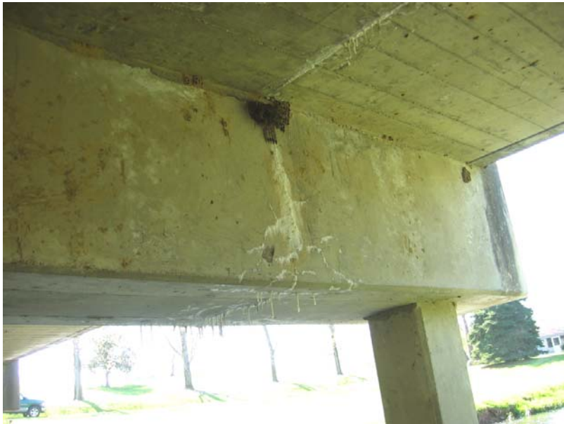
013 Cracks and efflorescence at the west interior bent
