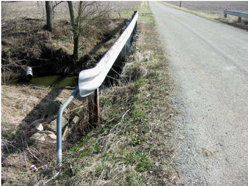
035 Eroded shoulder
