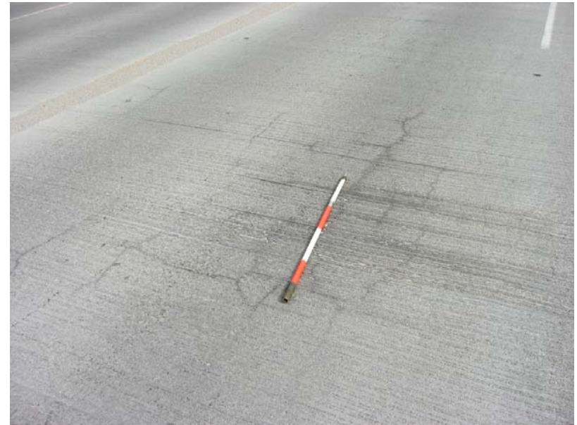
501 Cracks in the wearing surface
