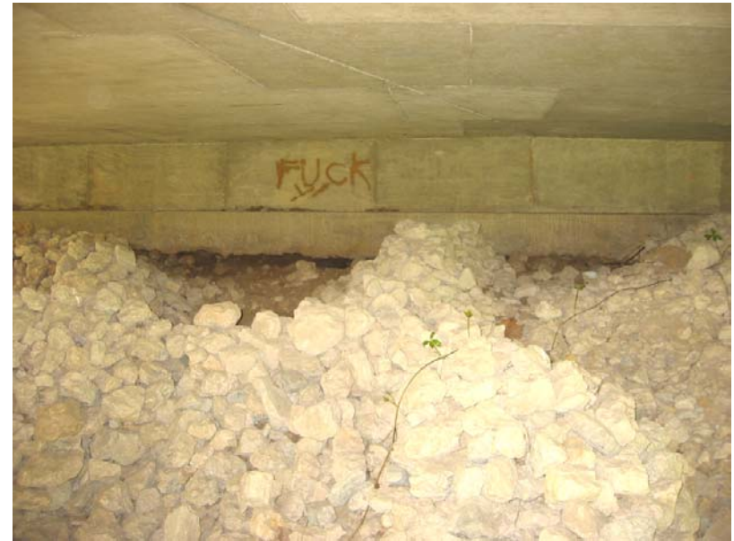
511 Southwest endbent cap undermined and riprap displaced
