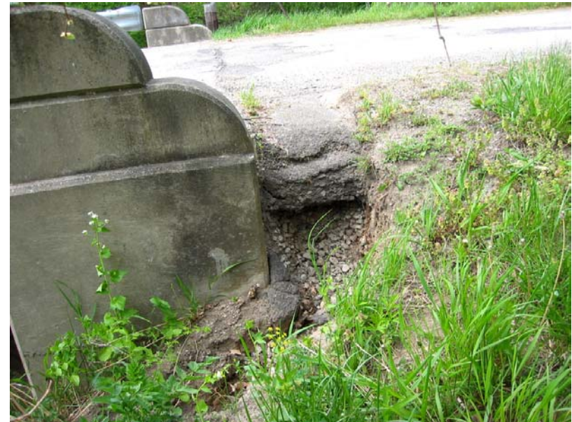
105 Shoulder erosion at the southeast shoulder
