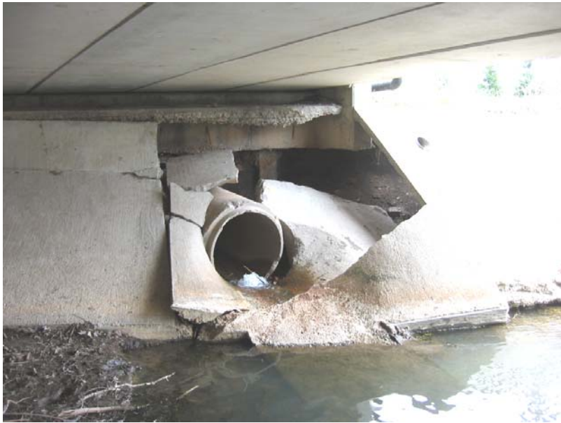
509 Failed sloped wall, lost fill – 1 of 3 photos
