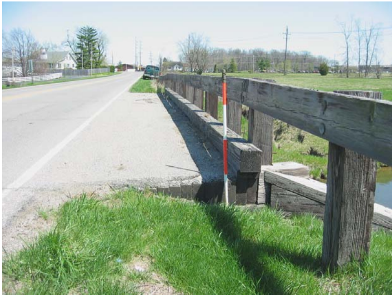
047 End of slab exposed to traffic
