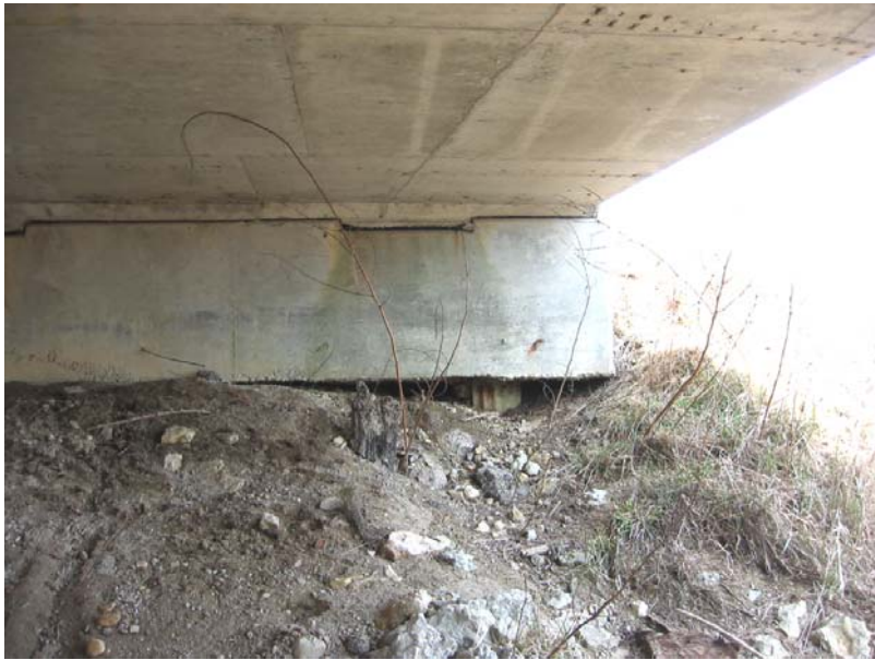
110 North end bent cap undermined
