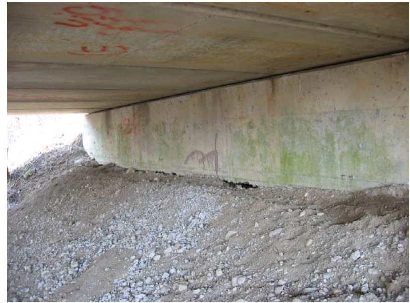
205 North end bent cap undermined
