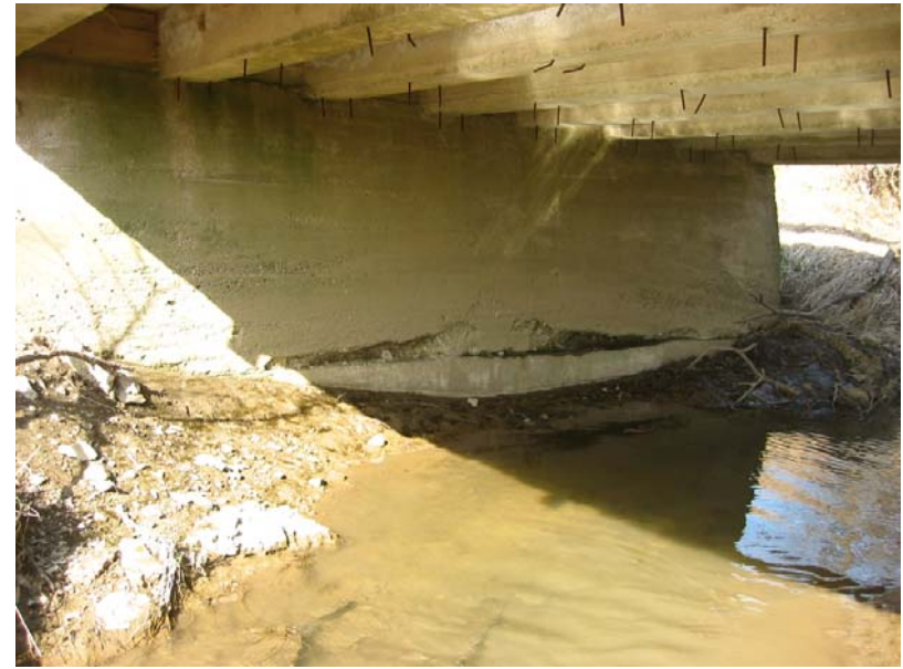
035 Deterioration at north endbent
