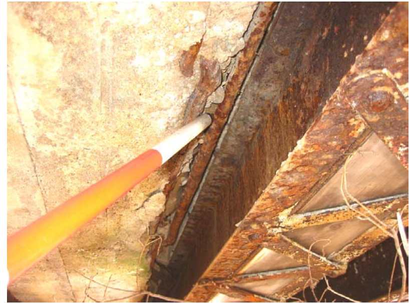
191 No tie-in at deck widening
