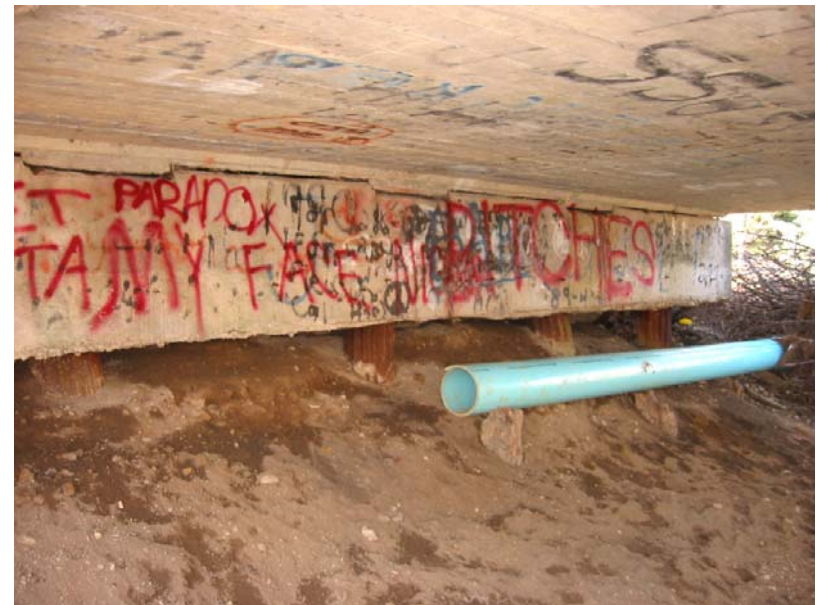
075 South end bent cap undermined
