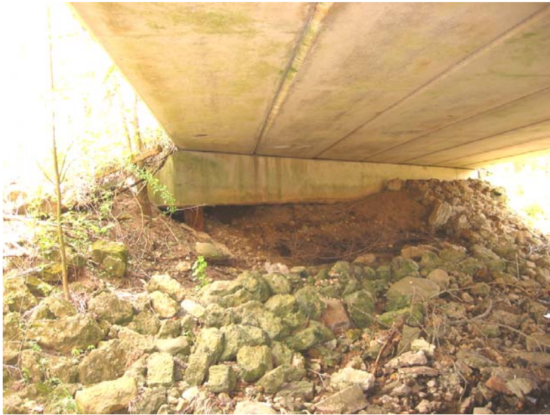
170 North end of east cap undermined
