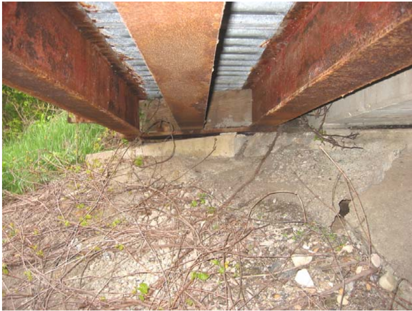
124 Substructure settled at the northwest corner
