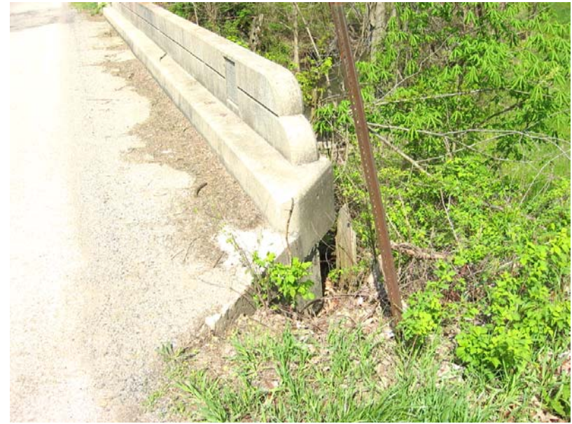
170 Northeast corner eroded
