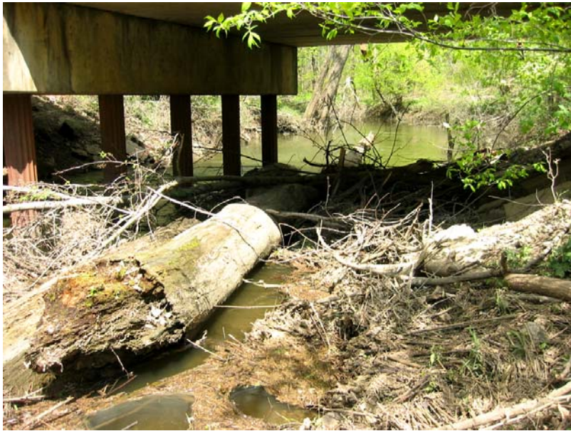
159 Large debris below bridge
