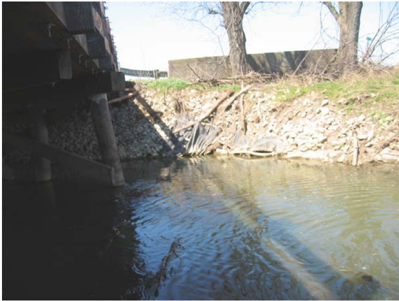
061 Riprap loss at the northwest corner
