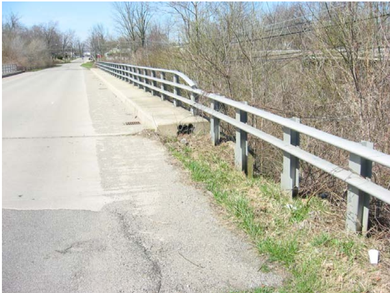
144 End of sidewalk exposed to traffic
