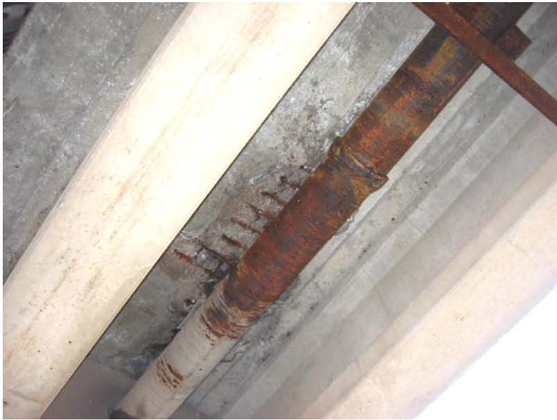
516 Deck spalls below in the south span
