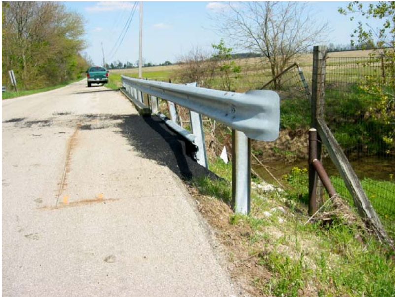
091 Southwest shoulder drops off in front of rail
