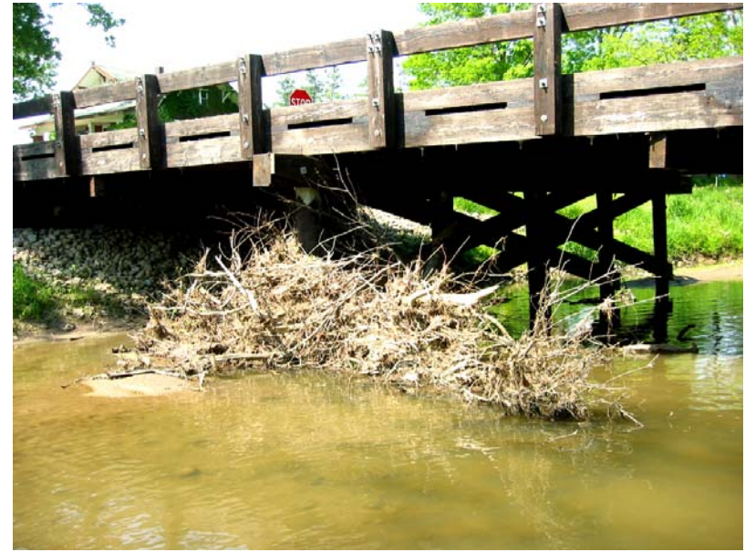
090 Debris accumulated at the south interior bent
