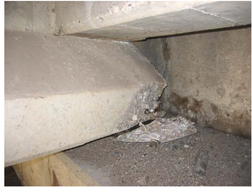
520 Typical damage to beams at the south endbent
