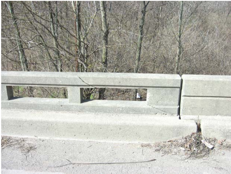
141 Damaged northwest rail
