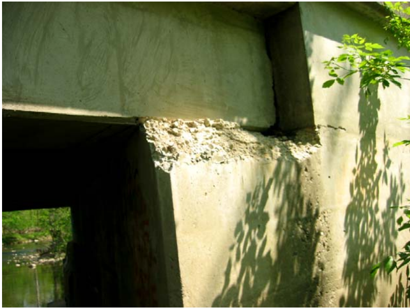
092 Southeast seat deterioration
