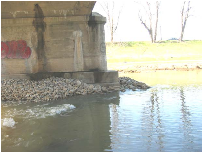
503 Riprap loss at the center pier
