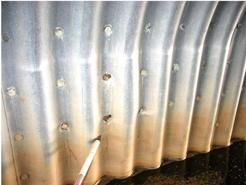
058 Bolt head torn through the arch plate
