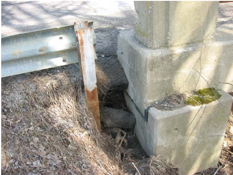
118 Erosion at southwest corner
