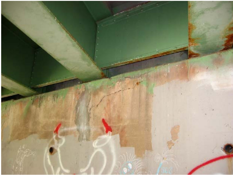
506 Top of north abutment cracked
