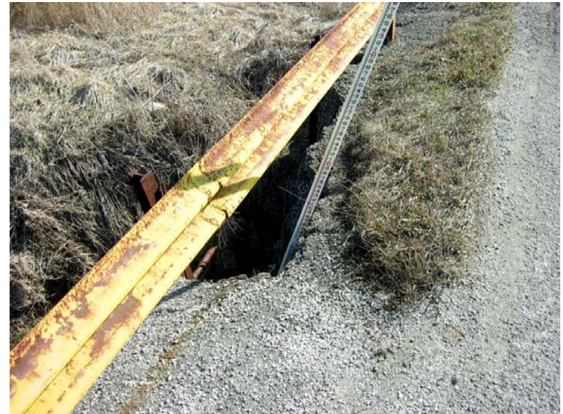
196 East side shoulder failed
