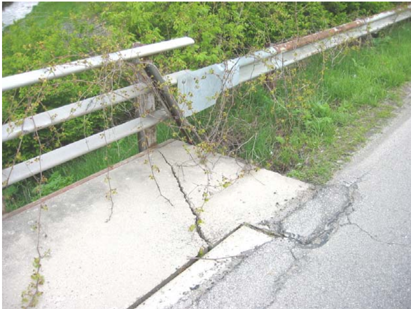
125 Widened deck cracked at northwest corner
