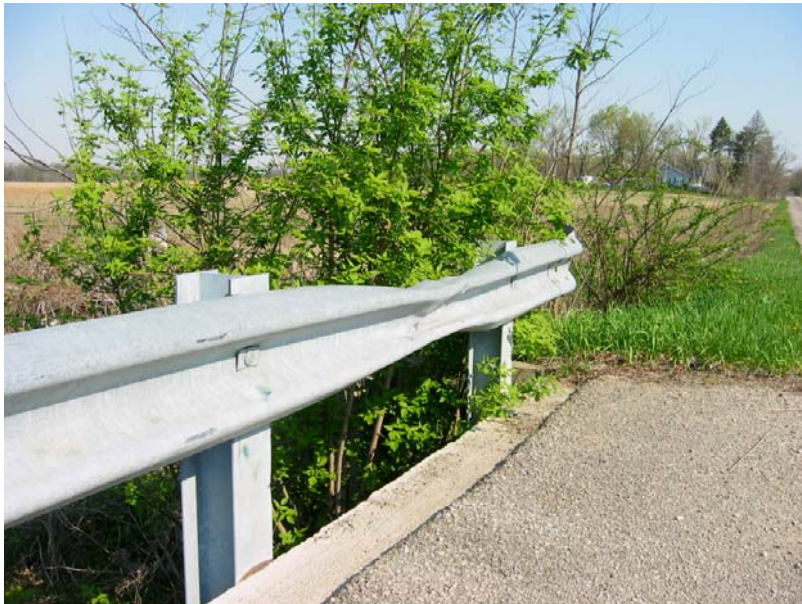
109 Damage at the west bridge rail
