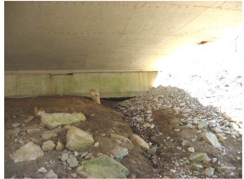
133 East end bent undermined
