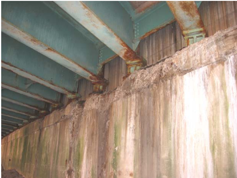
195 Abutment caps deteriorated
