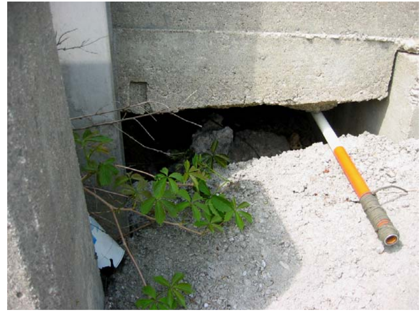
520 Void under the northeast wing and sloped wall.
