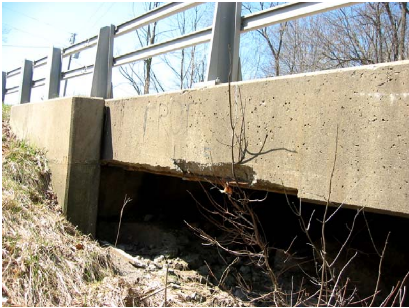
146 Spalls in the east coping - south span
