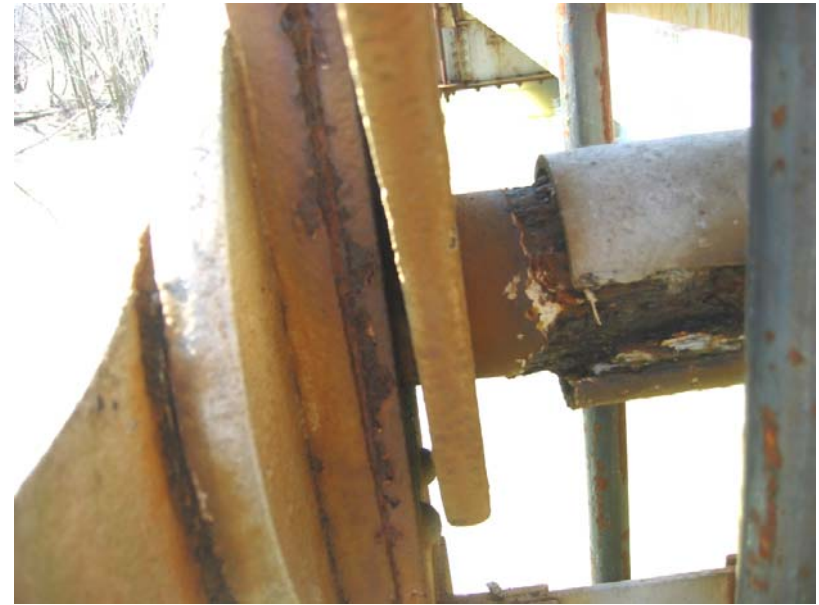
085 Section loss in pin L7-south
