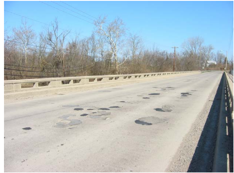
141 Wearing surface spalls and patches
