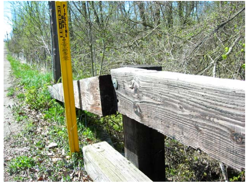
057 Loose rail protruding at the southwest corner
