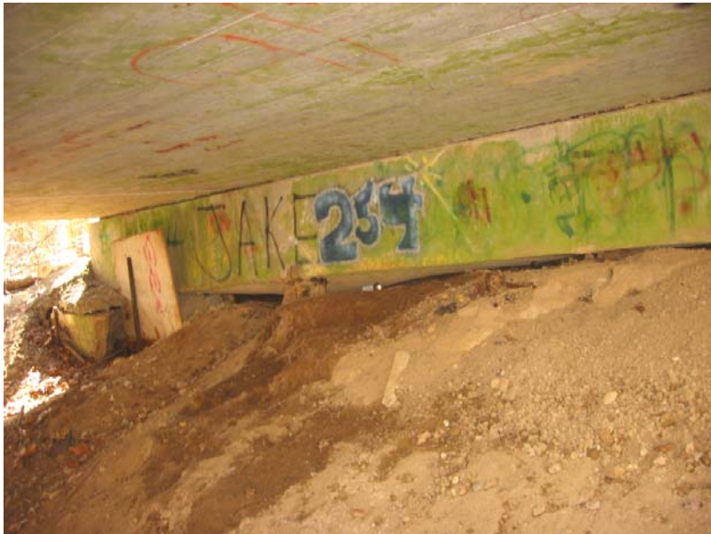
112 West end bent cap undermined
