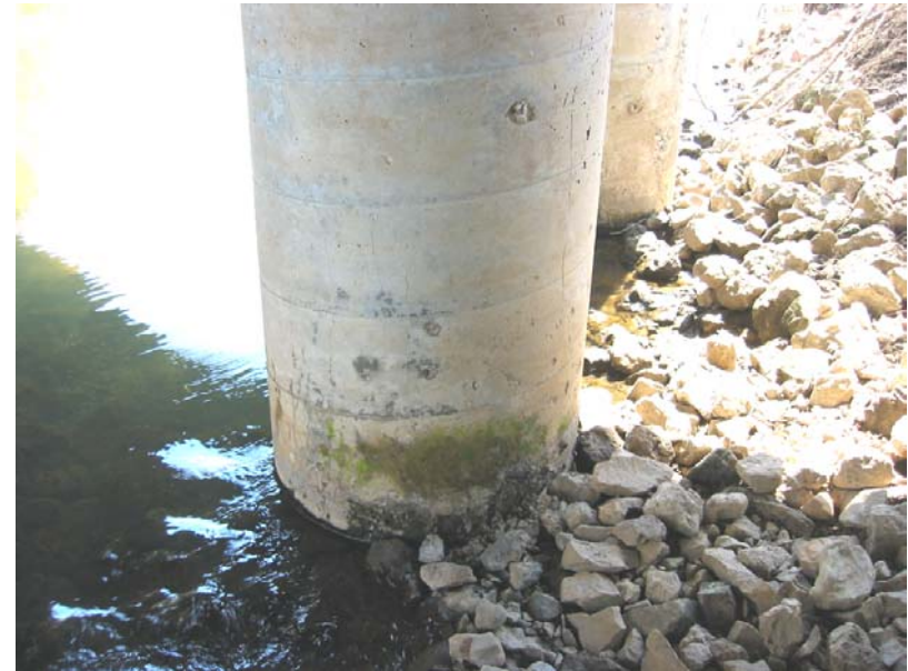
189 Cracks and deterioration at pile encasement
