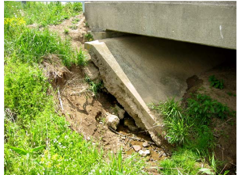
099 Erosion under the sloped wall at the southeast corner
