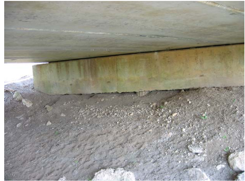
270 East end bent undermined
