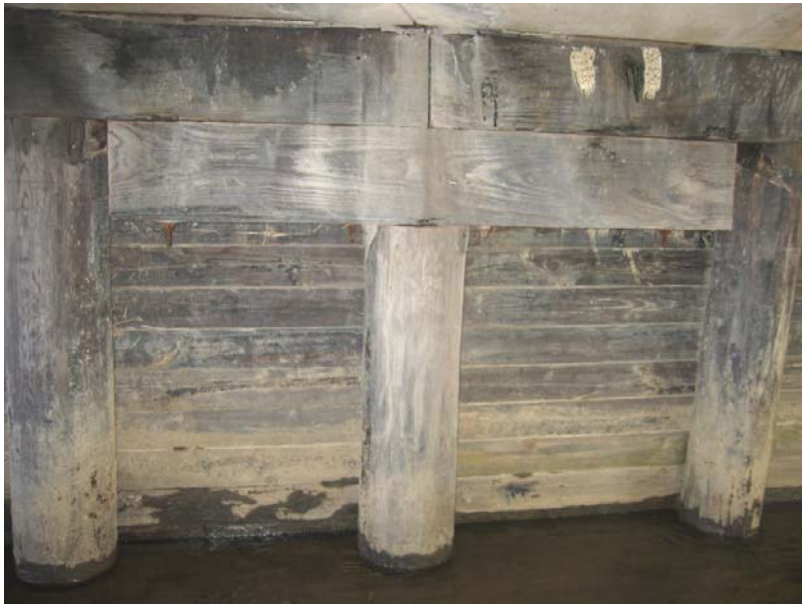
050 Configuration of center pile at north endbent
