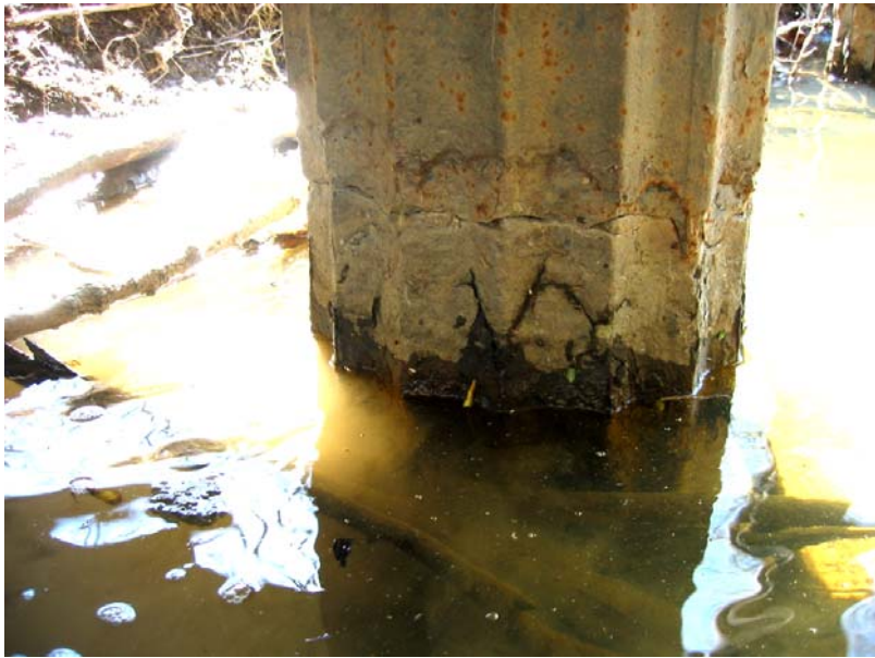
068 Pile cracked (typical)
