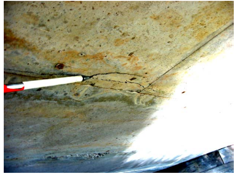
015 Cracks along the bottom corner of box beam
