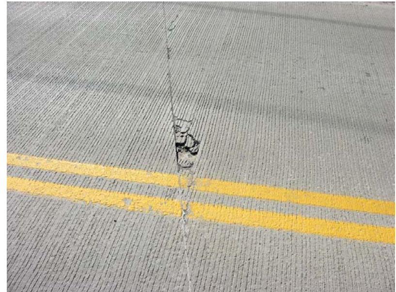
504 Pothole at the approach pad
