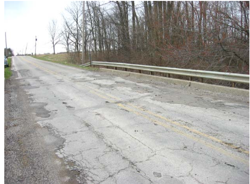
127 Wearing surface deterioration
