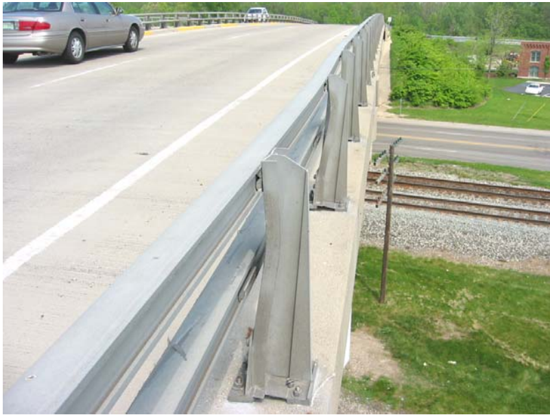
520 Two damaged bridge rail posts - northbound
