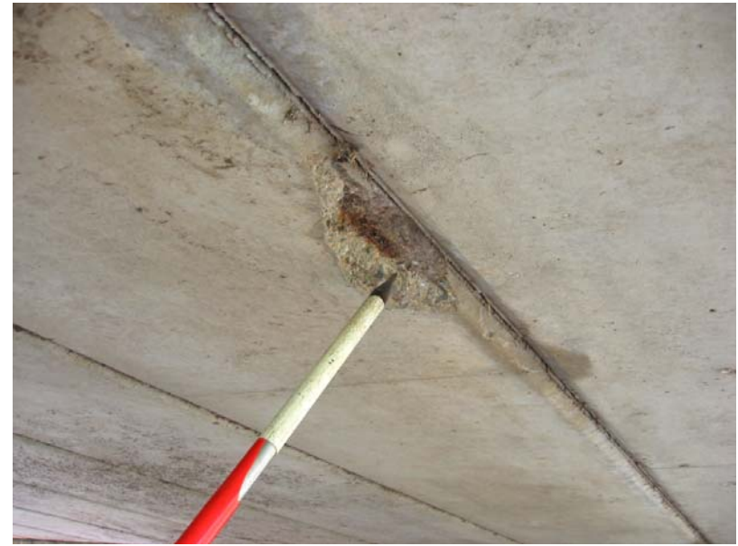
159 Spall in second beam from north in east span
