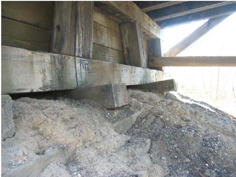
226 North end bent supports deflected and settled
