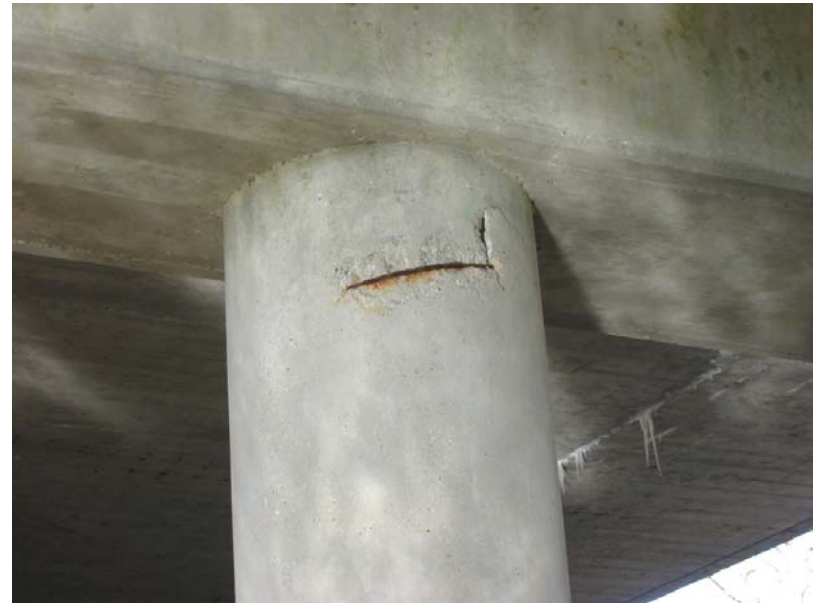
118 Concrete deteriorated at top of column
