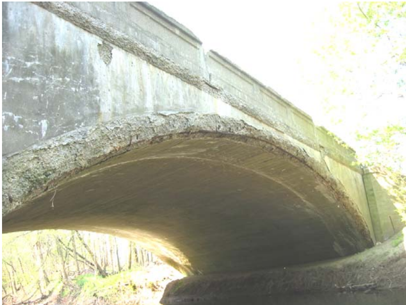
122 North coping deterioration
