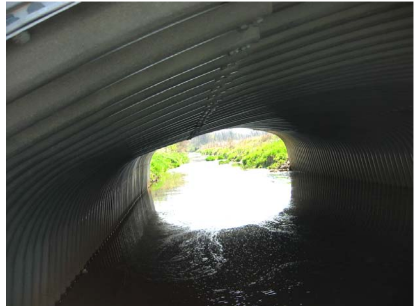
058 Distortion at the north side of the arch
