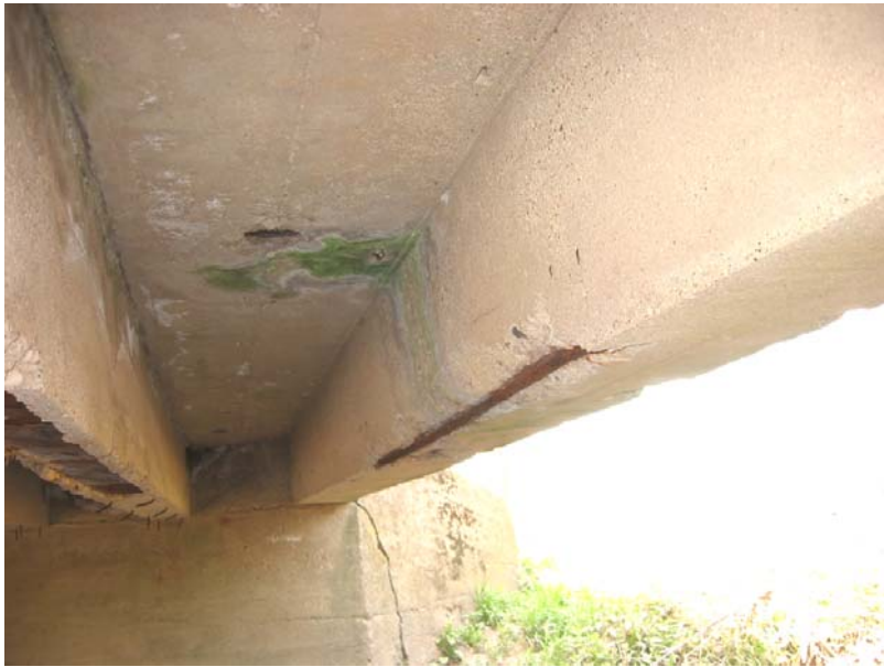
087 Outside reinforced concrete beam spalled - section loss in reinforcing steel
