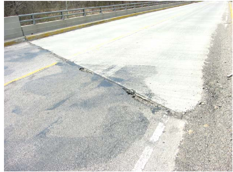
051 Potholes in asphalt overlay at the east approach pad
