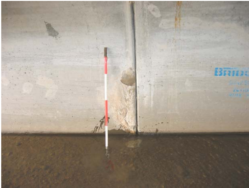
070 Deteriorated patch in arch below
