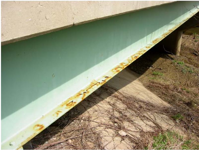
051 Paint failure at the beams
