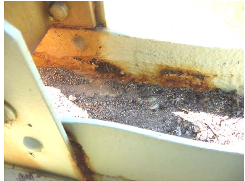
161 Rust-through at one leg at L5
