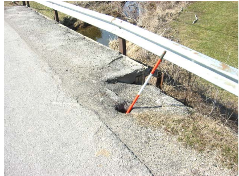
191 Hole in pavement at northeast
