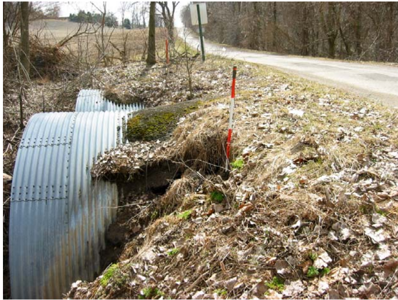
040 Shoulder loss on east side
