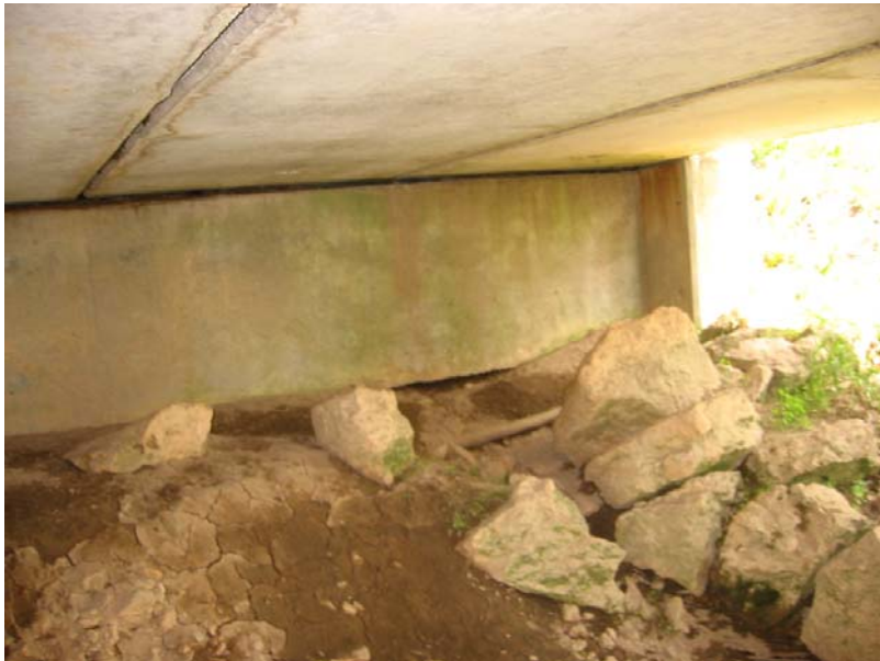
105 East end bent cap undermined
