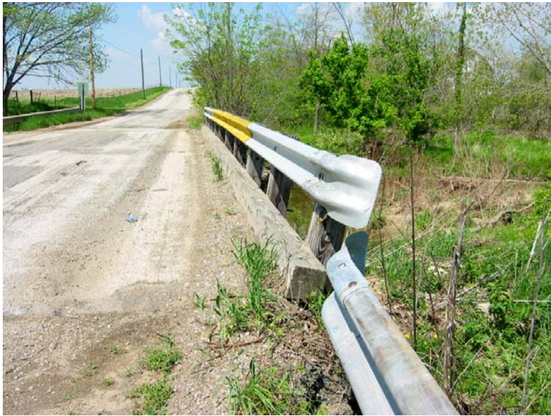
103 Northeast rail leaning - outer slab timbers rotated
