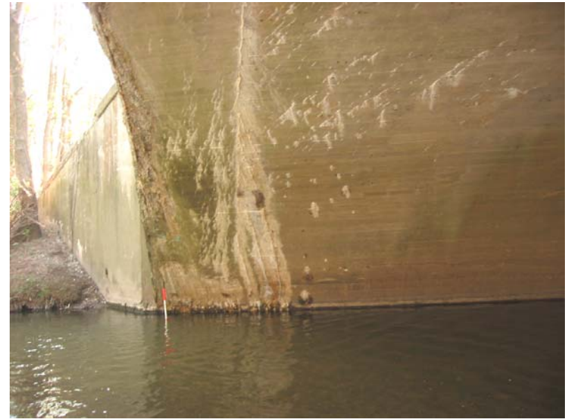
122 Heavy efflorescence at the northeast arch ring
