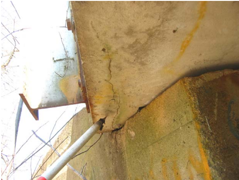
213 Crack at the west beam in the northwest corner
