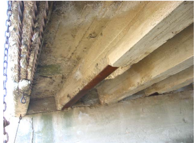
204 Beam encasement deteriorated
