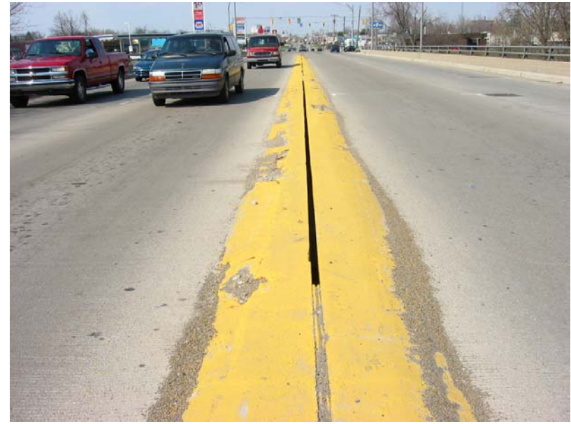
516 Center joint missing, roll curb spalled
