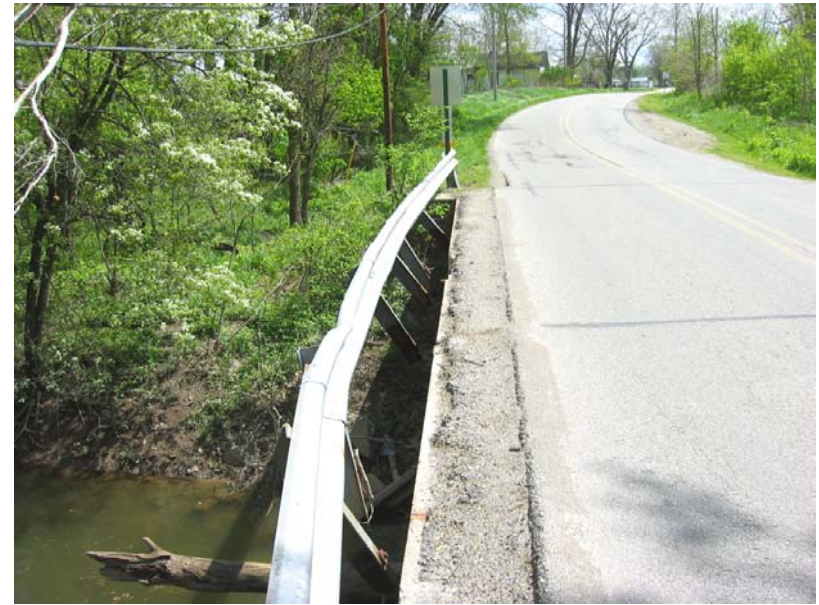
159 North bridge rail damage
