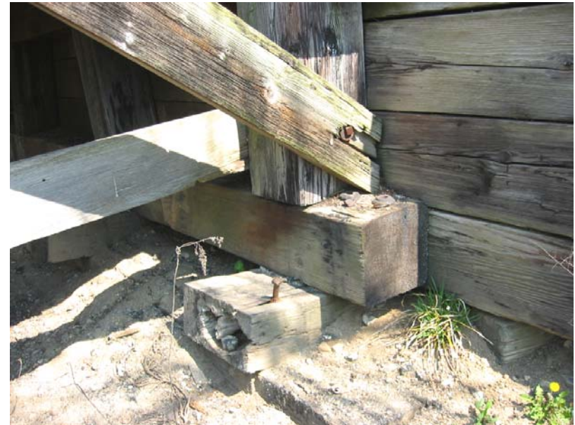
226 Northeast diagonal brace split and rotted and support base rotted
