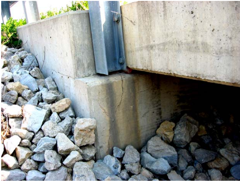
072 Cracked abutment at the northwest corner
