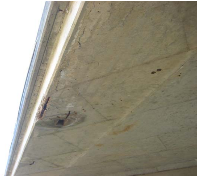
111 Cracks and spalls at the west coping
