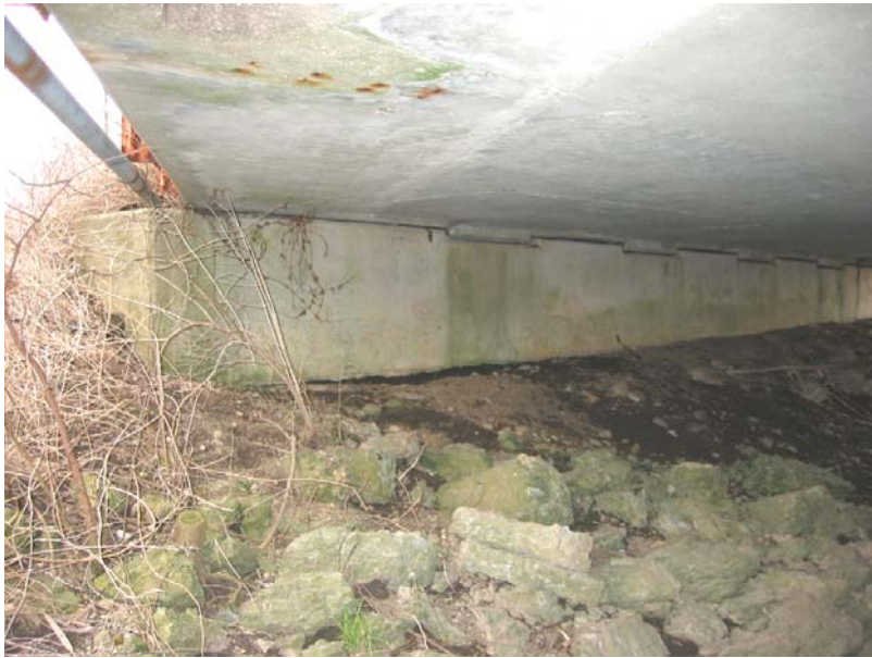
138 South endbent undermined
