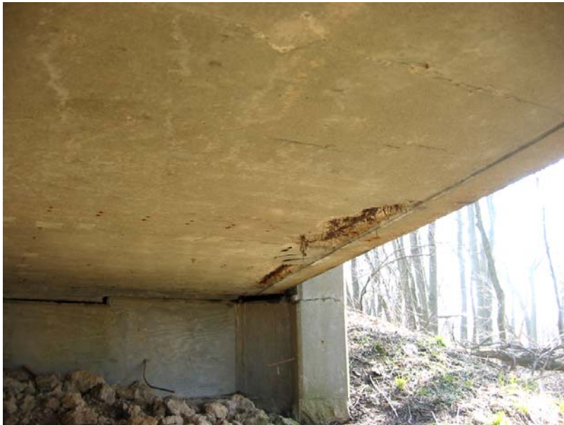
101 Spalls near the south coping in the east span
