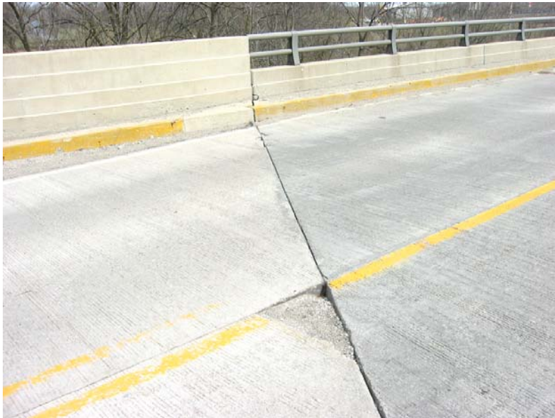
051 Spalls at west concrete approach next to joint
