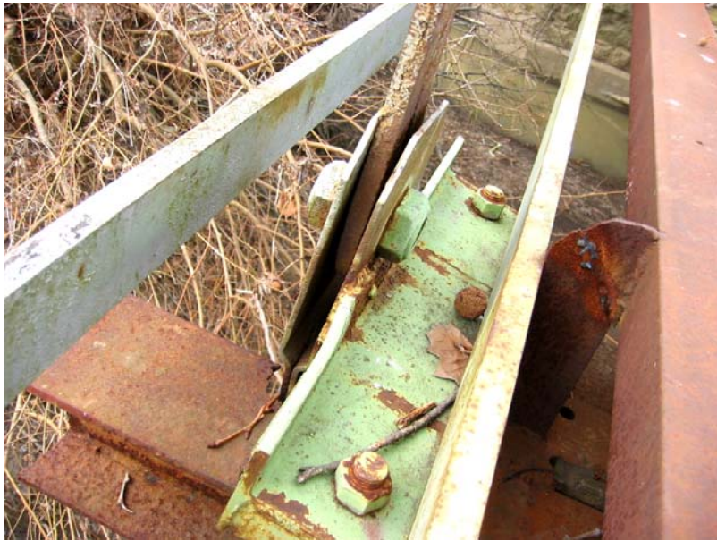
045 Panel point L3 south - retrofitted hanger welded to old hanger
