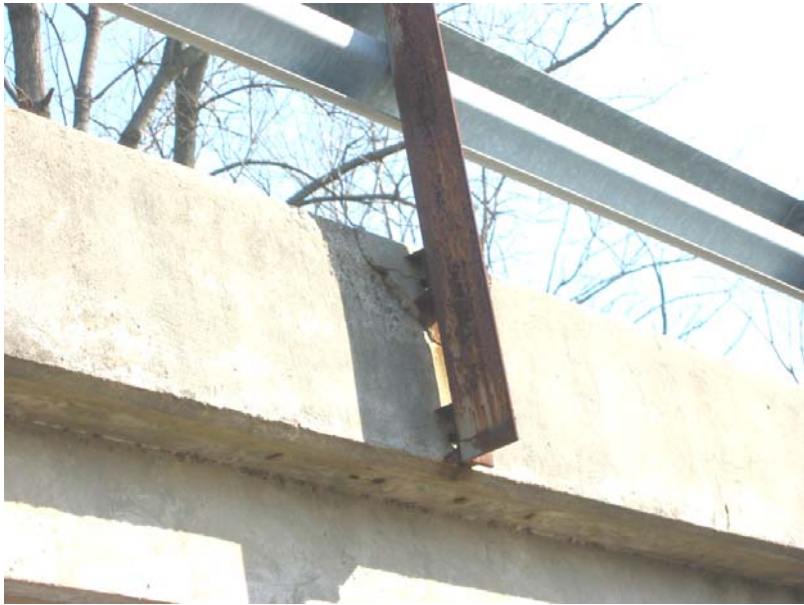
115 Spall at rail post connection
