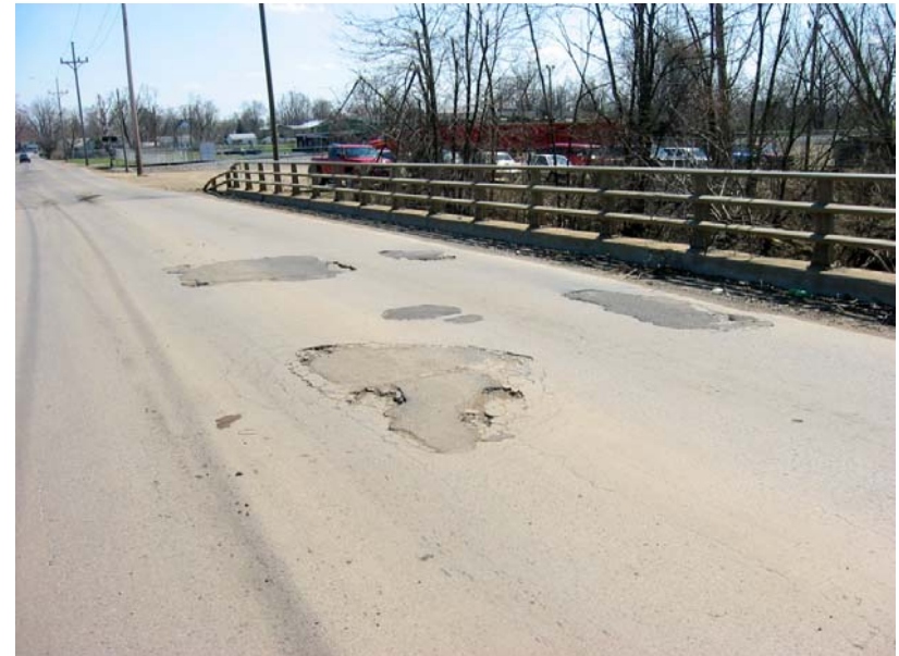
268 Wearing surface heavily spalled
