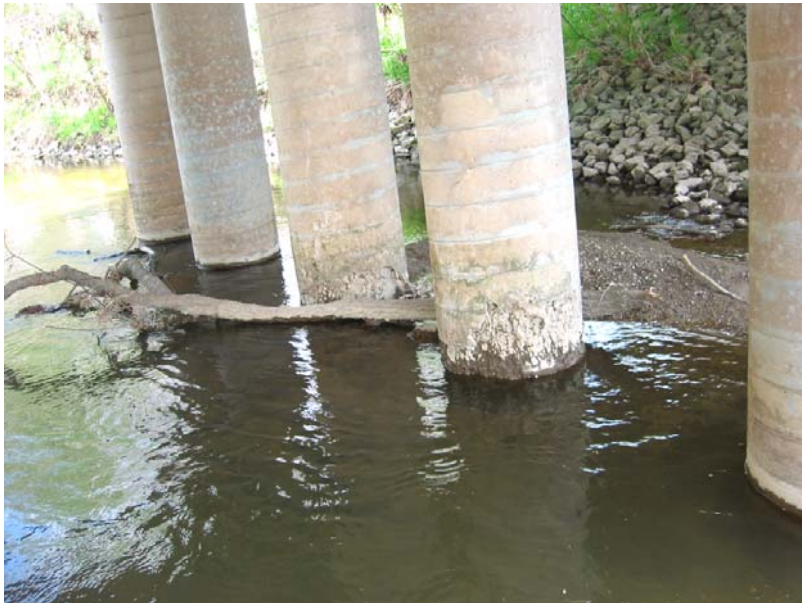
163 Pile encasement damage at the south interior bent
