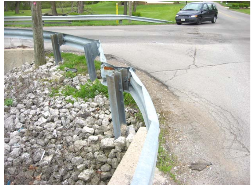
143 Northeast approach rail damaged
