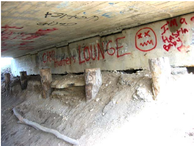
075 North end bent cap undermined
