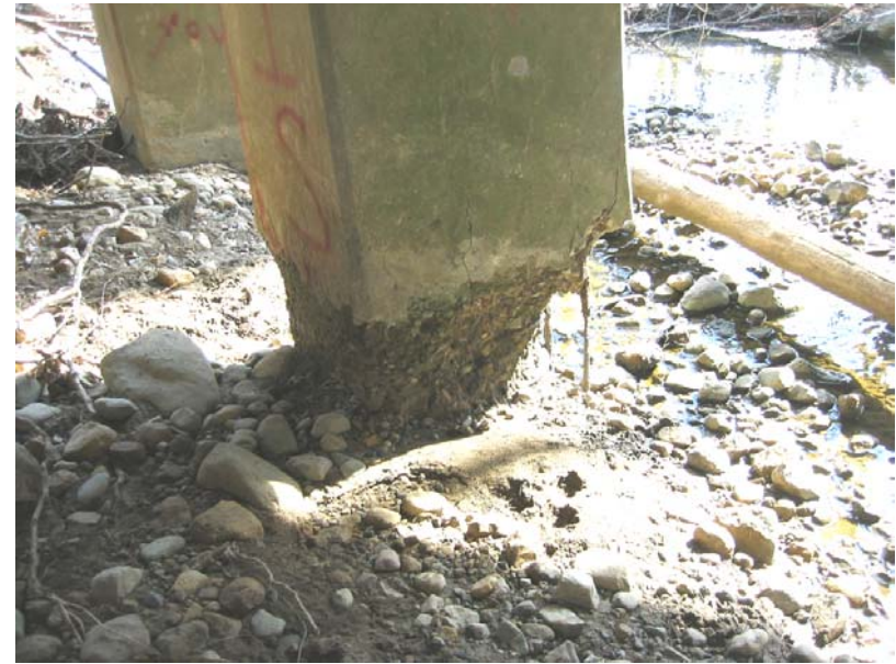
112 Pile encasement deteriorated in east interior bent
