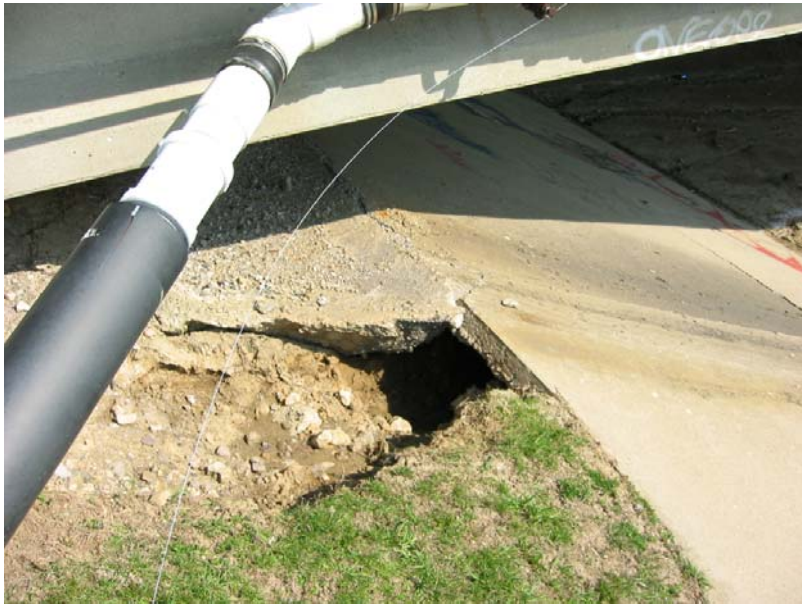
516 Void in the north slope wall
