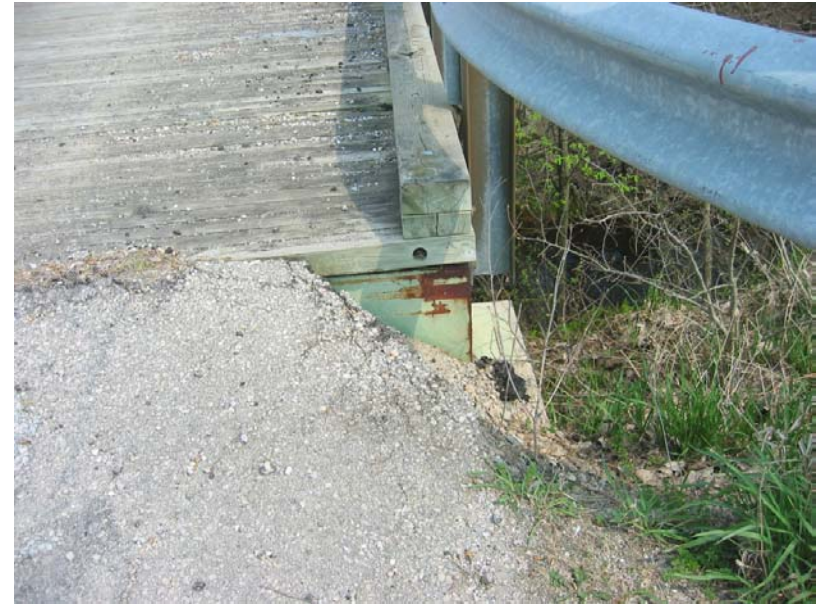
017 Erosion at the southwest corner
