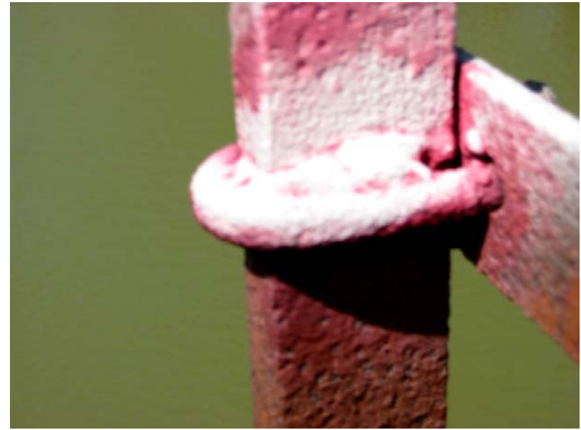
045 Panel point L7 north - U-bolt welded to vertical; possible crack at base of weld
