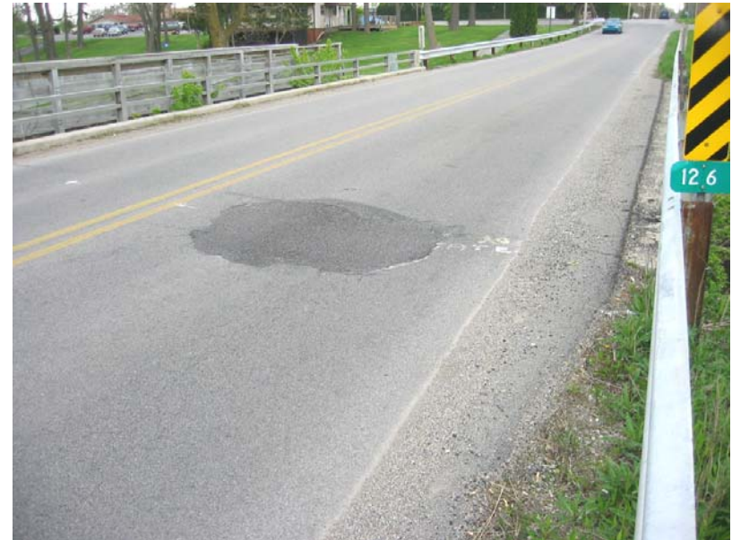
126 Apparent fill loss at south approach
