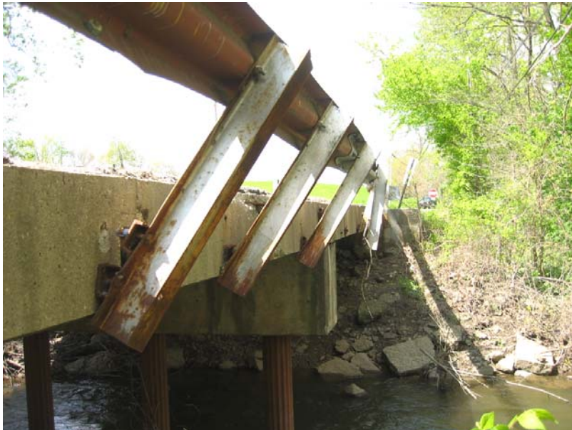
159 North rail and beam damage
