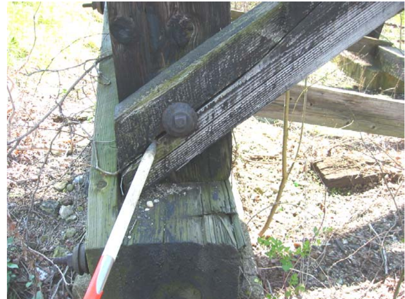
226 Split brace at south bent frame
