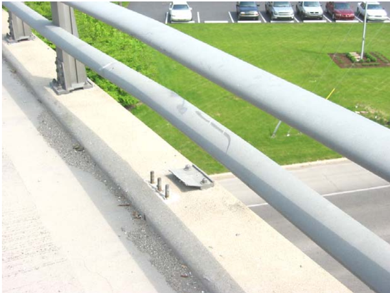
520 Missing bridge rail post - northbound
