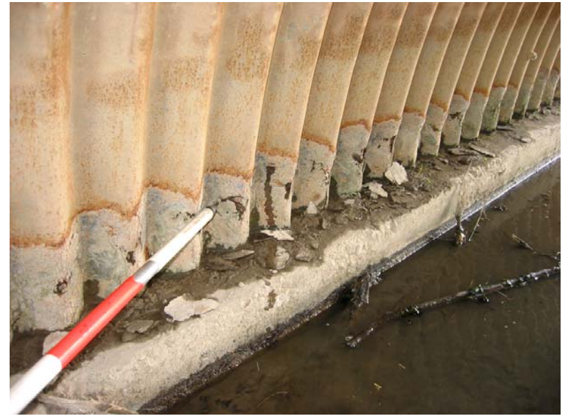
507 Advanced rust at the base of the arches
