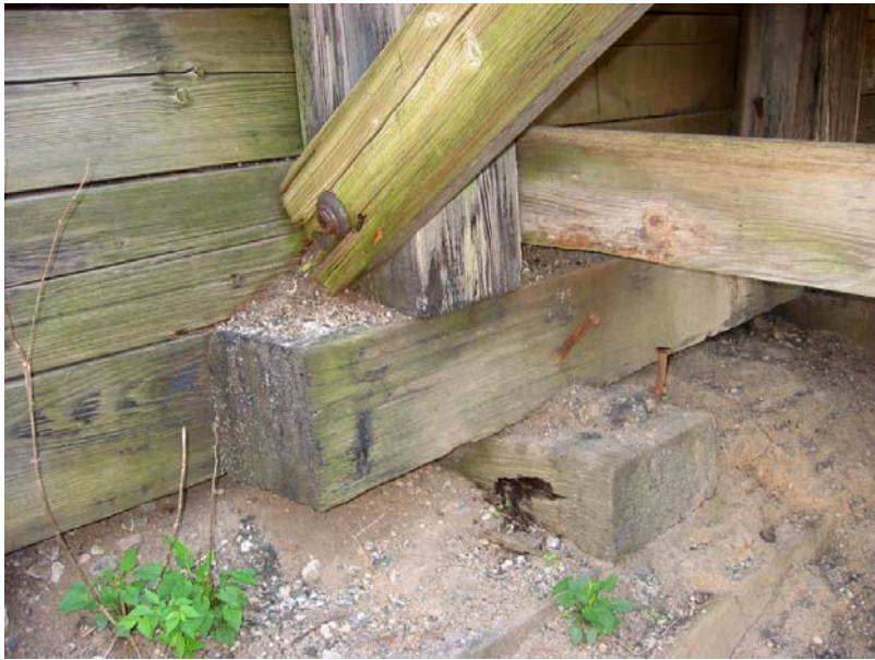
226 Northwest diagonal brace split and rotted and support base rotted
