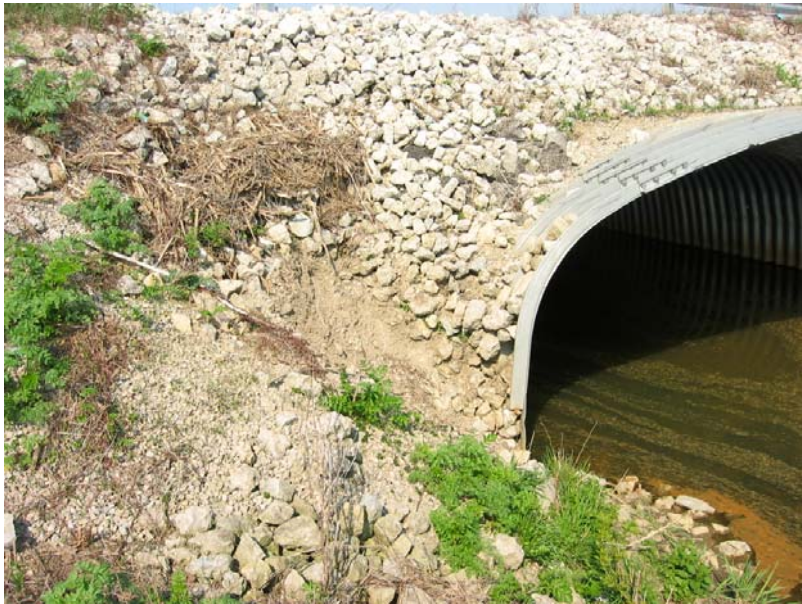
058 Erosion at the southeast corner
