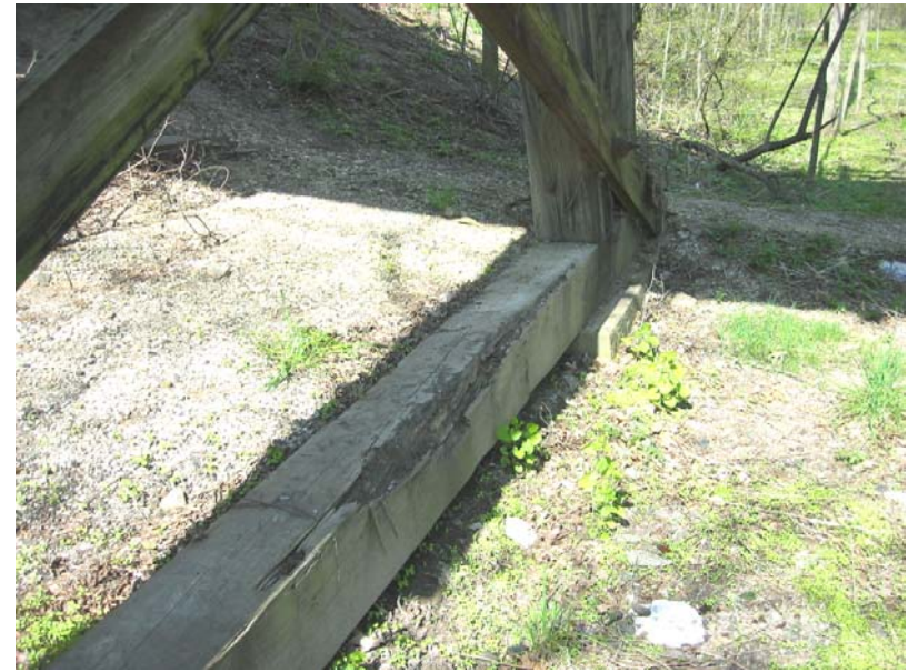
226 Some rot in bottom cross member of south interior bent
