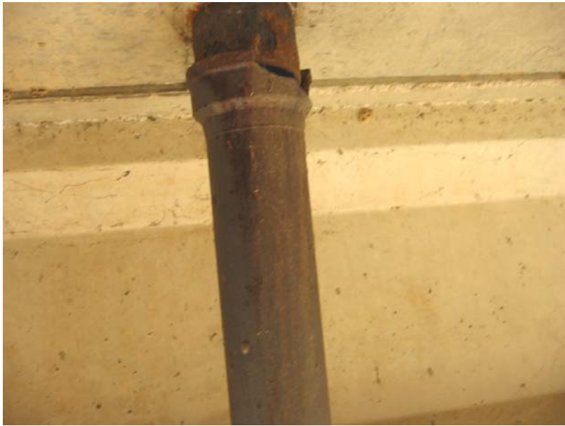
123 Northeast pipe extension broken
