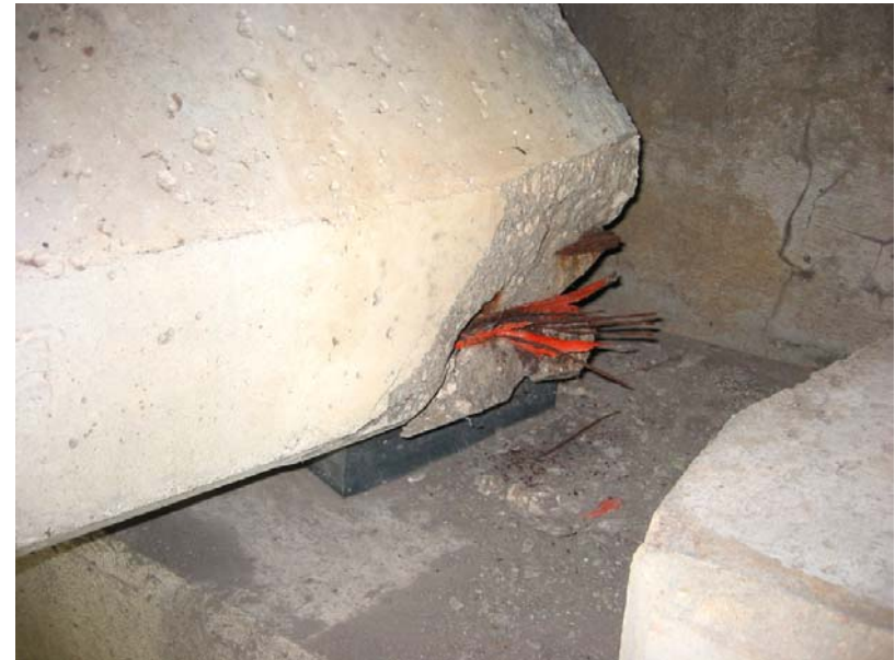
193 Spalls at beam ends
