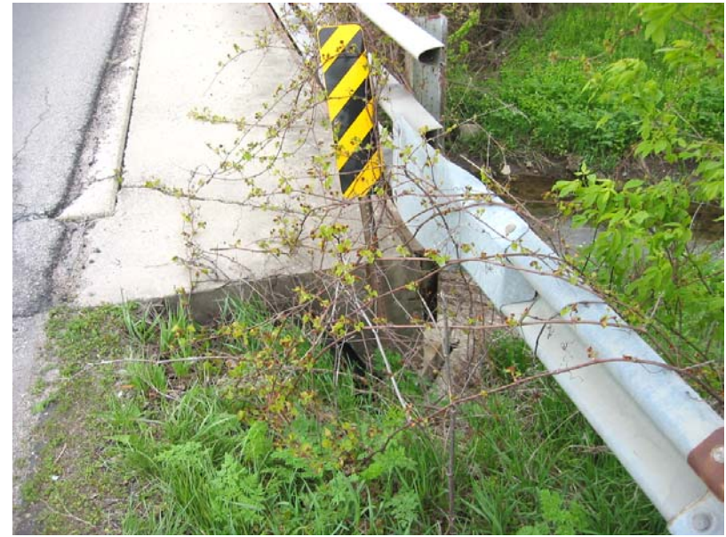
125 Erosion - end of deck exposed
