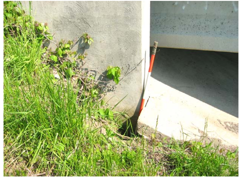
193 Typical erosion at the corners and voids under the slopewall
