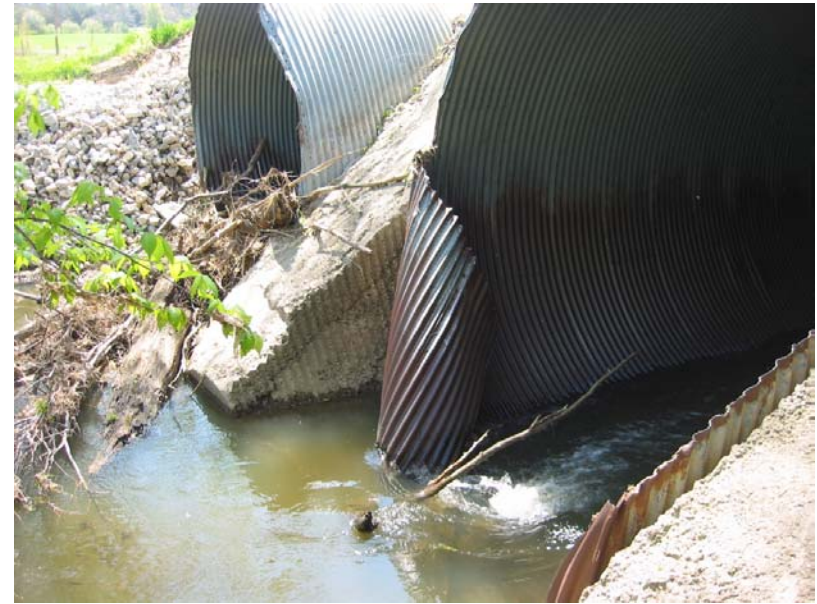
016 West pipe - corrugated metal folding inward
