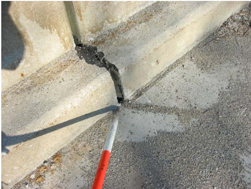
123 Open joint at the curb
