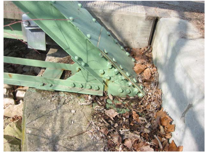
108 Typical debris at endposts
