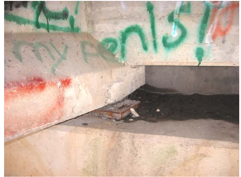
141 Damaged beam and deteriorated bearing
