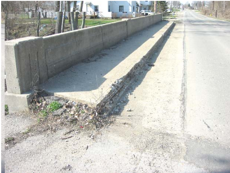
502 Deteriorated curb
