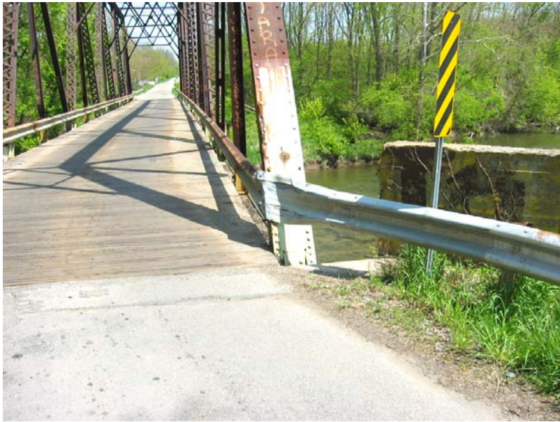
161 Rail damage at the southwest corner
