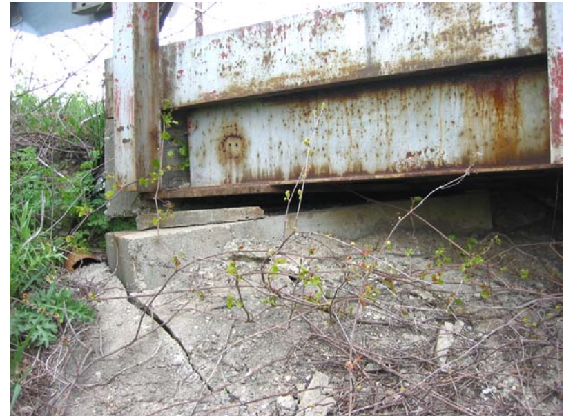
125 Substructure settled at northwest corner
