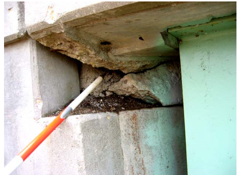
051 Haunches broken at the endbents
