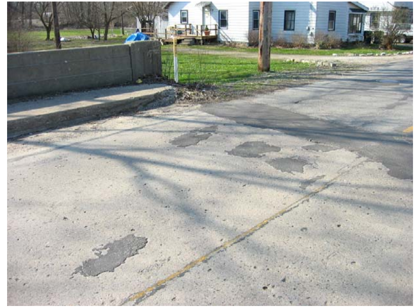
502 Wearing surface spalls and patches
