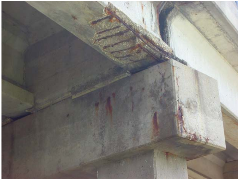
520 Beam damage at the west end of the north interior bent
