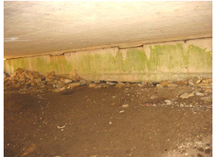
133 West end bent undermined
