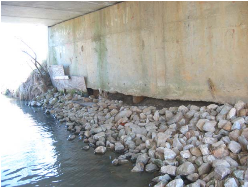
053 South abutment undermined
