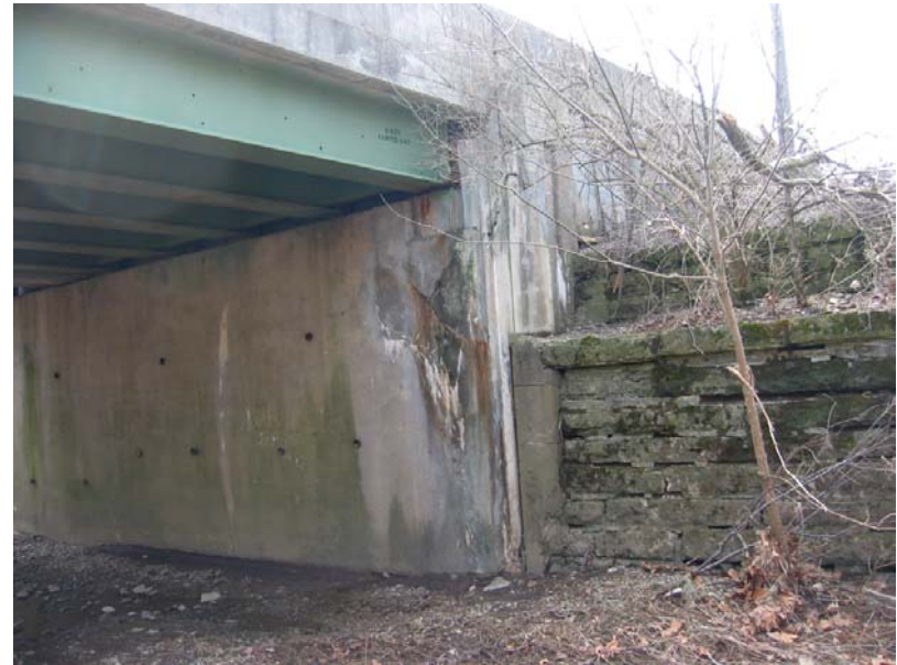
027 Southwest abutment corner cracked and efflorescing
