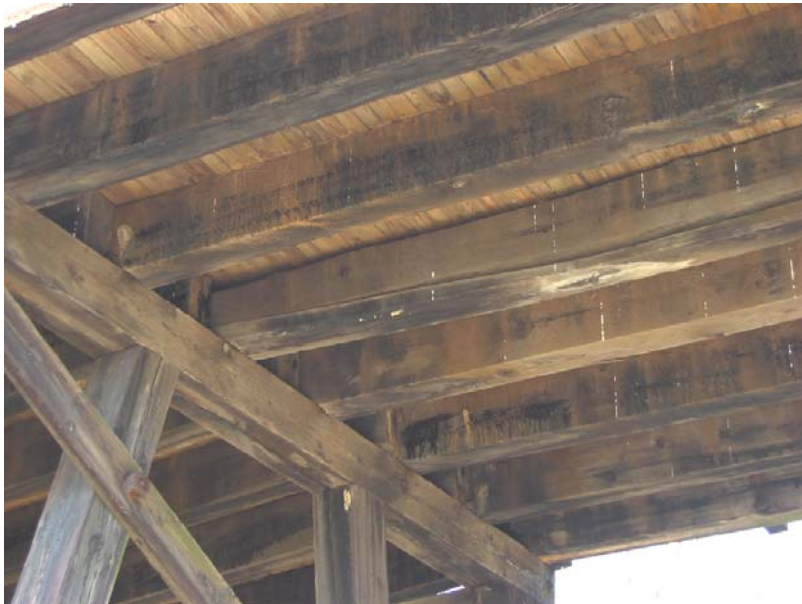
226 Split beam in main span with gap between beam and floor timbers
