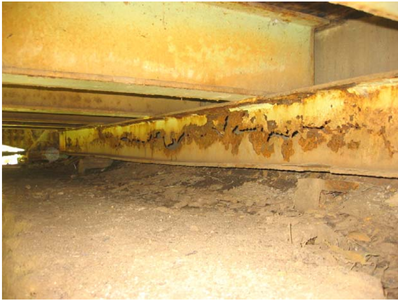
161 East end floor beam - web failed
