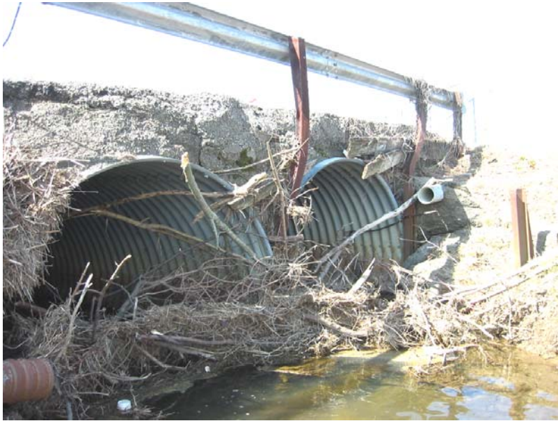
190 Debris at inlet, failing slope, inadequate guardrail.
