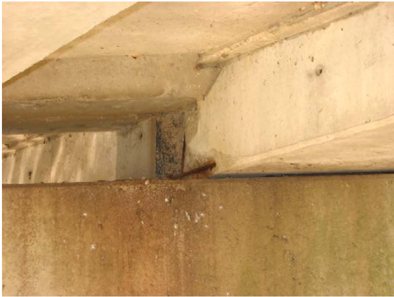
171 Moderate damage at end of beam over the east pier
