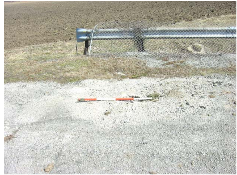
190 Hole in road surface due to fill loss
