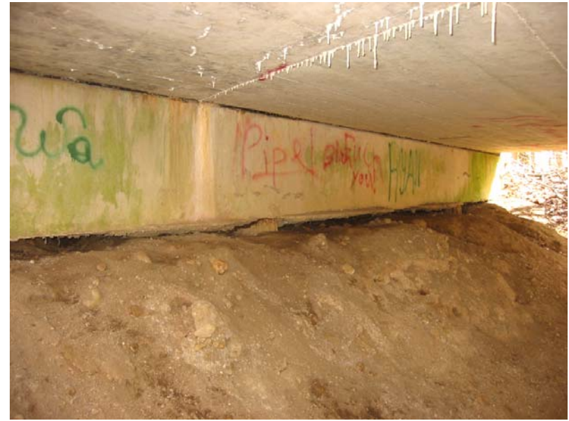
112 East end bent cap undermined
