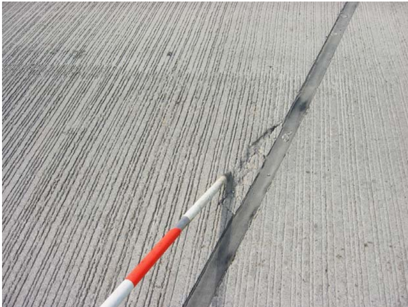
520 Wearing surface damage at a joint - northbound
