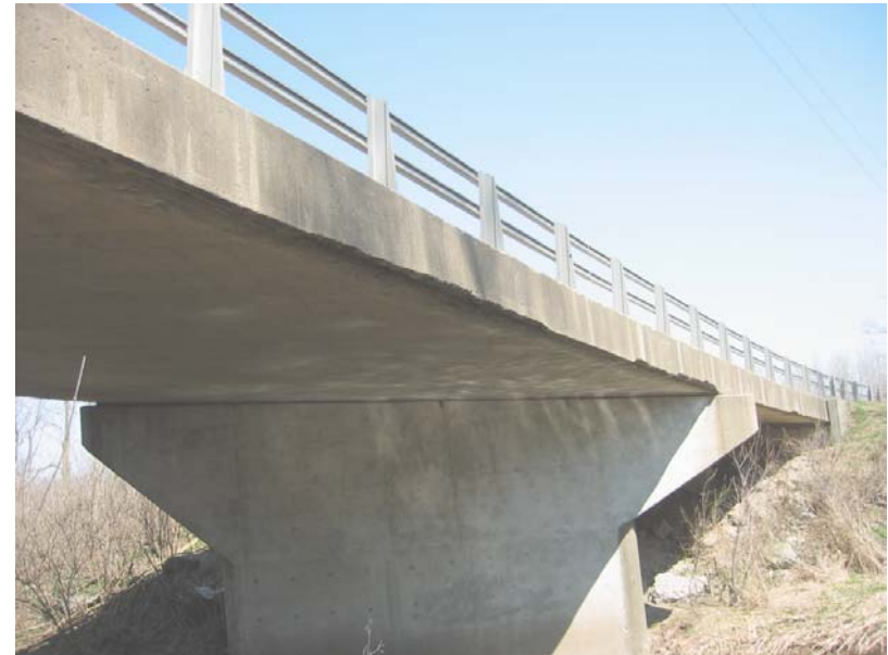
146 Spalls in the east coping - center span
