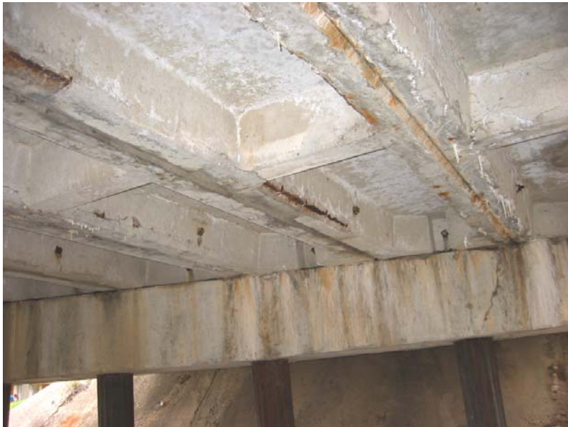
127 Beam spalls at center span
