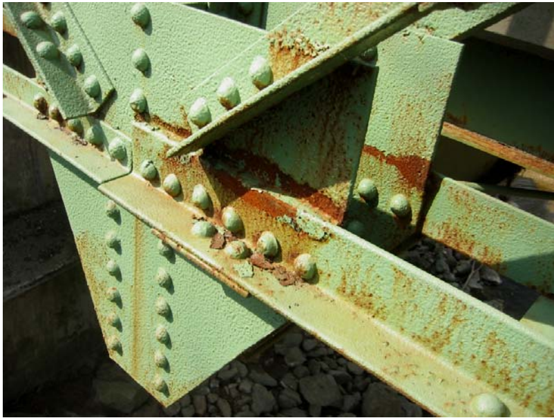
108 Southeast floor beam connection - outside of outer plate
