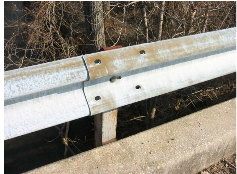
115 Bridge rail splice not bolted
