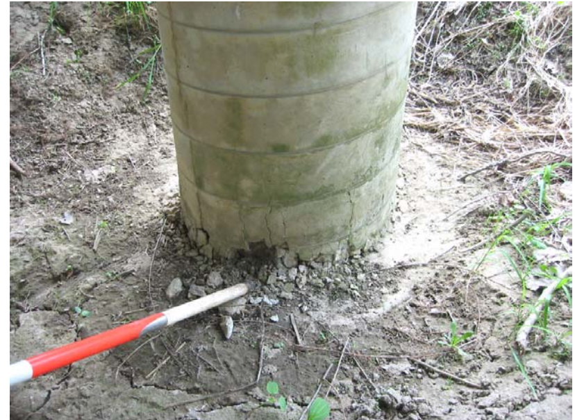
163 Pile encasement damage at the north interior bent
