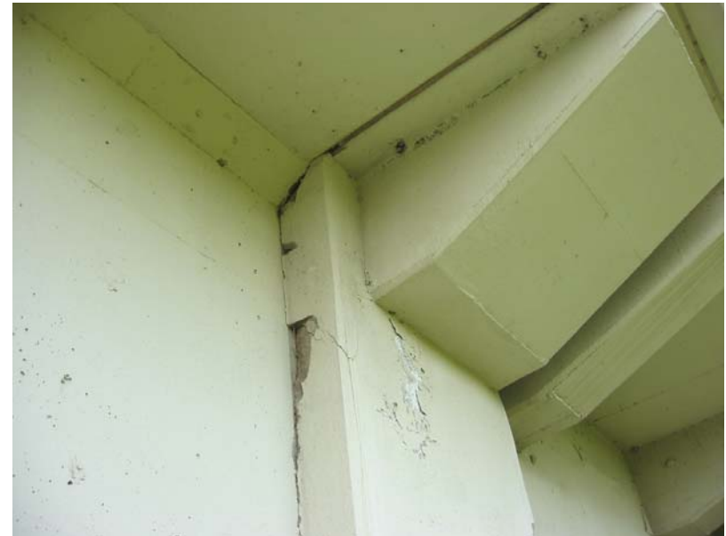
514 Spalls and cracks at column
