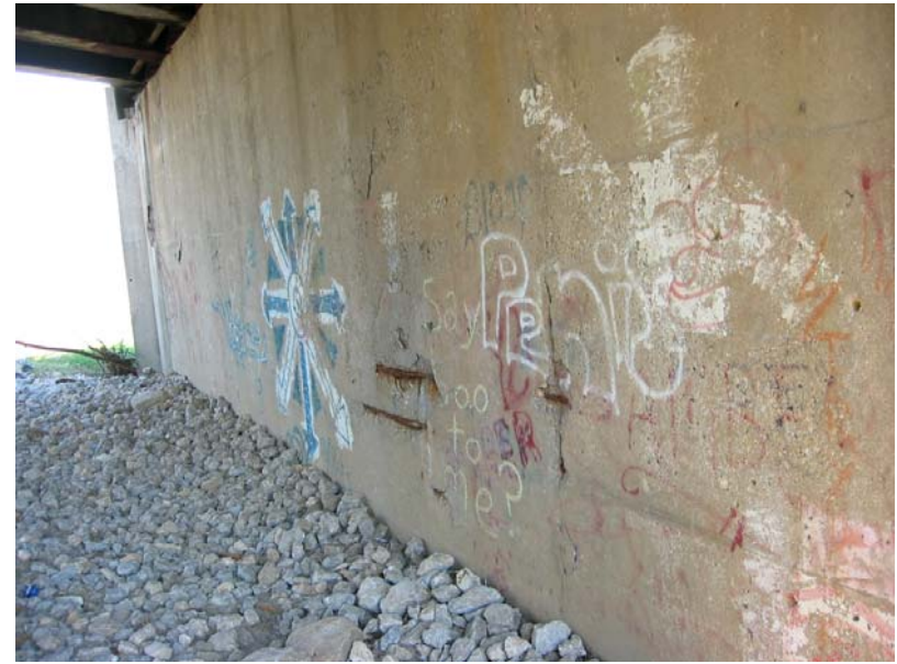
513 Spalls, delamination at the face of the west pier
