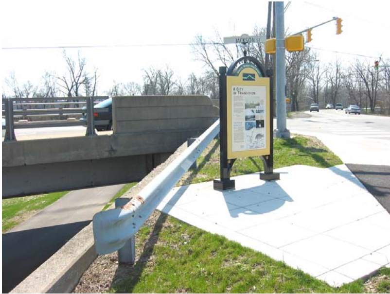
513 Low rail next to pedestrian trailhead and adjacent to retaining wall
