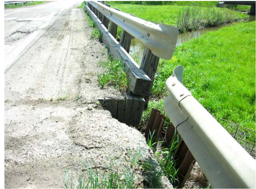
103 Southwest rail leaning - outer slab timbers rotated
