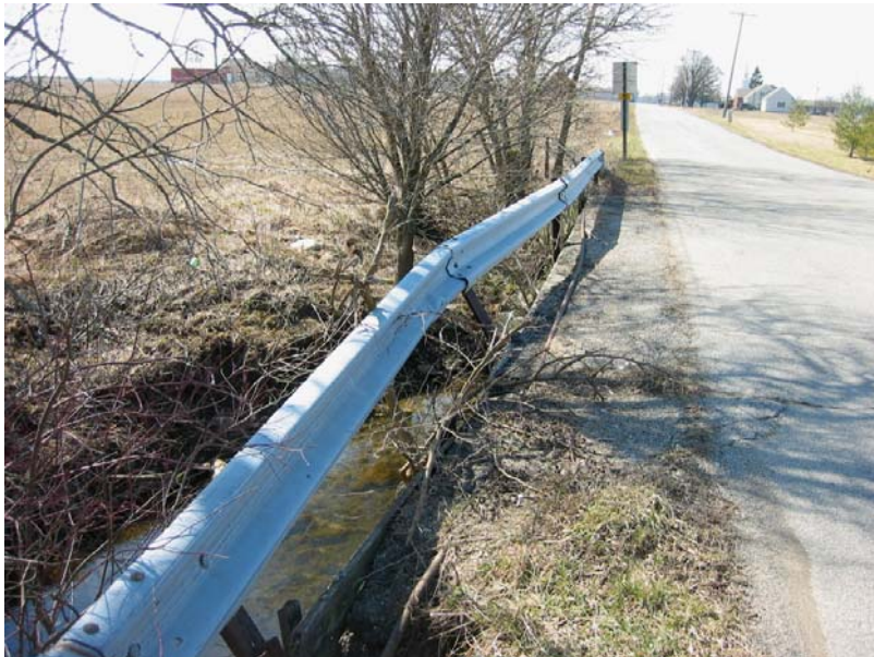
191 Damaged south rail
