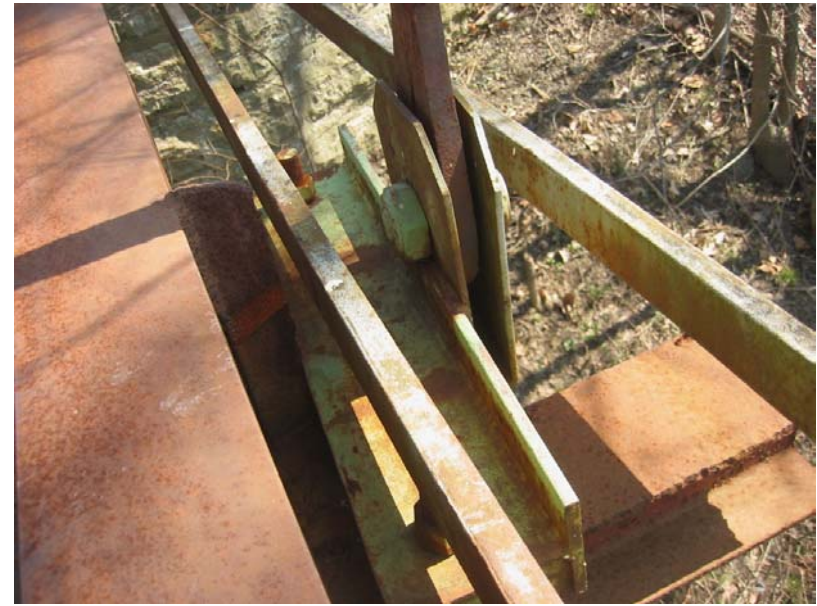
045 L11 south - retrofitted hanger welded to old hanger
