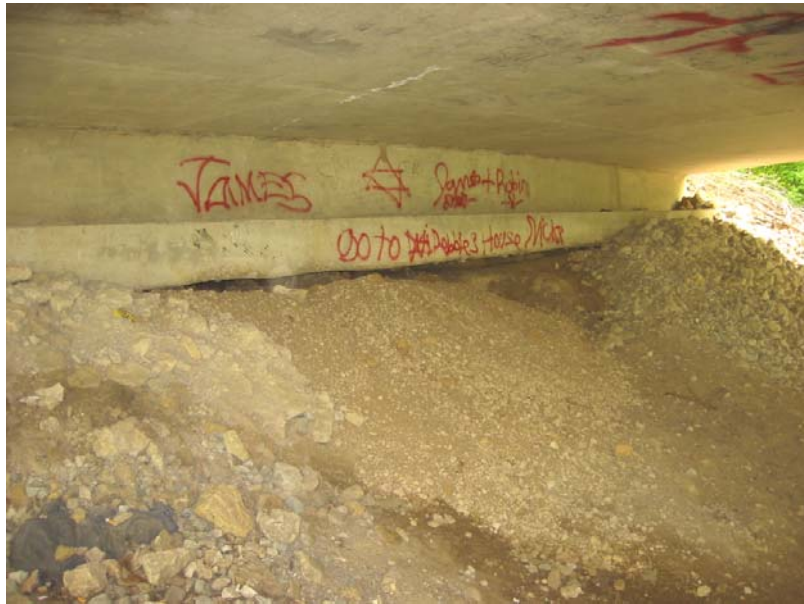
511 Northeast endbent cap undermined
