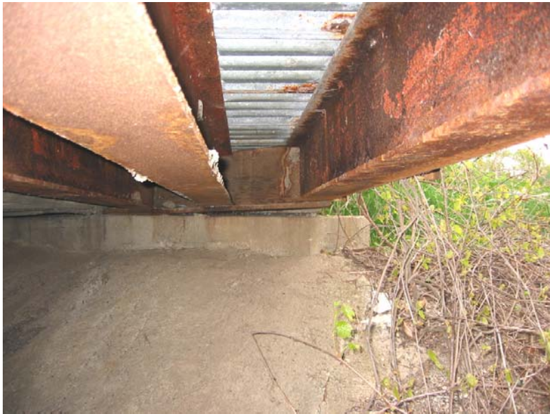
125 Substructure settled at the northeast corner
