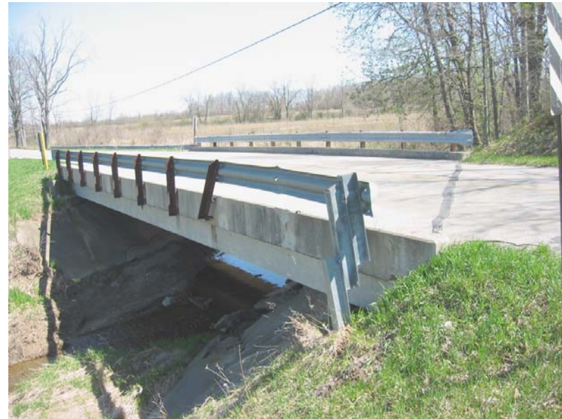
056 North bridge rail damaged
