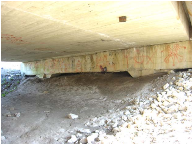
502 Erosion at the south endbent
