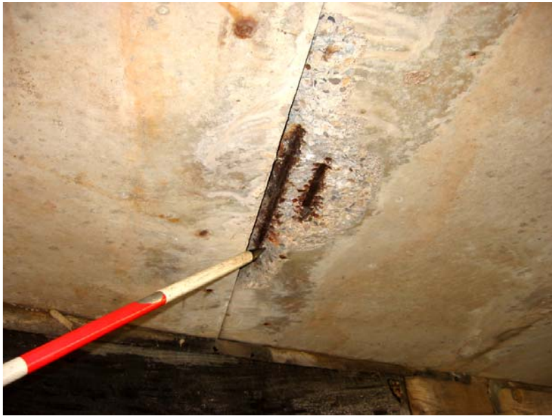
015 Spalled beam and broken strands
