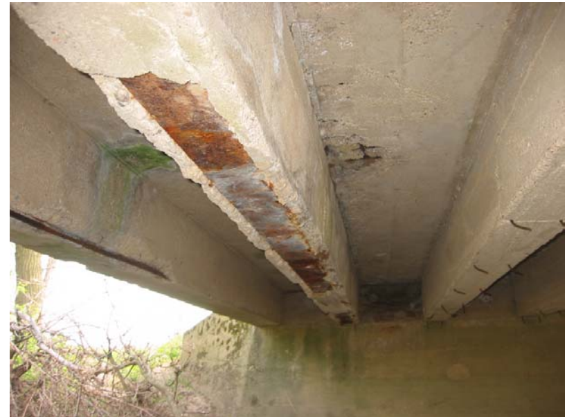
087 Concrete spalled and heavy delamination at encased beams
