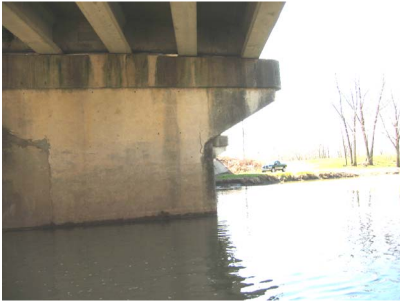
141 Spall at the north pier
