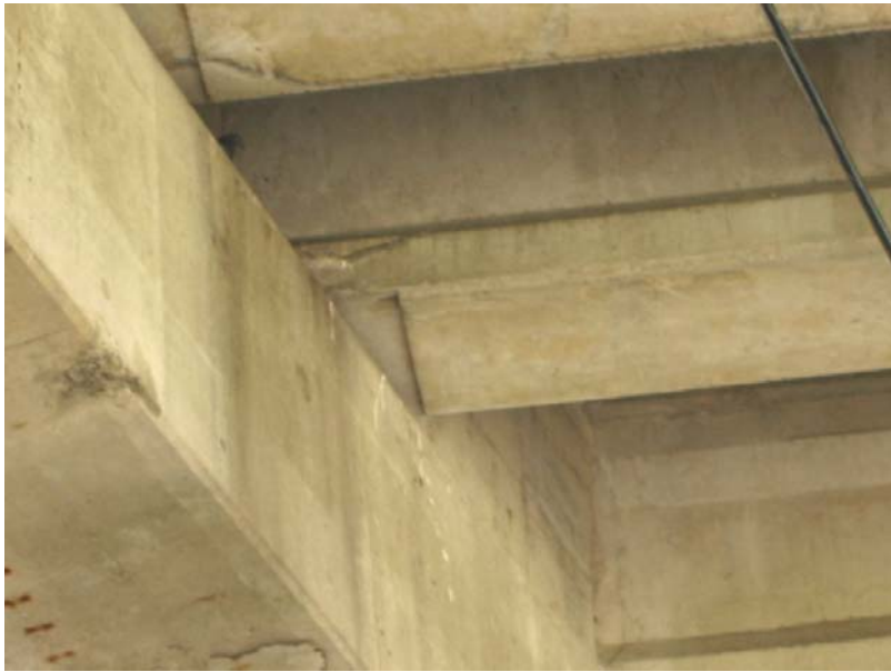
520 Crack at the bottom flange in beam at the 2nd interior bent from the south
