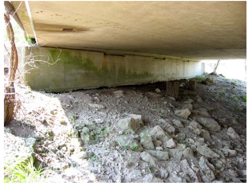
059 South end bent undermined
