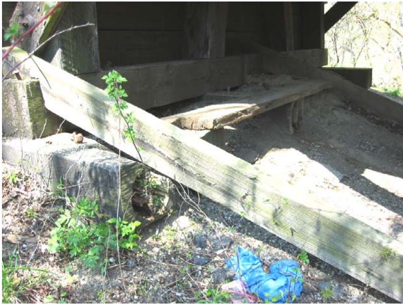
226 Two support timbers rotted at the south end
