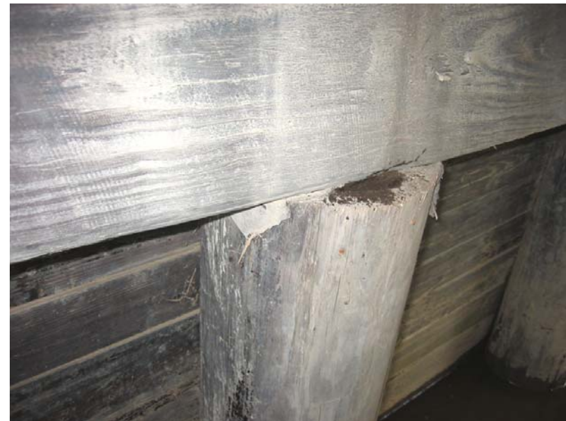
050 Center pile in north endbent
