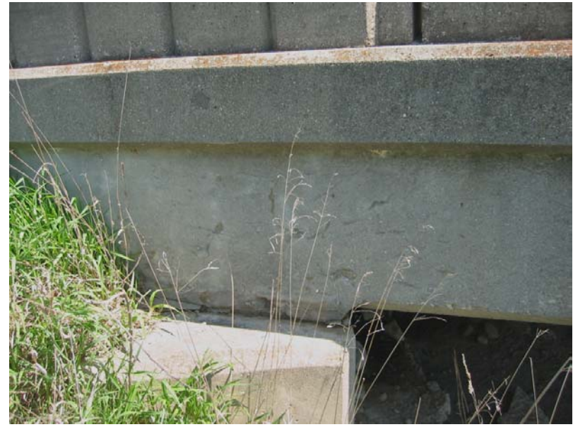
069 Cracks in coping at the northwest corner
