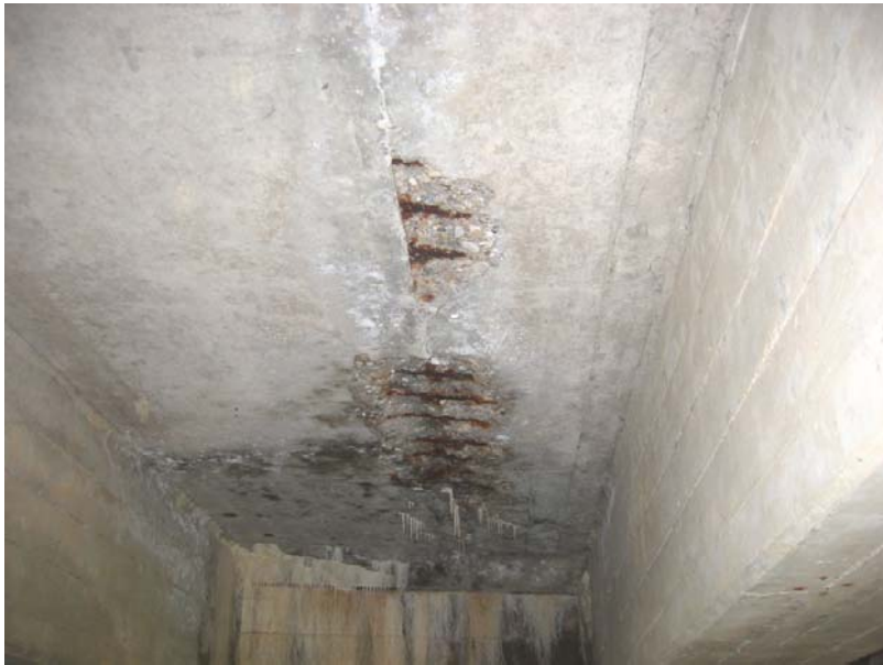
501 Spalled deck below
