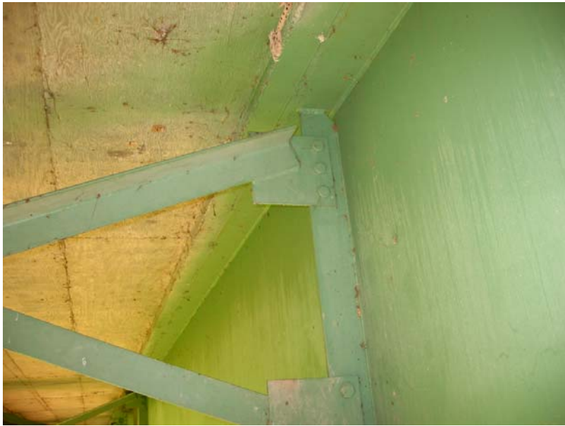
095 Typical diaphragm at the top
