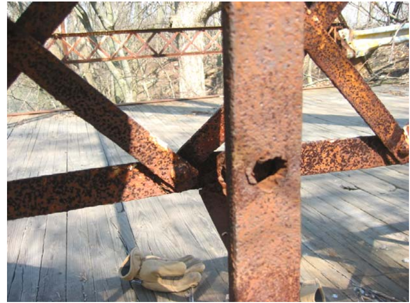
045 Panel point L11 south - hole in vertical
