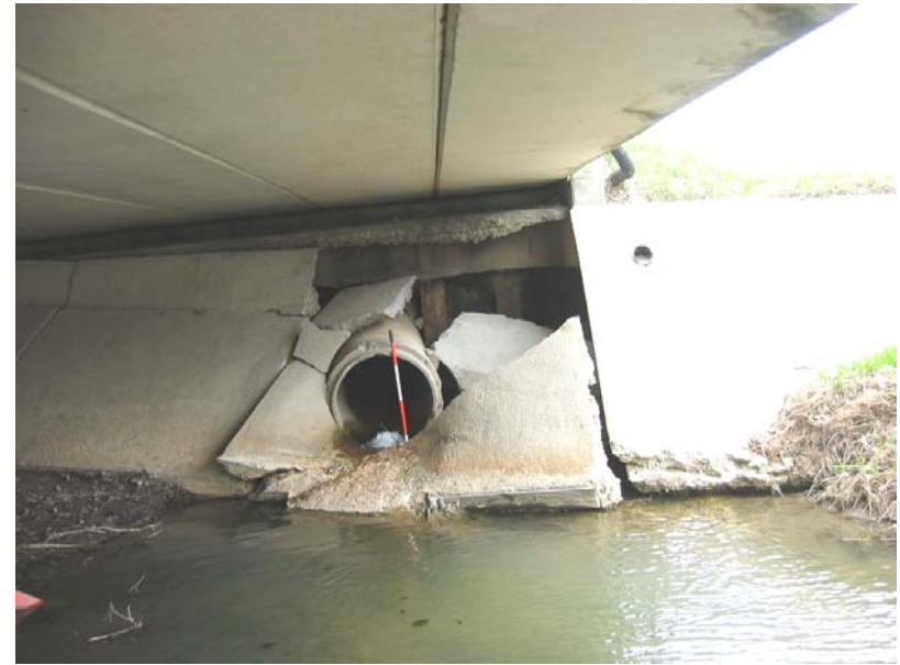
509 Failed sloped wall, lost fill – 2 of 3 photos
