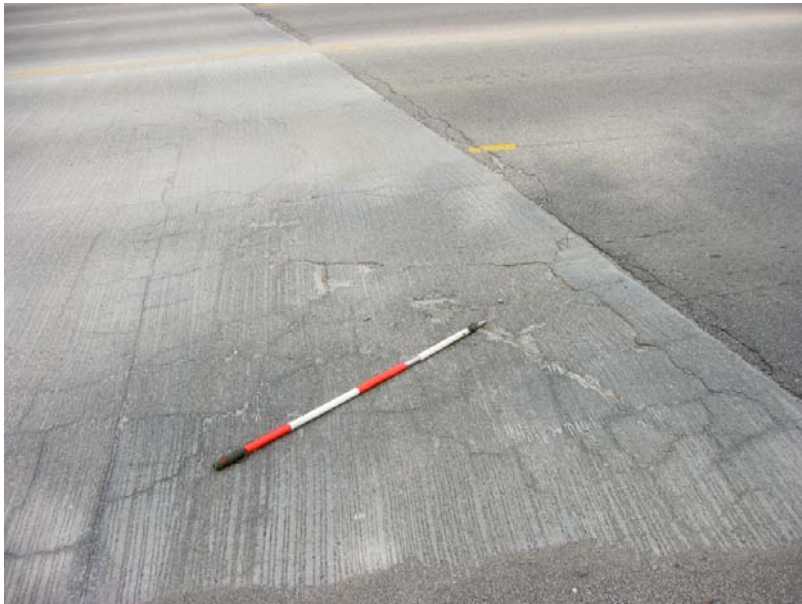
501 Cracks in the wearing surface at the north end
