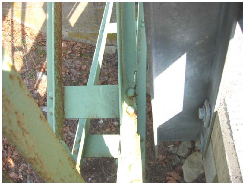
108 Northwest diagonal cut to accomodate bridge rail post
