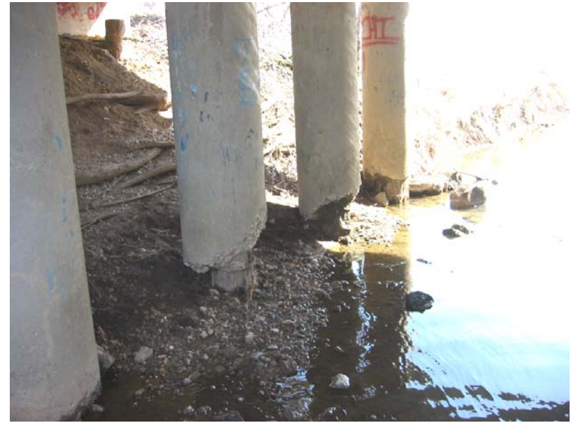
075 Heavy spalling at pile encasements
