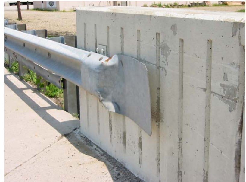
508 Transition damage at the northeast corner
