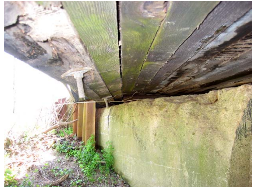
103 Northeast outer timbers unsupported.
