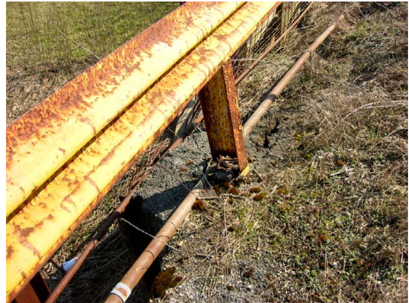
194 Rail posts rusted through
