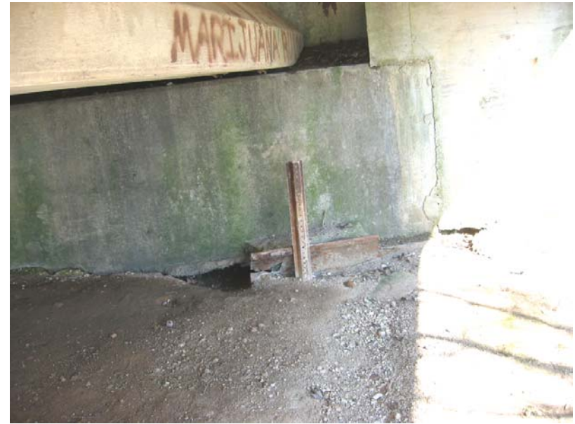
141 North end bent undercut near the east end
