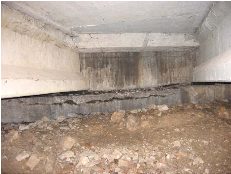
519 Delamination at the south end bent cap
