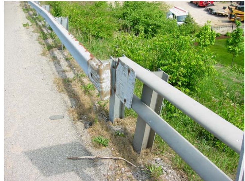
520 Typical transition from aluminum to steel rail
