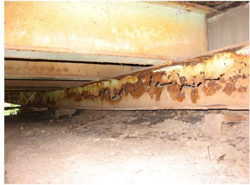
161 East end floor beam - web failed
