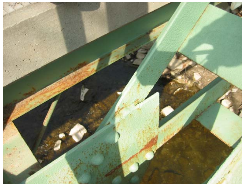
108 Southeast floor beam connection - outside of inner plate.
