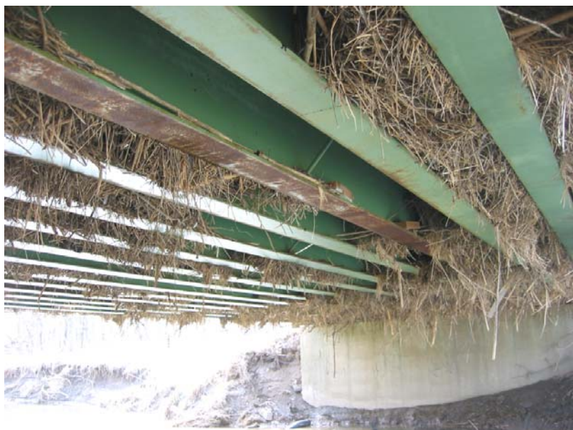
037 Debris in beams
