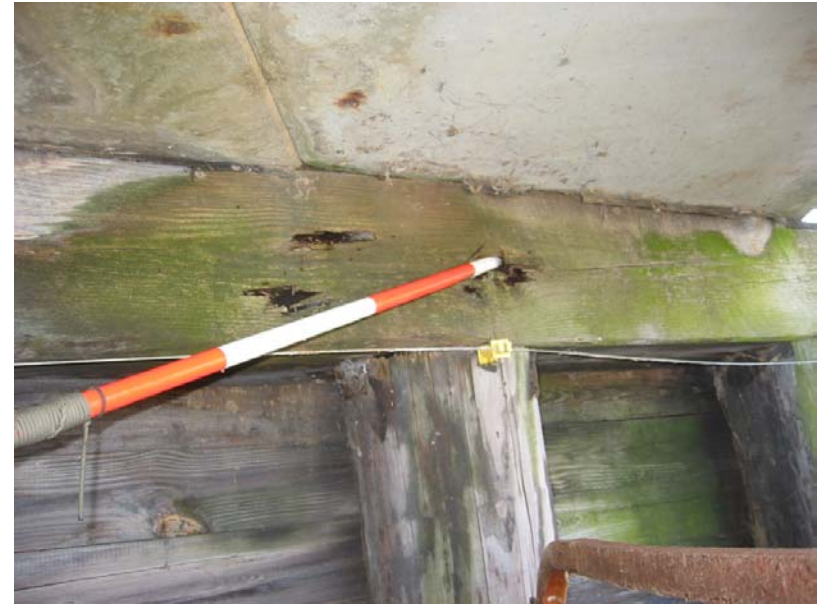
015 Considerable rot in the south end bent cap
