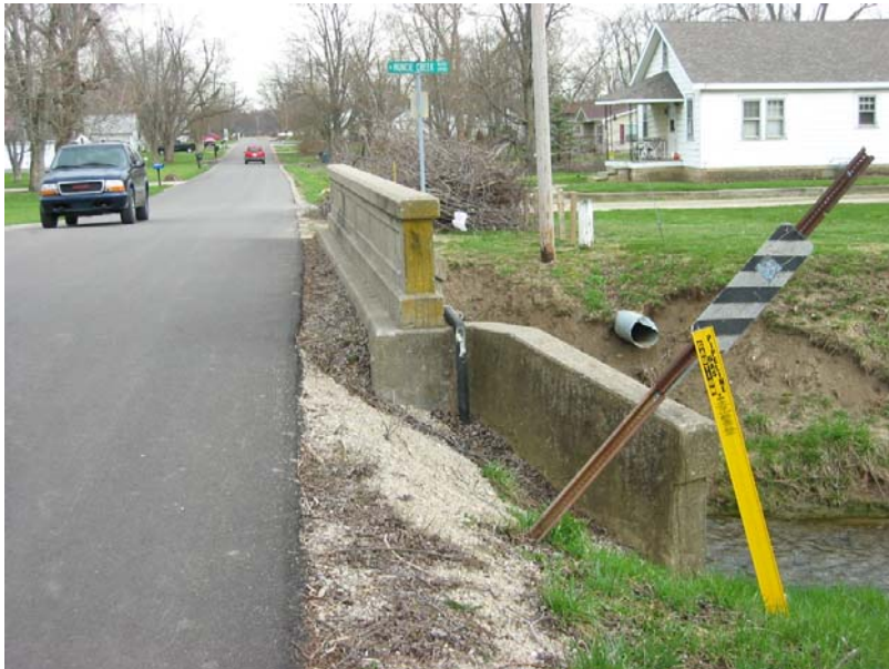
245 End of curb and rail exposed to traffic
