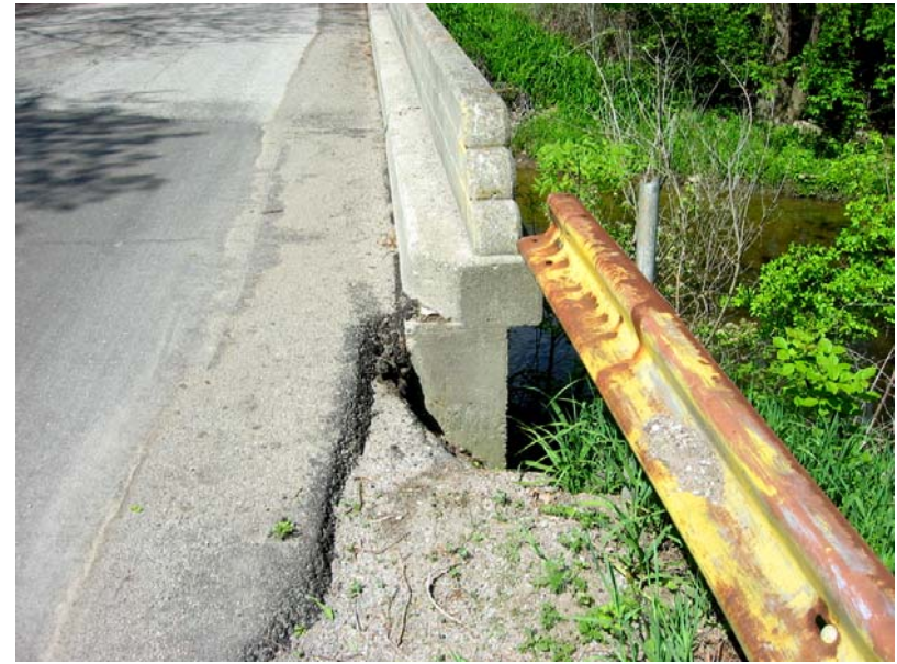
092 Eroded northeast shoulder.
