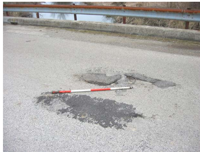
138 Deck spalled
