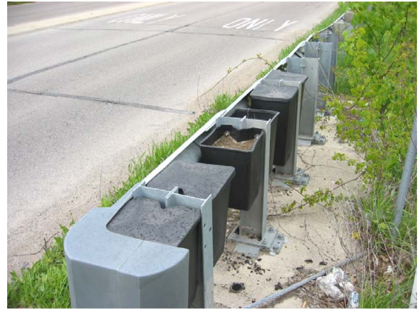
124 Lids missing at southeast attenuator
