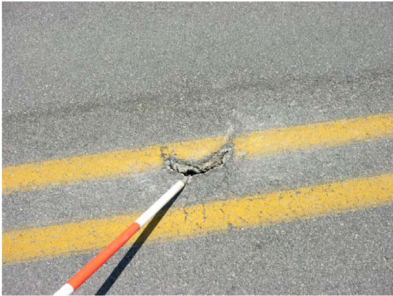
020 Spalled deck concrete coming through new asphalt wearing surface
