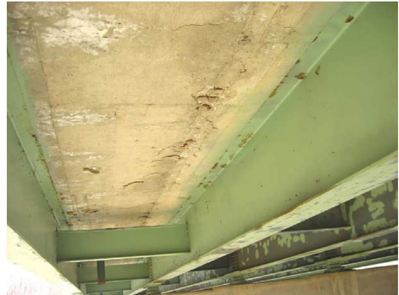
051 Spalls in deck at the east span near the south side
