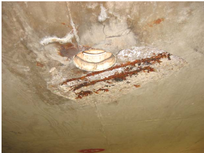
511 Spalls around PVC drain outlet
