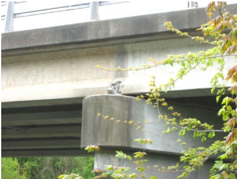
149 Deteriorated grout at beam ends over piers
