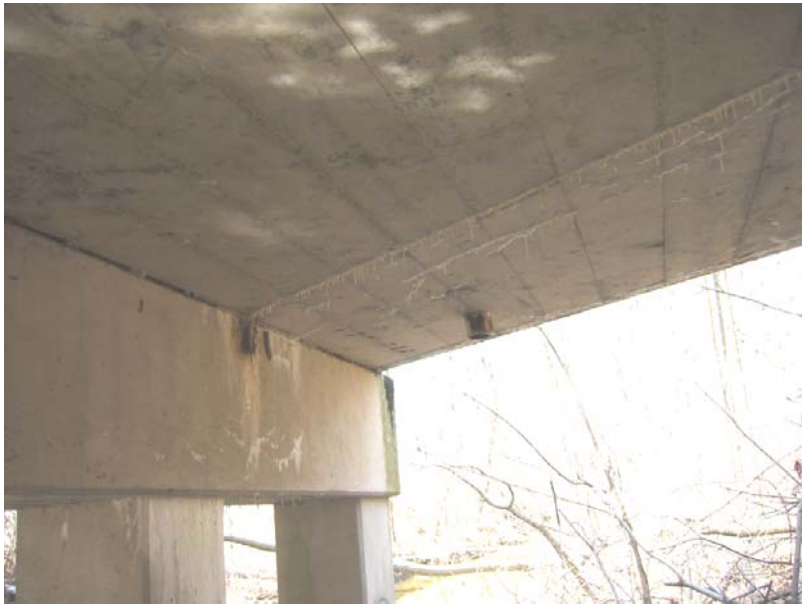
112 Cracks and efflorescence in slab and cap
