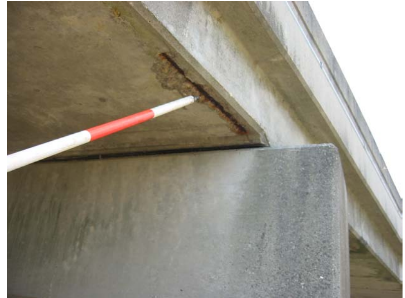
001 Spalls below the slab at the east coping south of the south pier
