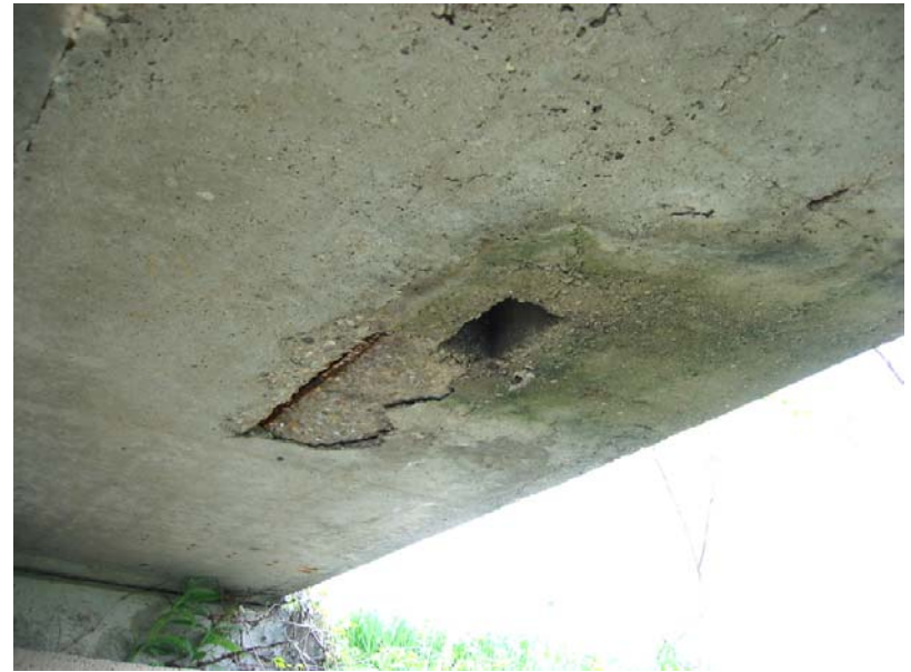
100 Spalled slab below
