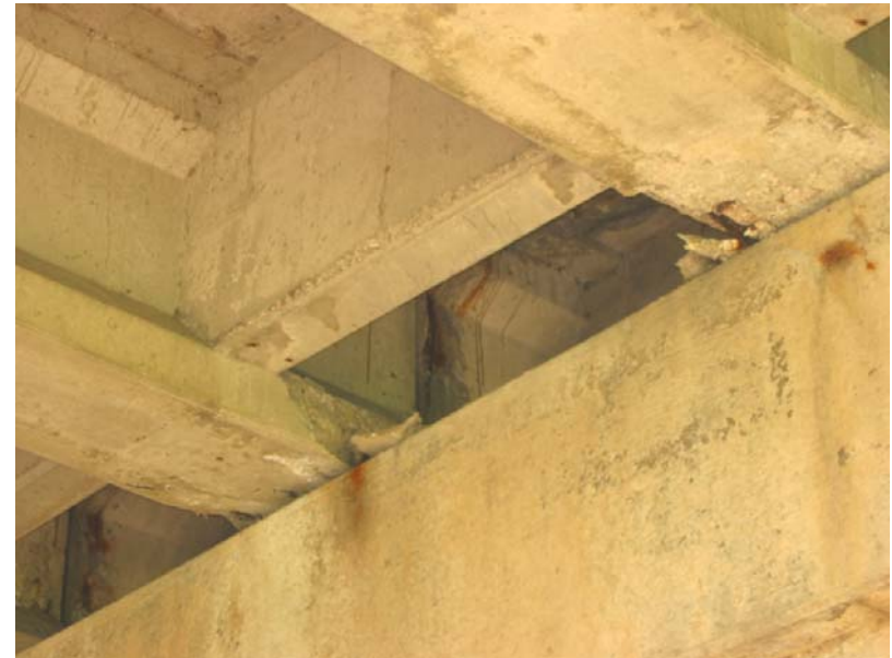
516 Damaged beams at the north pier
