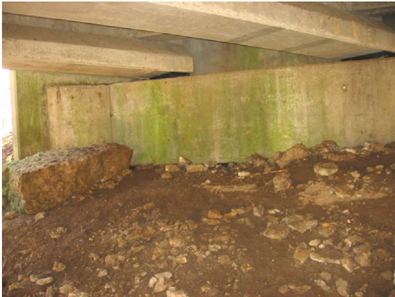
084 Undermining at the south end bent
