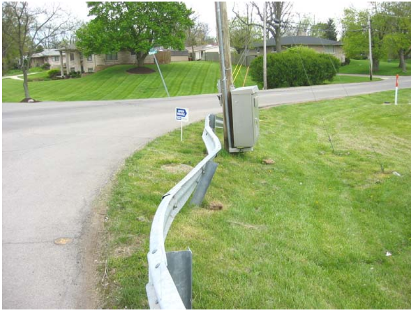
143 Southeast approach rail damaged
