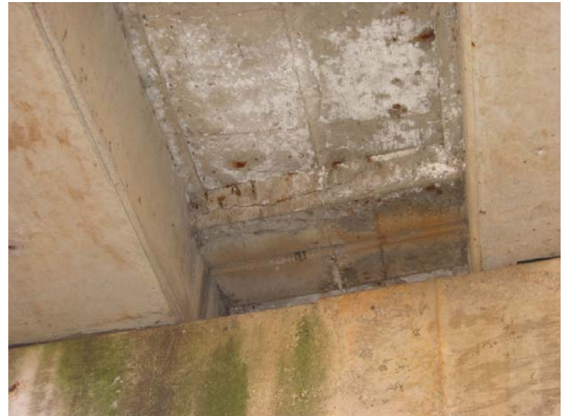
179 Cracks in deck near the joints
