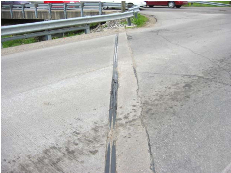
143 East joint deteriorated
