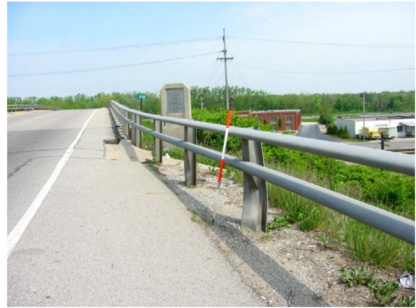
520 High aluminum rail and post damaged
