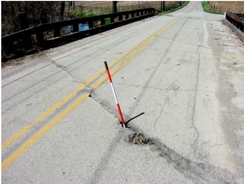
061 Apparent fill loss at the east end
