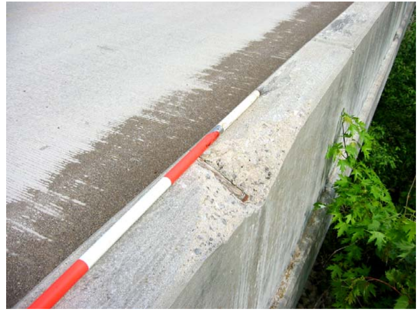
095 Spalled rail
