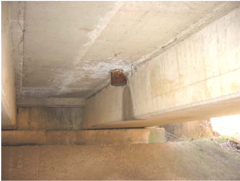
179 Deck drains onto the beams
