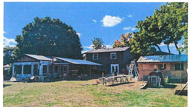
back yard, rear house view from INSIDE privacy fence
