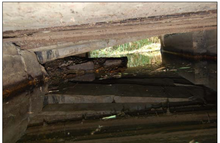
Collapsed at Mid Point
