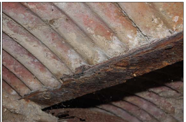
Beam Corrosion
