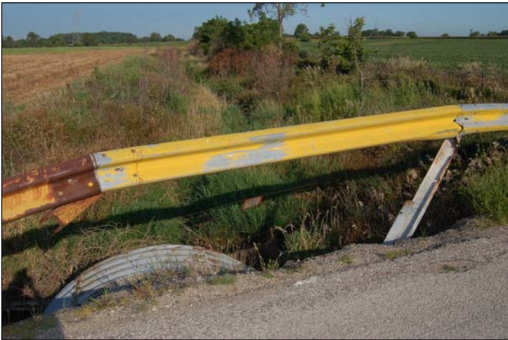
Damaged Railing
