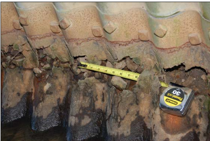
Corrosion - up close
