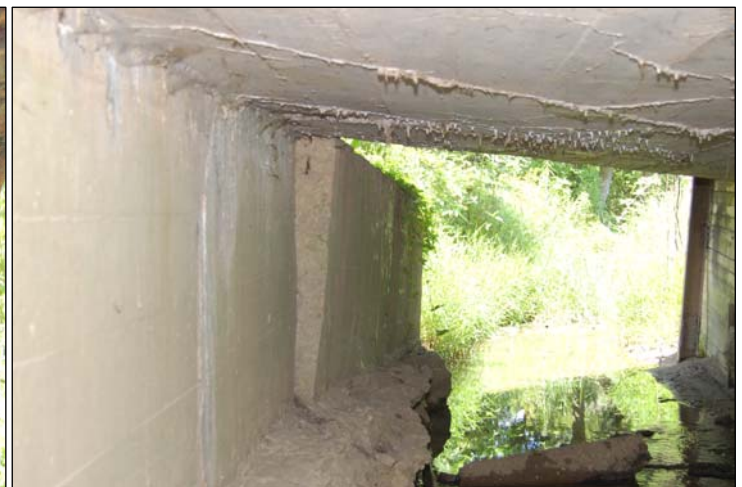
South West Abutment Movement
