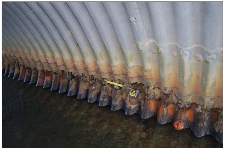
Corrosion – North Side
